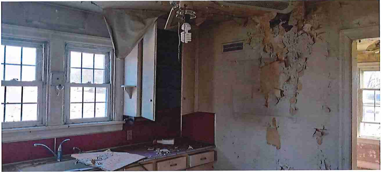
Kitchen Wall A
