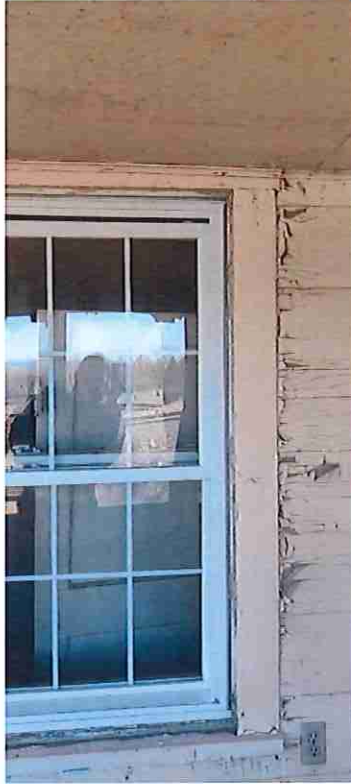
Back Porch Wood Window Components, Wall Side and Ceiling
