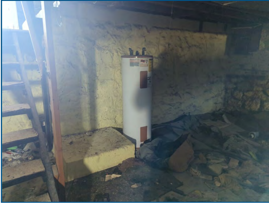
Photograph # 5 View of the basement.
