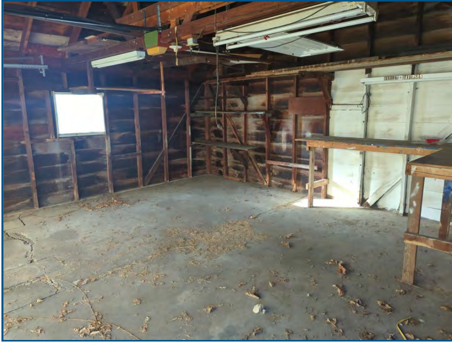
Photograph # 9 View of the interior of the garage.
