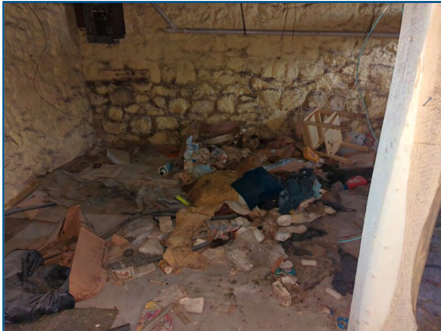
Photograph # 4 View of the basement.
