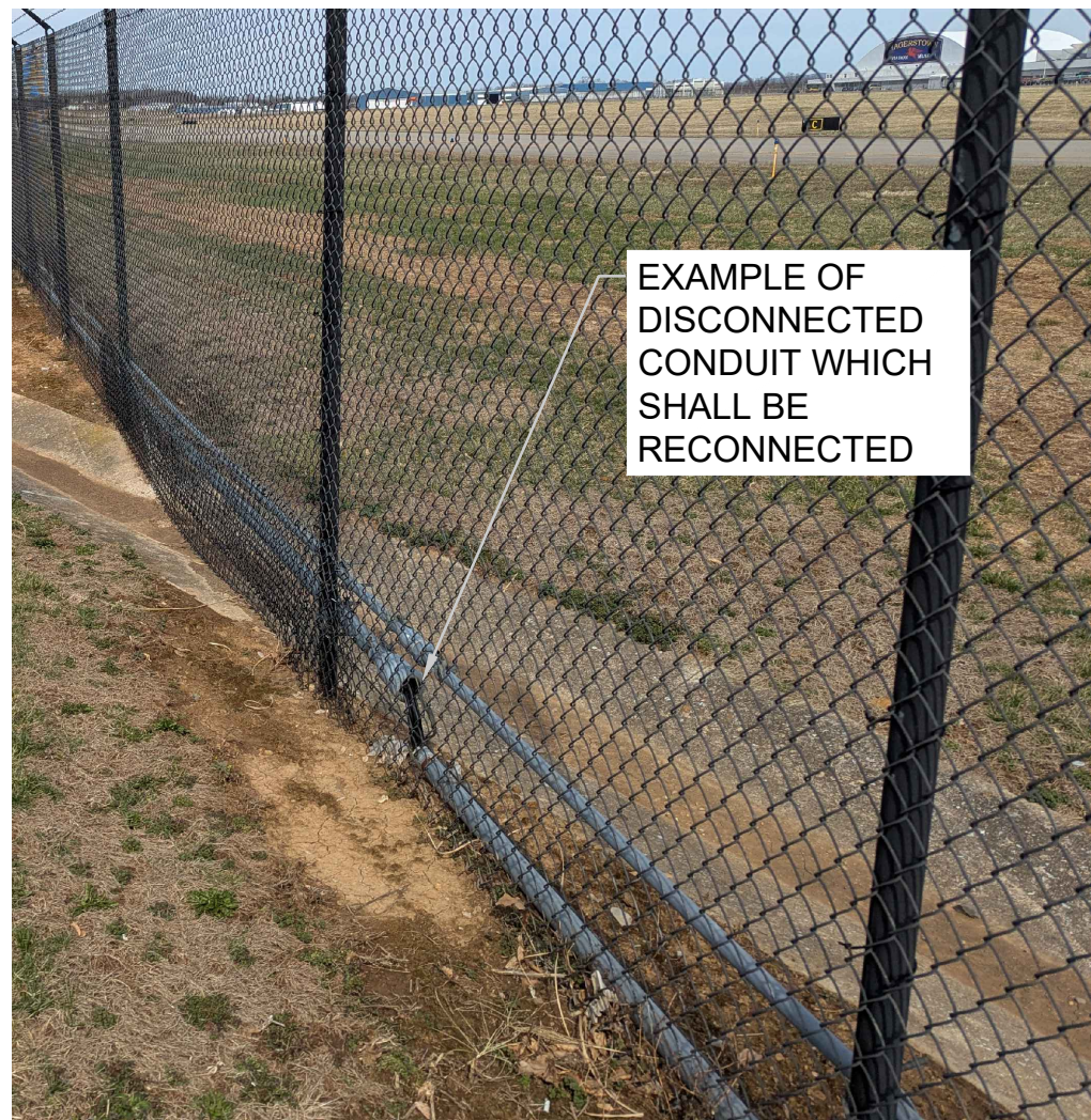
1 DISCONNECTED CONDUIT CU102 SCALE: NTS
