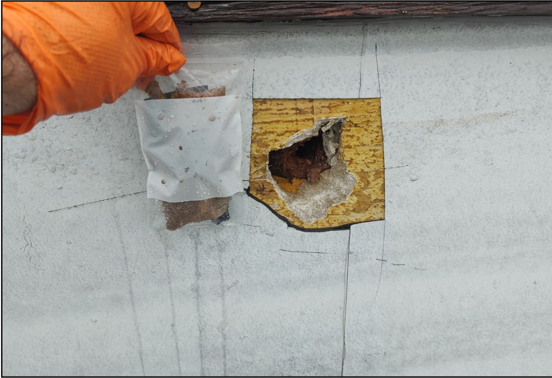
13. View of HA #20—Membrane, Rigid Fiber Board, and Cellulose-like Board located at the ~4-foot Wall at Roof Elevation Change between Western Low Main Roof and Upper Main Roof. Laboratory analysis reports a layer of this material contains 20% Chrysotile. Other layers examined by the laboratory were reported to contain Trace <1% Chrysotile, but such concentrations may be from contamination from the “Transite” layer.
