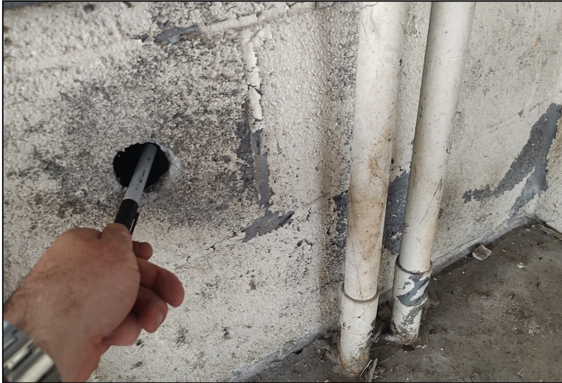
5. View of a test cut to inspect for the presence of Vermiculite within the CMU Block. Vermiculite was not identified in test cuts made by F&R.
