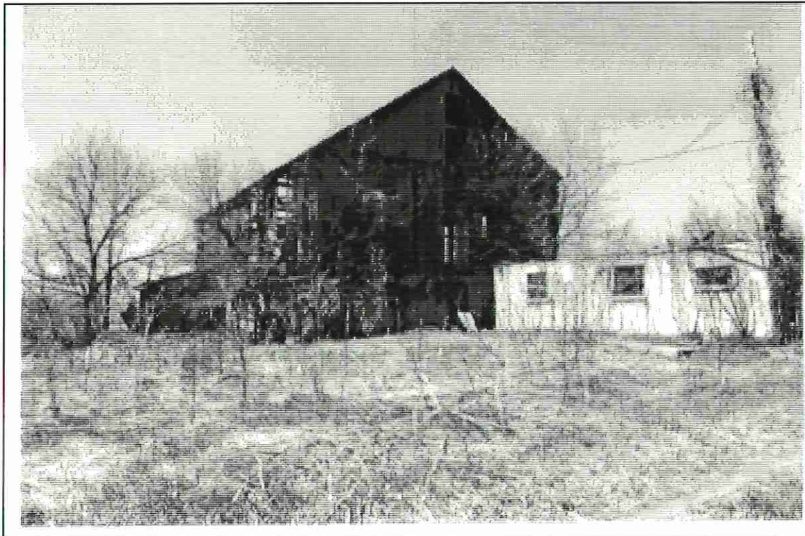
Figure 19. Main Barn, North Face.
