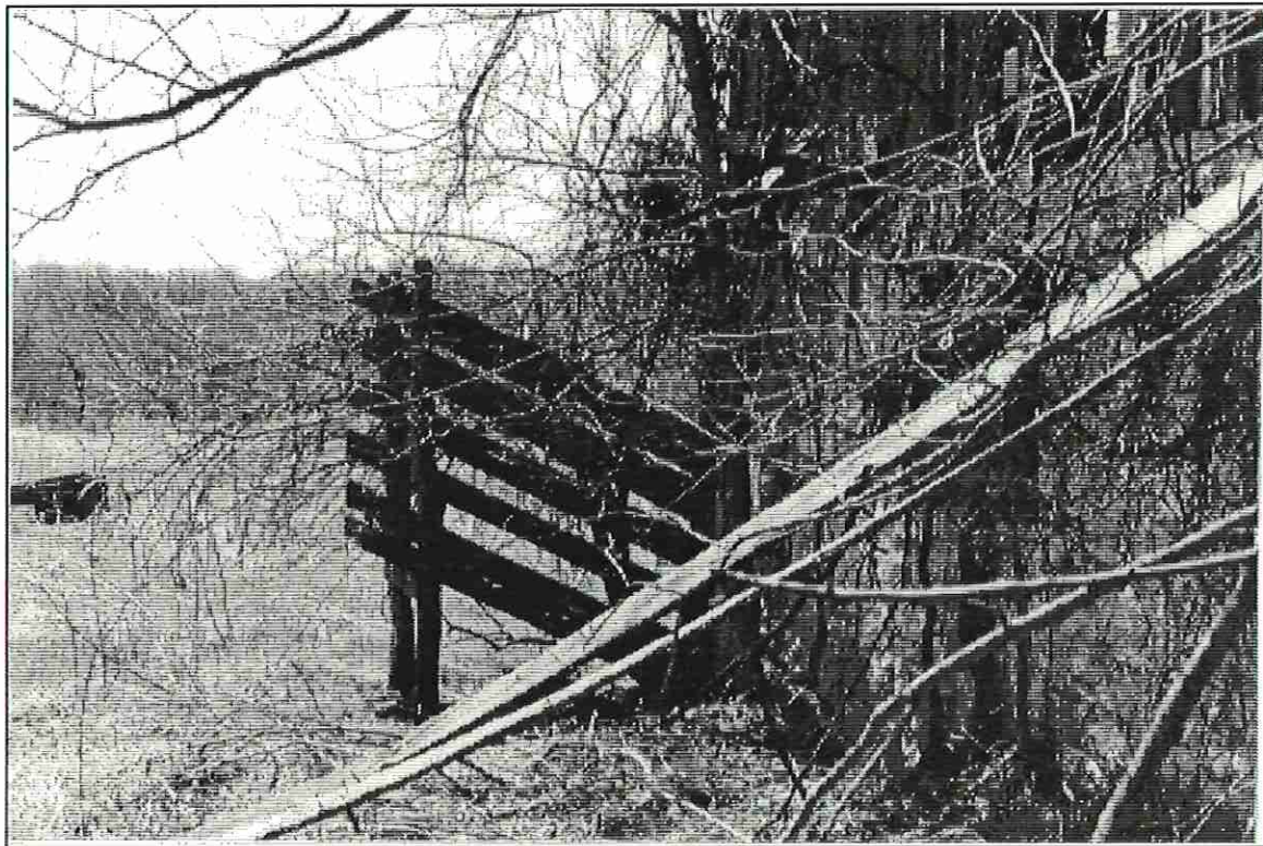
Figure 21. Main Barn, Livestock Chute.
