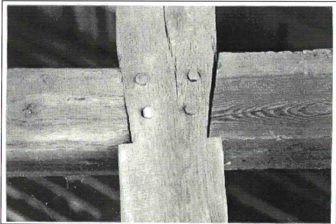
Figure 17. Main Barn, Interior Support Beam.
