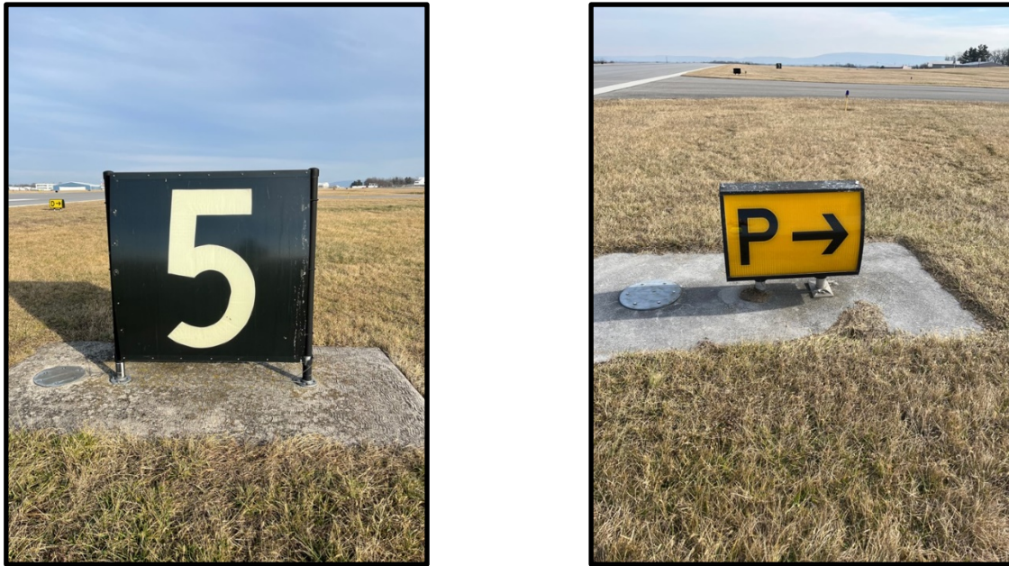
Figure 5.5 – Runway Distance Remaining Sign & Airfield Directional Sign
