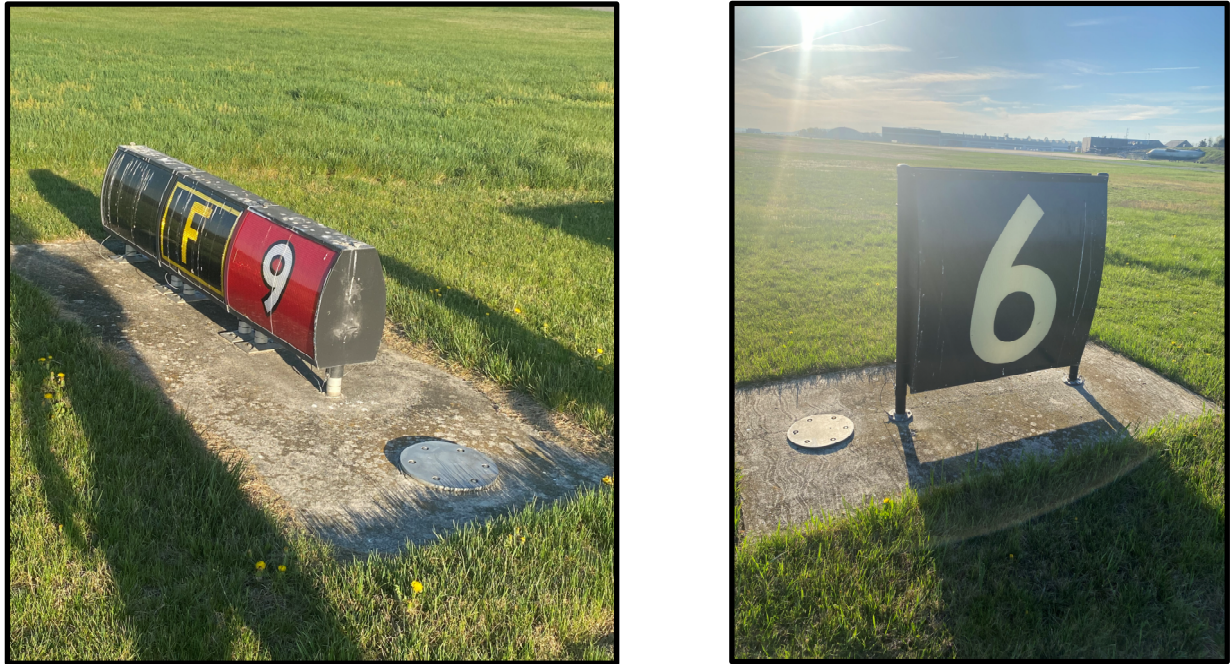
Figure 5.2 – Existing Airfield Signs and Foundations
