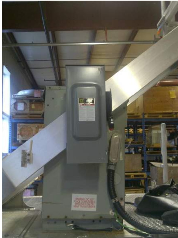
Main Disconnect located at front of trailer
