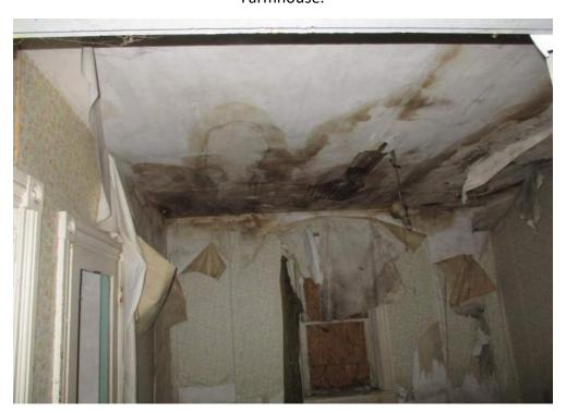
Photo #8: View of mold and water damaged observed in a room located on the  $2^{nd}$  floor of the Farmhouse.
