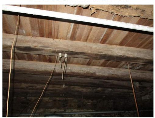
Photo #14: View of rotting wood observed in the basement of the Farmhouse.
