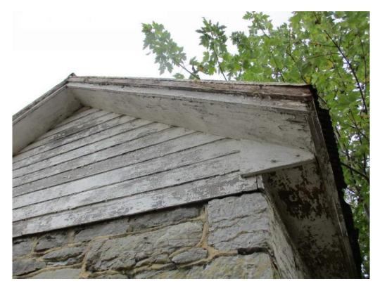
Photo #3: Sample PC #3 –White Wood Roof Overhang sample collected from the Smokehouse exterior.
