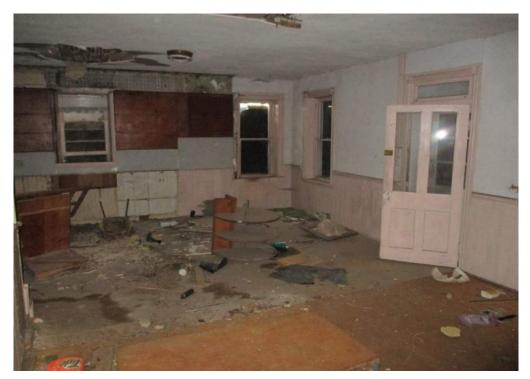
Photo #5:View of water damage observed through out the Kitchen of the Farmhouse.
