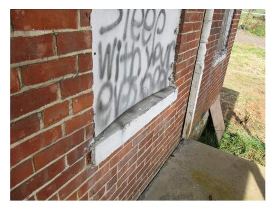
Photo #15: Sample PC #15— White Wood Window Sill sample collected from the Farmhouse's Front Porch.
