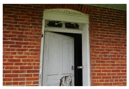
Photo #10: Sample PC #10 – White Wood Window Frame sample collected from the exterior of the Farmhouse's Front Porch above the door.
