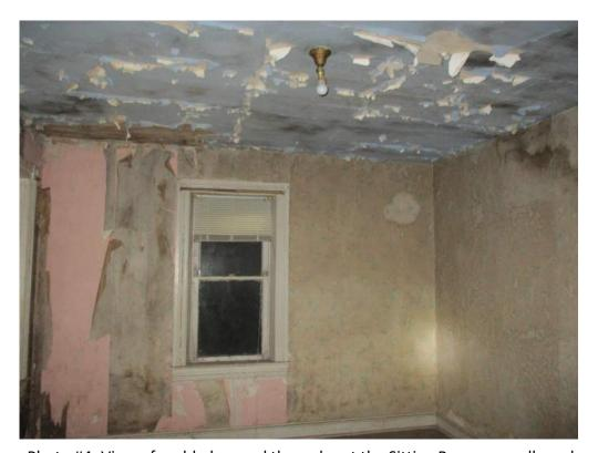
Photo #4: View of mold observed through out the Sitting Room on walls and ceiling in the Farmhouse.
