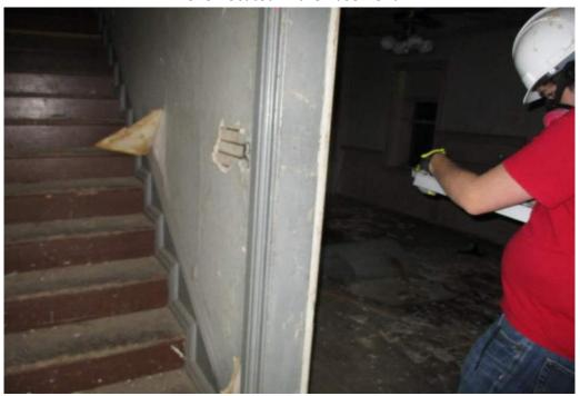
Photo #18: Sample PC #18 – Blue Plaster Wall sample collected from the Front Entrance Wall located in the Farmhouse.
