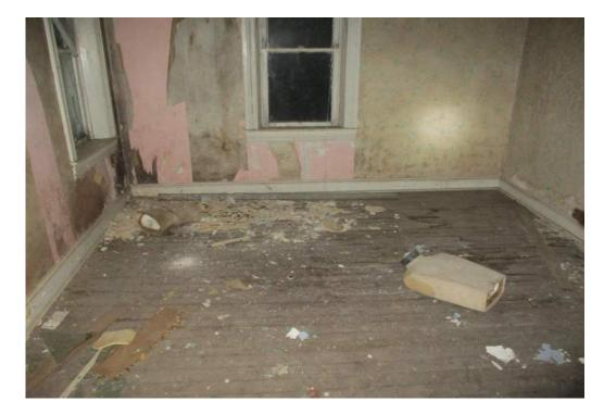
Photo #3: View of the water damage and mold observed in the Sitting Room of the Farmhouse.
