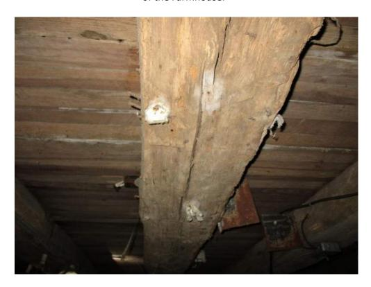
Photo #2: Samples 2A-2C — White insulation collected from a wooden beam located in the basement of the Farmhouse.
