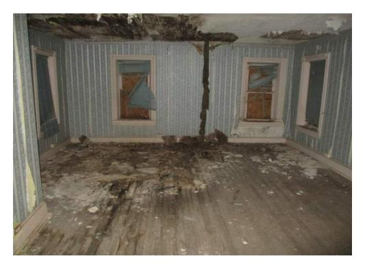
Photo #9: View of mold observed in one of the rooms located on the 2<sup>nd</sup> floor of the Farmhouse.
