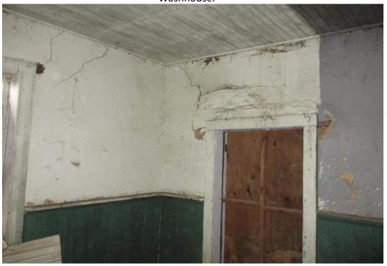
Photo #28: Sample PC #28 – White Plaster Wall sample collected from the Washhouse.
