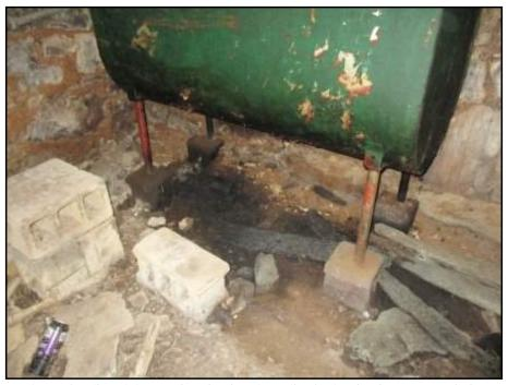
View of soil staining under the heating oil AST in the basement of the Farmhouse.
