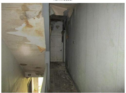
Photo #6: View of mold and water damage observed on the under carriage of the  $2^{nd}$  floor stairs.
