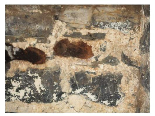
Photo #15: View of mold observed on the wall in the Basement of the Farmhouse.
