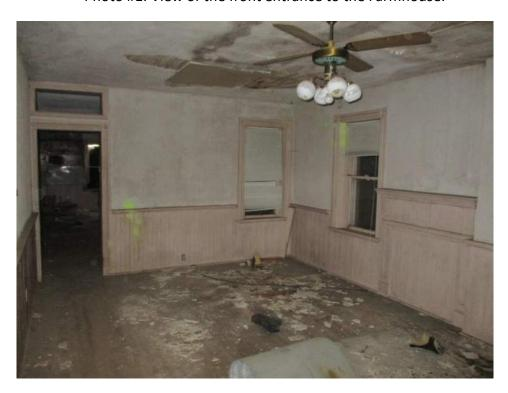
Photo #2: View of the water damage on the ceiling in the Living Room of the Farmhouse.
