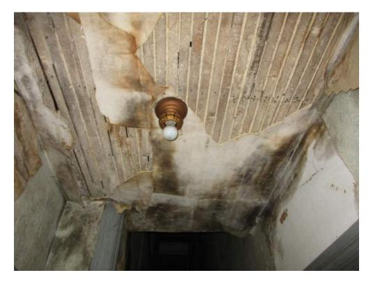
Photo #7: View of mold observed on the 2<sup>nd</sup> floor hallway ceiling of the Farmhouse.
