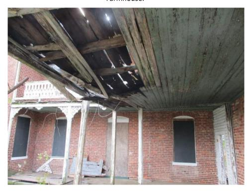
Photo #16: View of rotting wood observed on the exterior of the Farmhouse.
