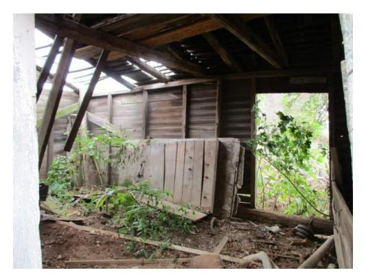
Photo #17: View of rotting wood observed in the Chicken House.
