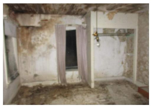
Photo #11: View of mold observed in one of the rooms located on the 2<sup>nd</sup> floor of the Farmhouse.
