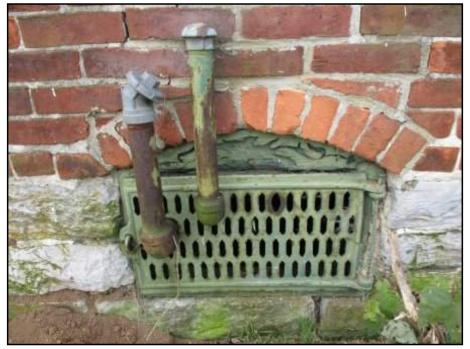
View of AST vent and fill pipes on the north-facing exterior of the Farmhouse.
