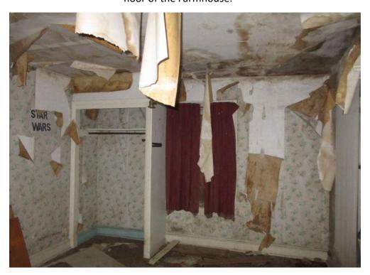
Photo #10: View of water damaged observed in a room located on the  $2^{nd}$  floor of the Farmhouse.
