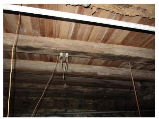
Photo #14: View of rotting wood observed in the basement of the Farmhouse.
