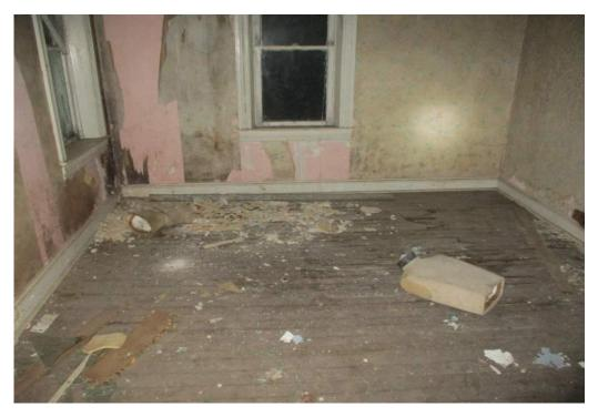
Photo #3: View of the water damage and mold observed in the Sitting Room of the Farmhouse.
