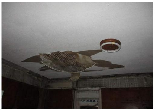
Photo #10: Samples 10A-10B – White Drywall/Texture Ceiling collected from the Kitchen of the Farmhouse.
