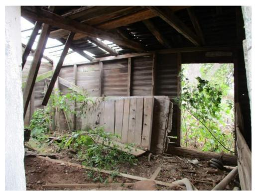
Photo #17: View of rotting wood observed in the Chicken House.
