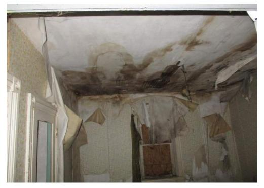
Photo #8: View of mold and water damaged observed in a room located on the  $2^{nd}$  floor of the Farmhouse.
