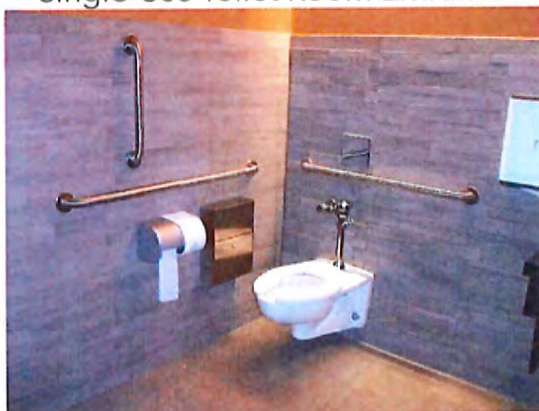
Single-Use Toilet Room Accessible Water Closet
