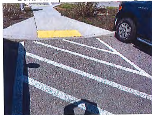
Curb Ramp at Access Aisle
