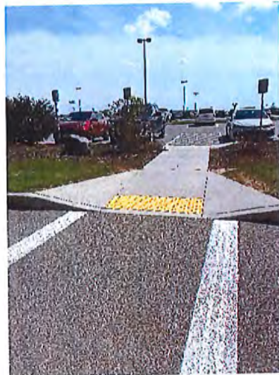
Curb Ramp at Road Crossing
