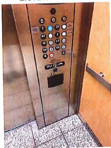
Elevator Control Panel
