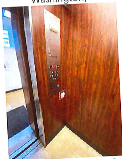
Elevator Control Panel
