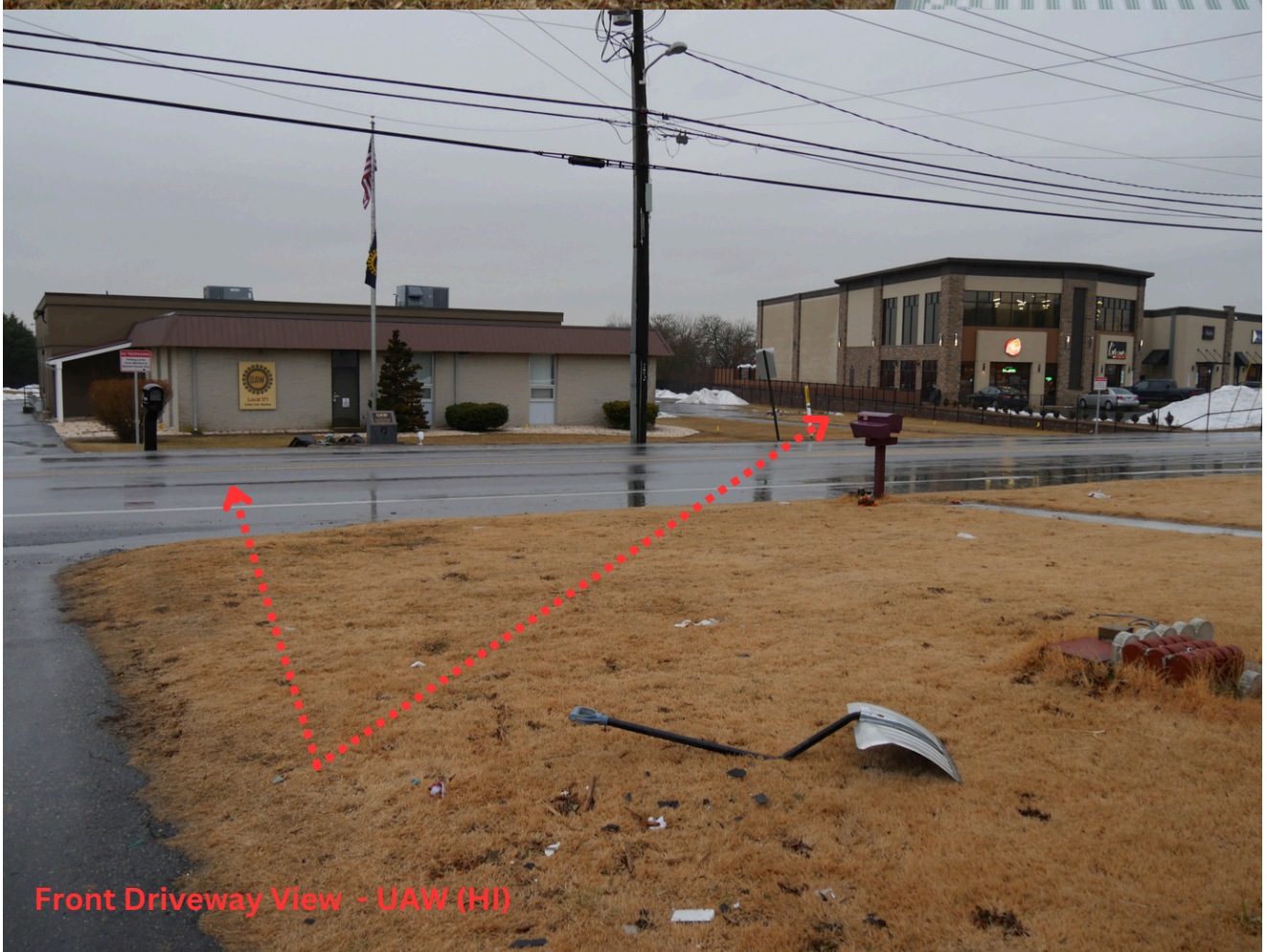
Yard - Disrepair, sheds caving in, litter
