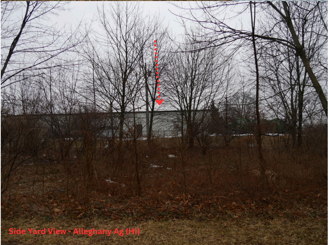
Yard - Disrepair, Sheds Caving In, Litter
