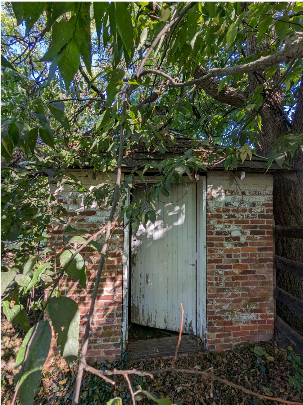
Smokehouse, facing north, pyramidal roof wood shingle and entrance
