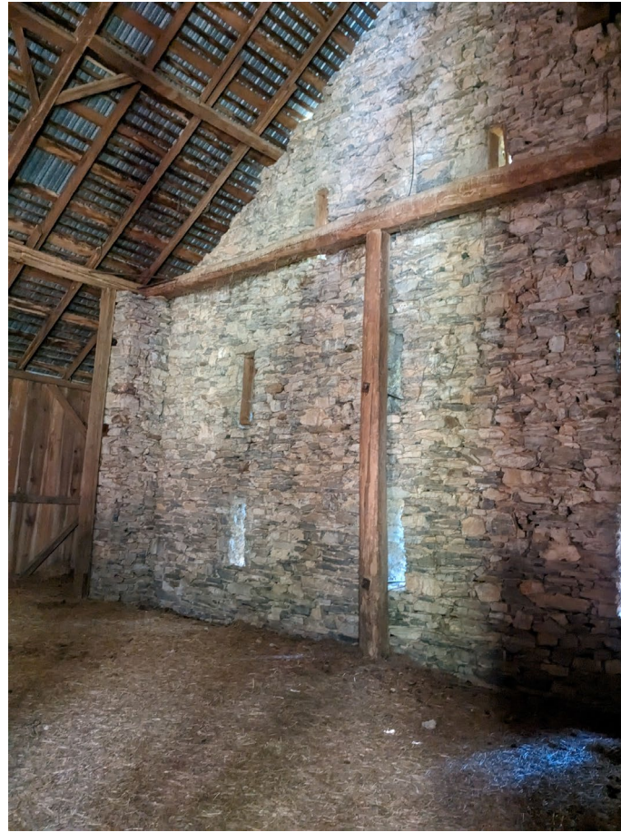
Bank Barn, interior, east wall, venting and timbers with opening
