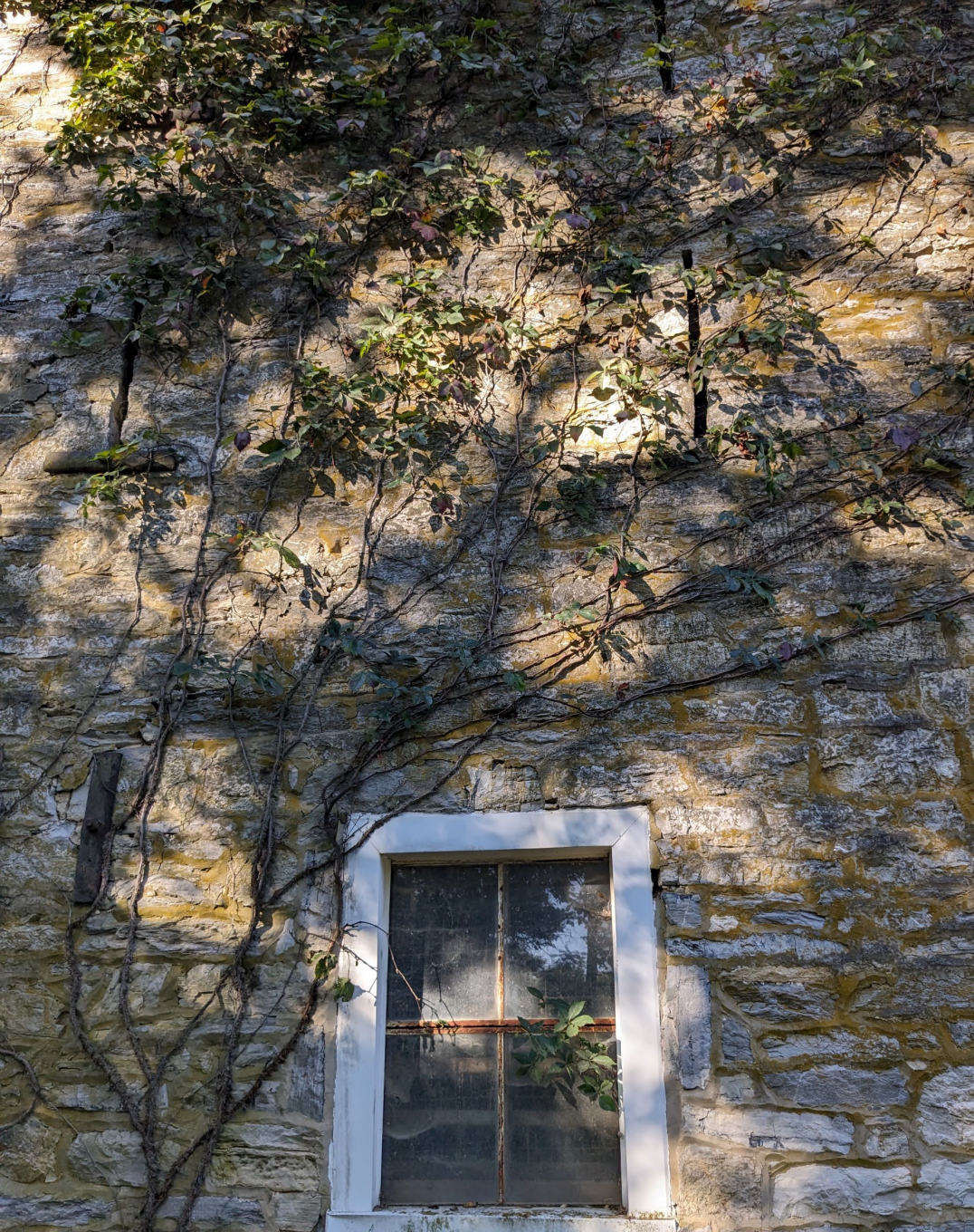
Bank Barn, facing west, windows and venting with metal straps
