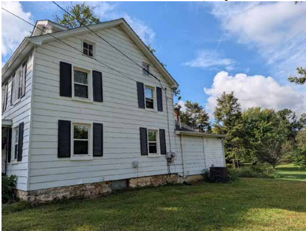
Photo 4: Northside of structure, facing south
