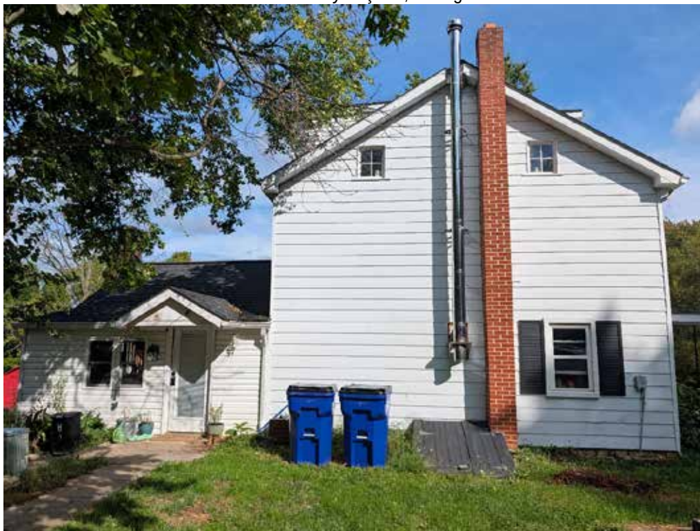
Photo 2: Southside of structure, facing northwest
