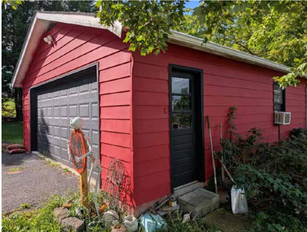
Photo 5: Existing Garage, facing south
