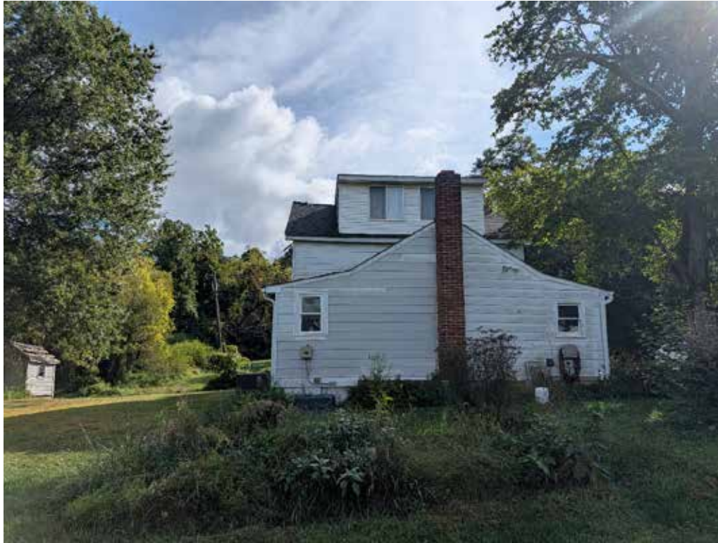
Photo 3: Rear of ell and main structure; facing east
