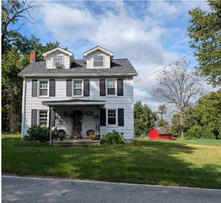
Photo 1: Primary Façade, facing west
