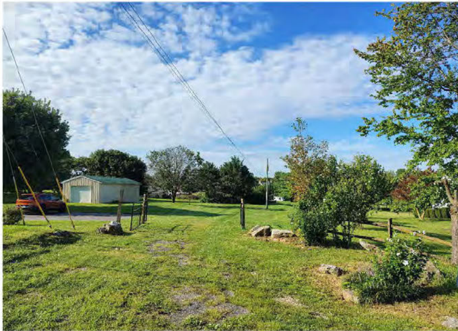
Photograph 13 – Looking south at the potentially NRHP-eligible Stotler Farm (WA-II-144) from the sharp curve in Mt. Aetna Road. View of the house and outbuildings is obscured by dense trees, shrubbery, and modern buildings.
