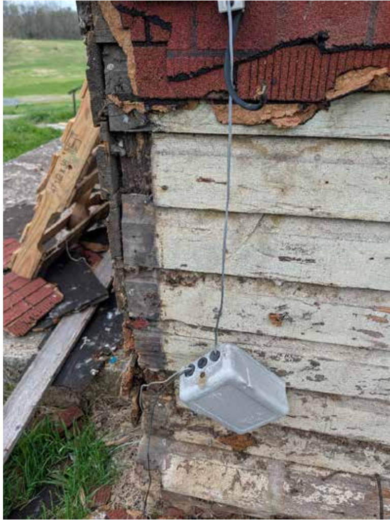
Photo 7: Siding Condition, typical
