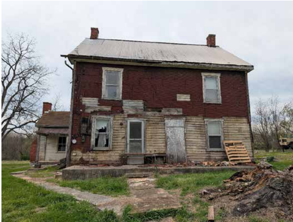
Photo 1: Front façade, facing west
