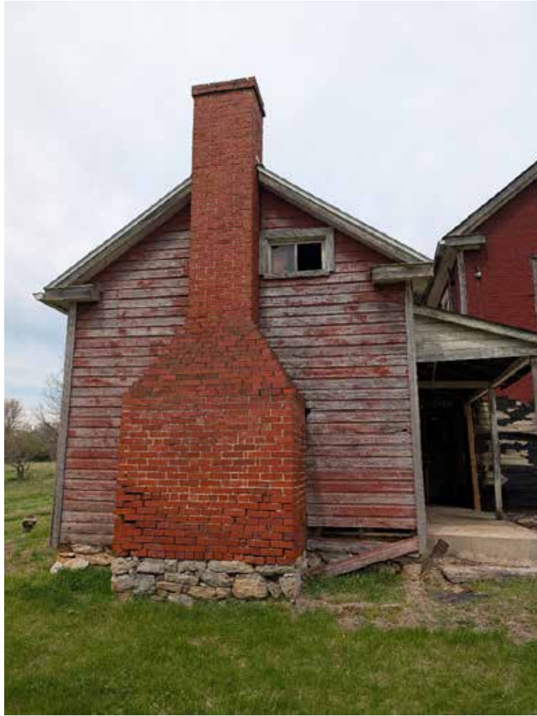
Photo 4: Summer Kitchen chimney, facing north
