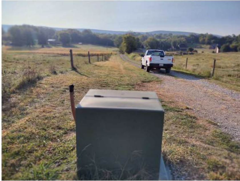
Photograph 11– Looking southeast at the proposed access/utility easement from the ground-based transformer.
