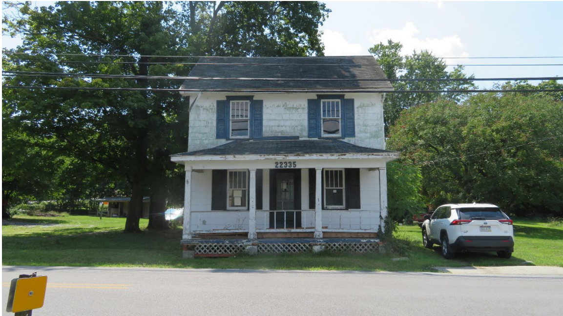
Photo 1: Existing Dwelling, Pre renovation
