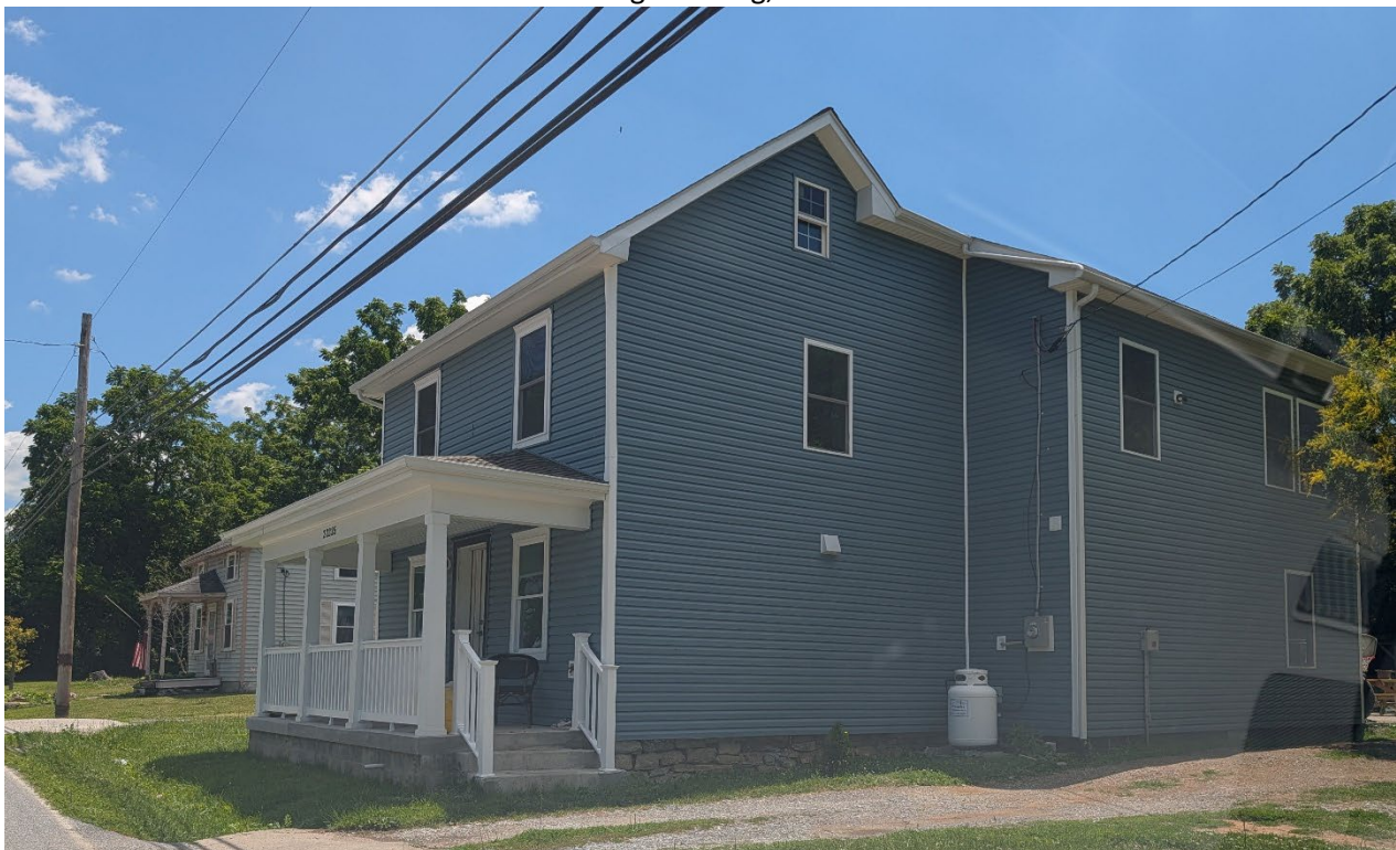
Photo 2: Existing Dwelling, post renovation, taken from Old Georgetown, facing southeast
