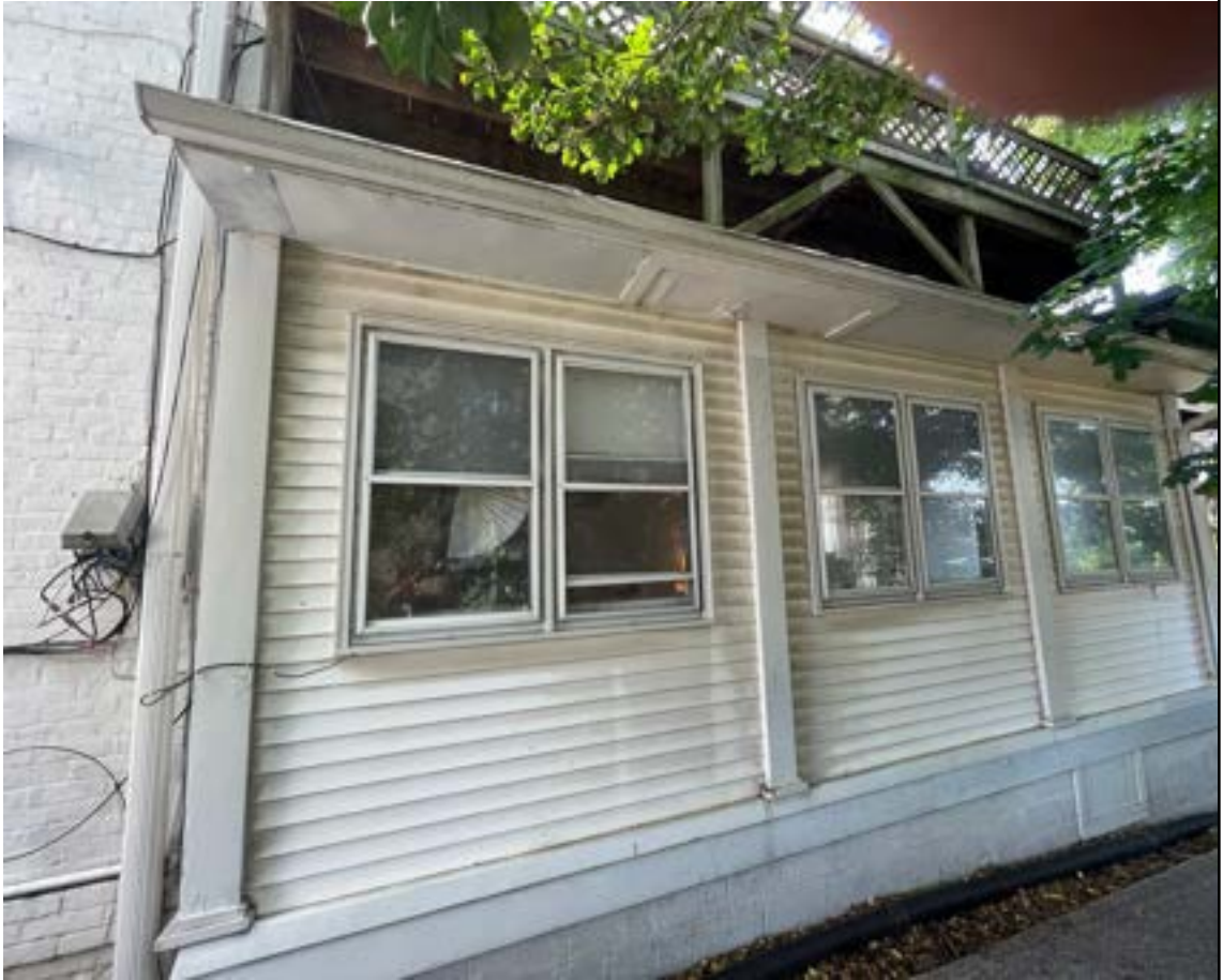
7. Enclosed porch (south side of building)
