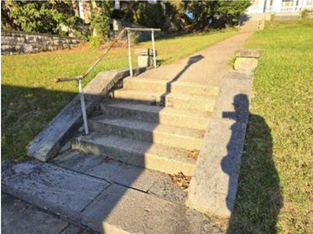
2. Steps leading to sidewalk
