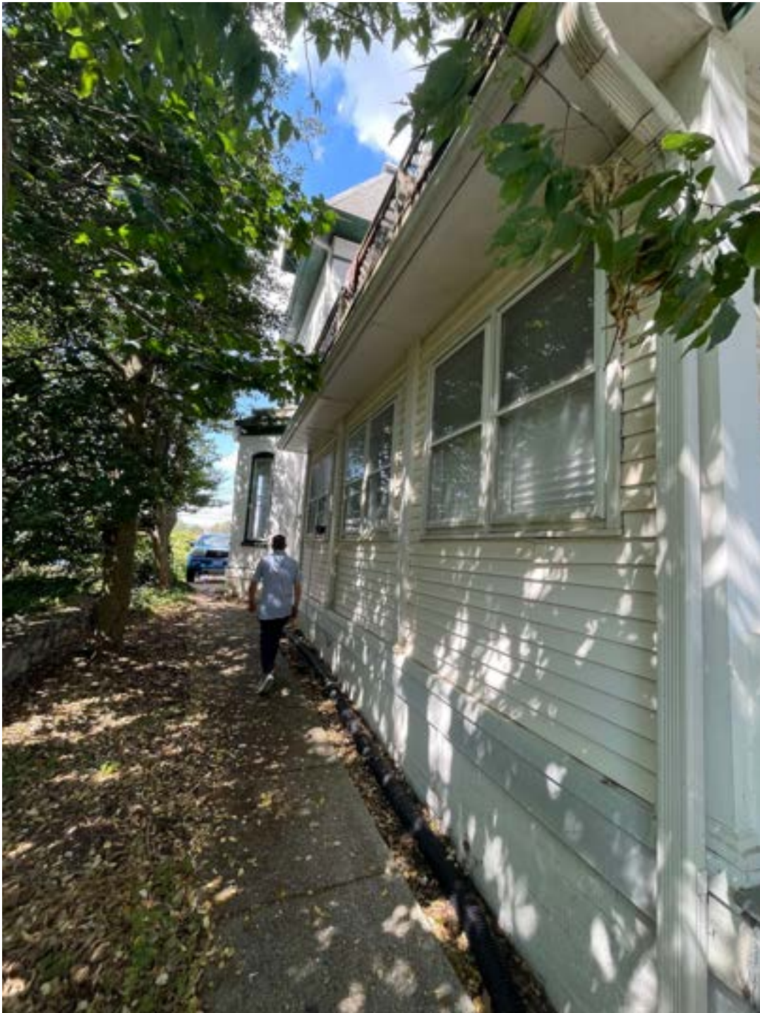
6. Left side of building
