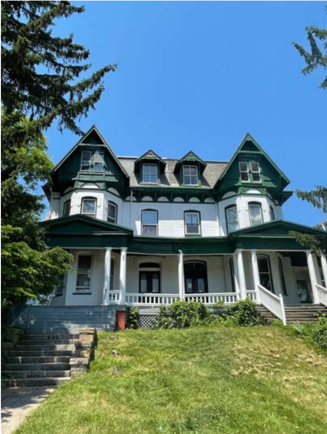
1. Street-facing view of building (left half is 335)
