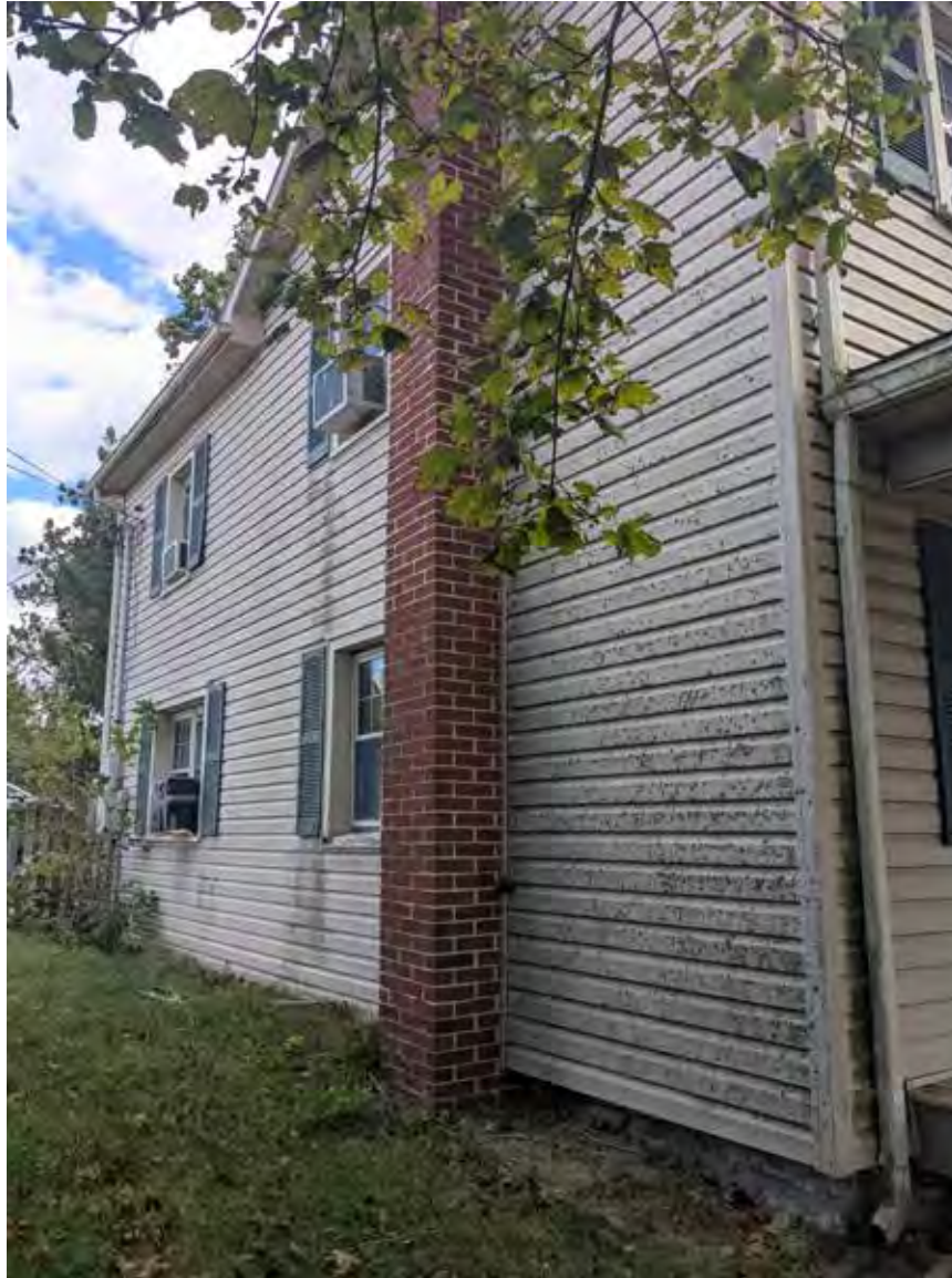
Photo 5: North façade, facing southeast
