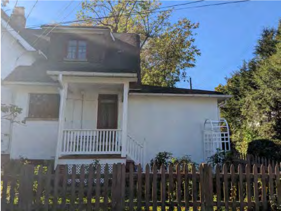
Rear elevation, facing south
