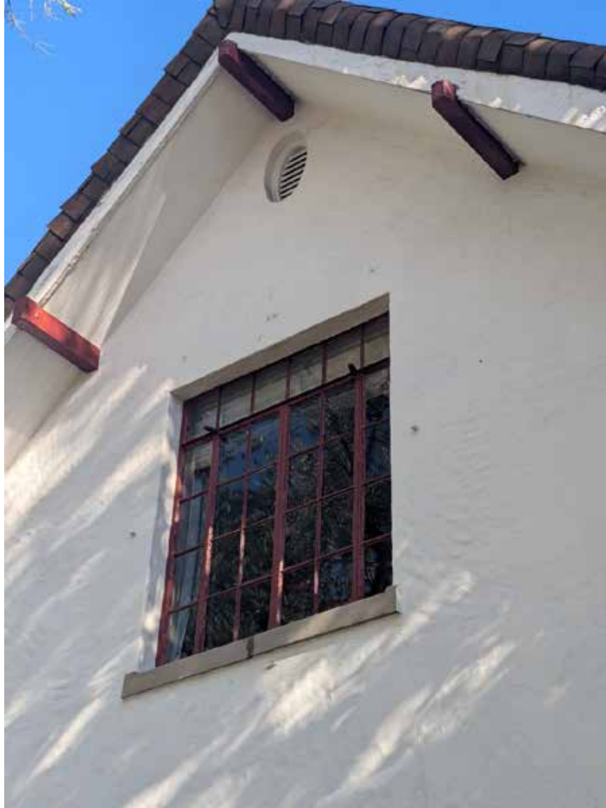
2 nd Story casement window detail, Front Elevation, Facing North
