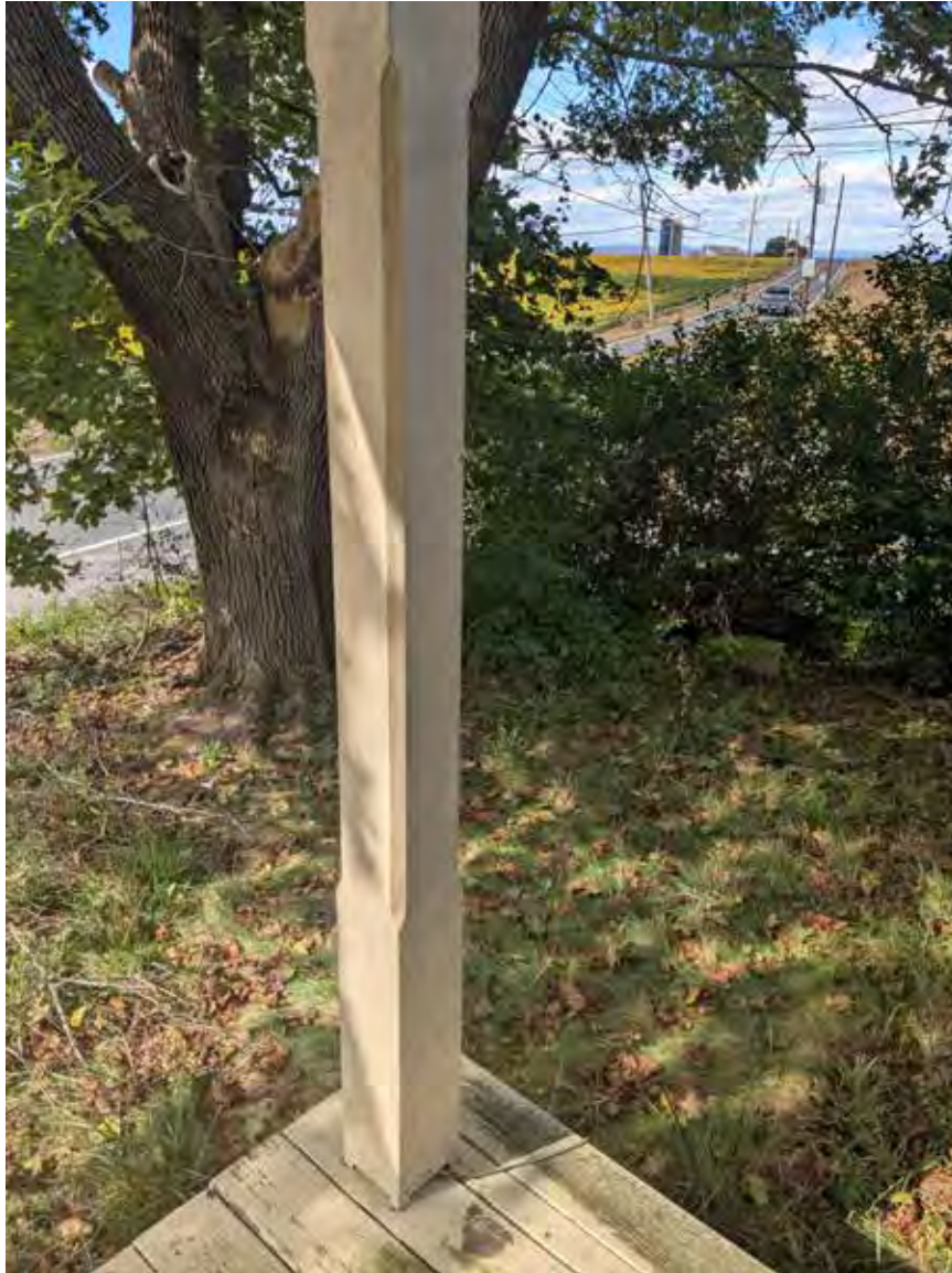
Photo 8: Front porch column detail
