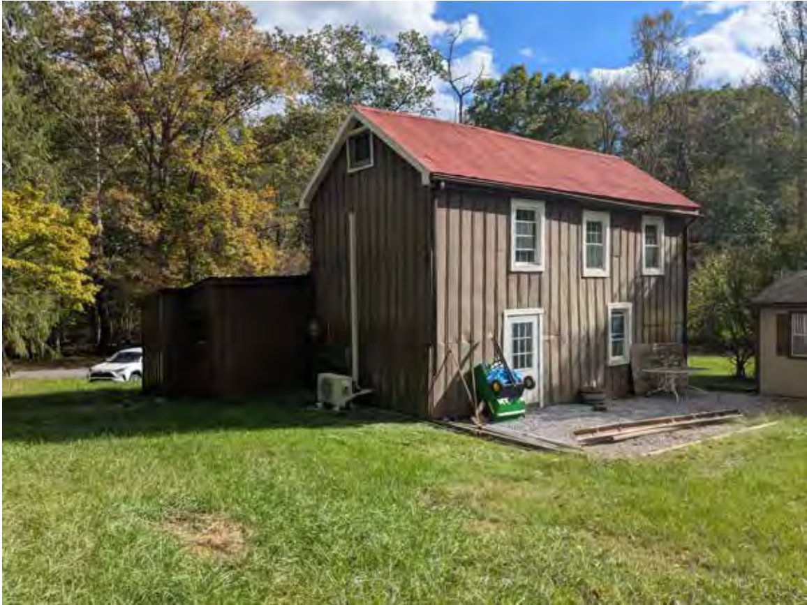
Rear of house, facing south
