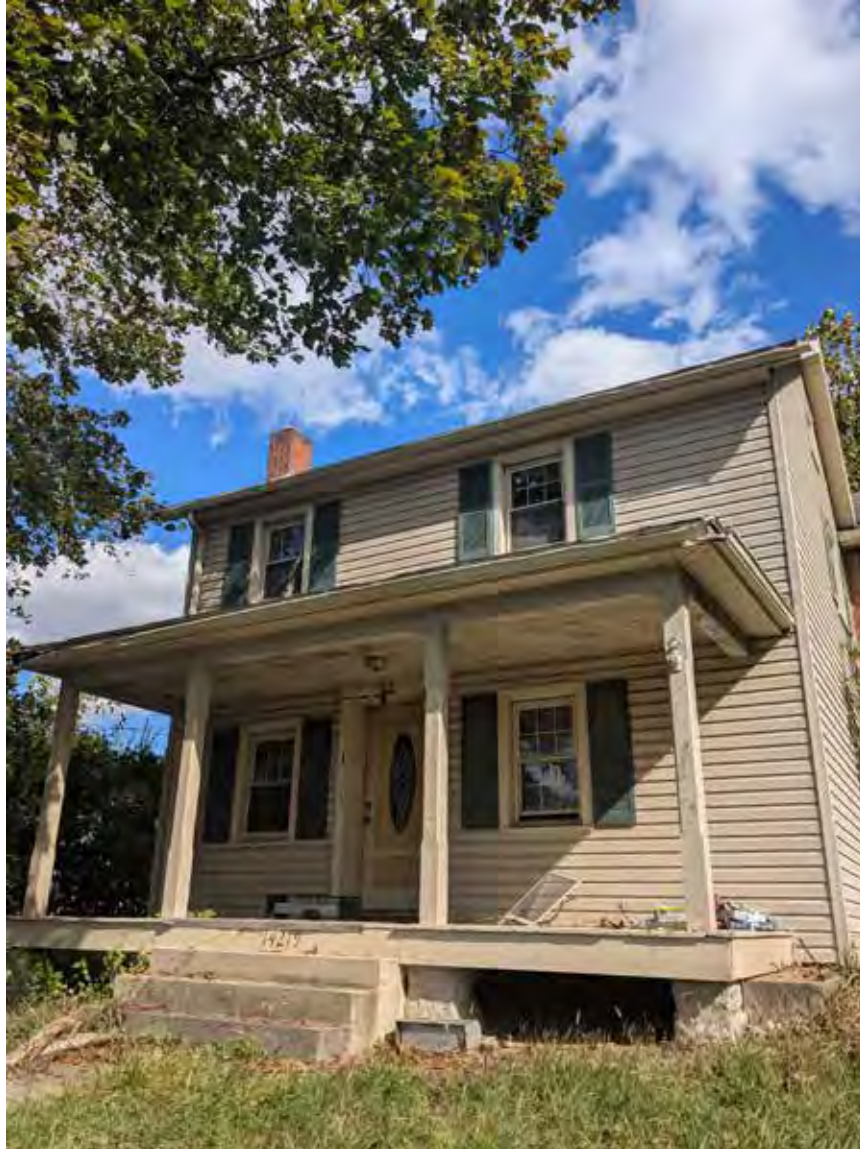
Photo 1: Front Façade, Facing East
