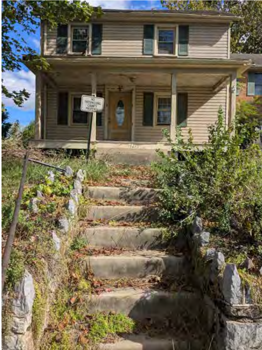
Photo 6: Front Steps; retaining wall detail; facing east
