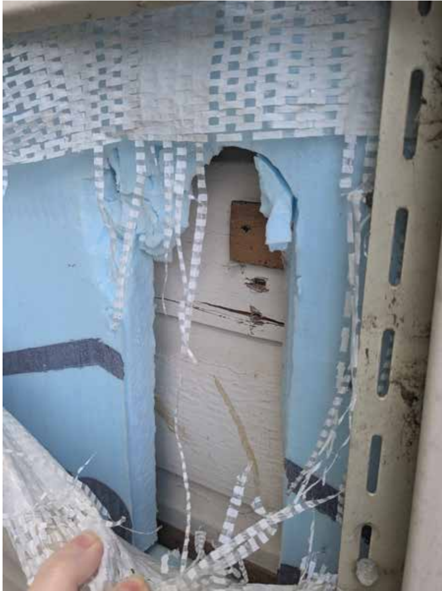
Photo 12: Main dwelling, wood siding detail, photo taken at rear of dwelling
