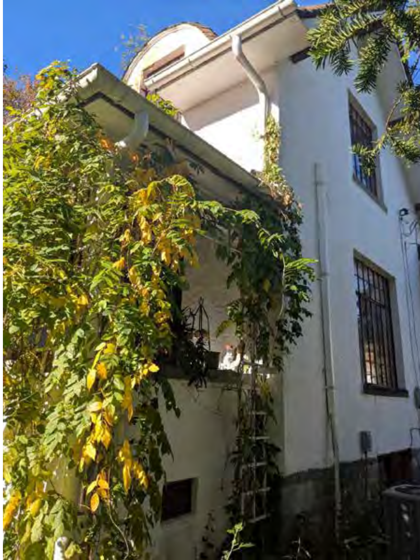
Rear elevation at east porch, facing west
