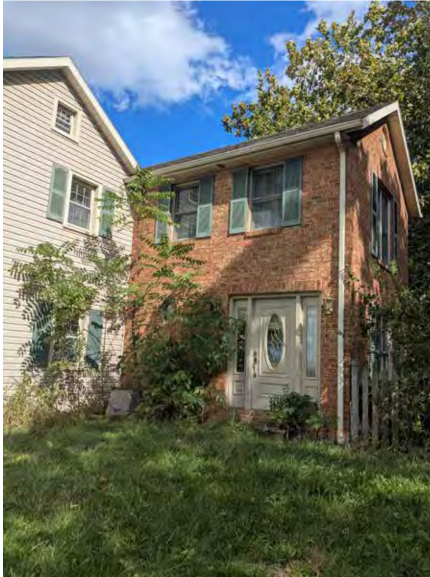
Photo 2: Front Façade Addition, Facing East
