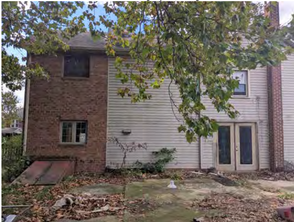
Photo 4: Rear façade, facing west
