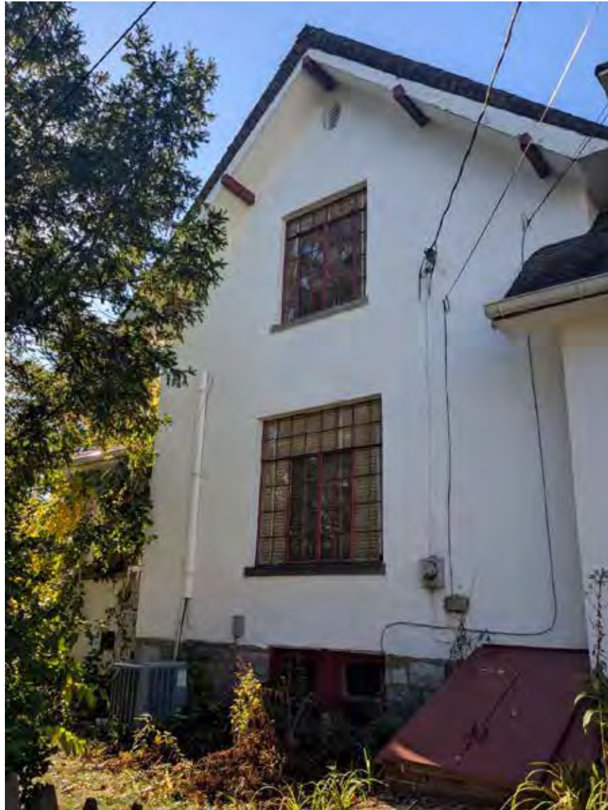
Rear Elevation including 2 nd story casement window, facing south
