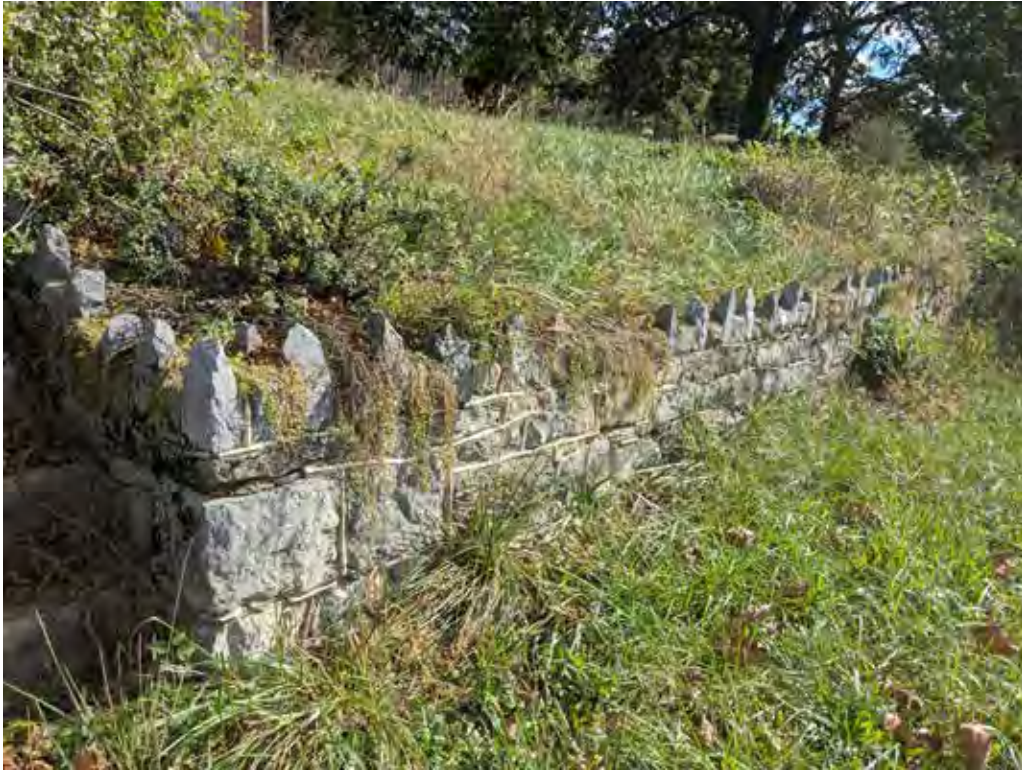
Photo 7: retaining wall detail running south along Maugansville road; facing south
