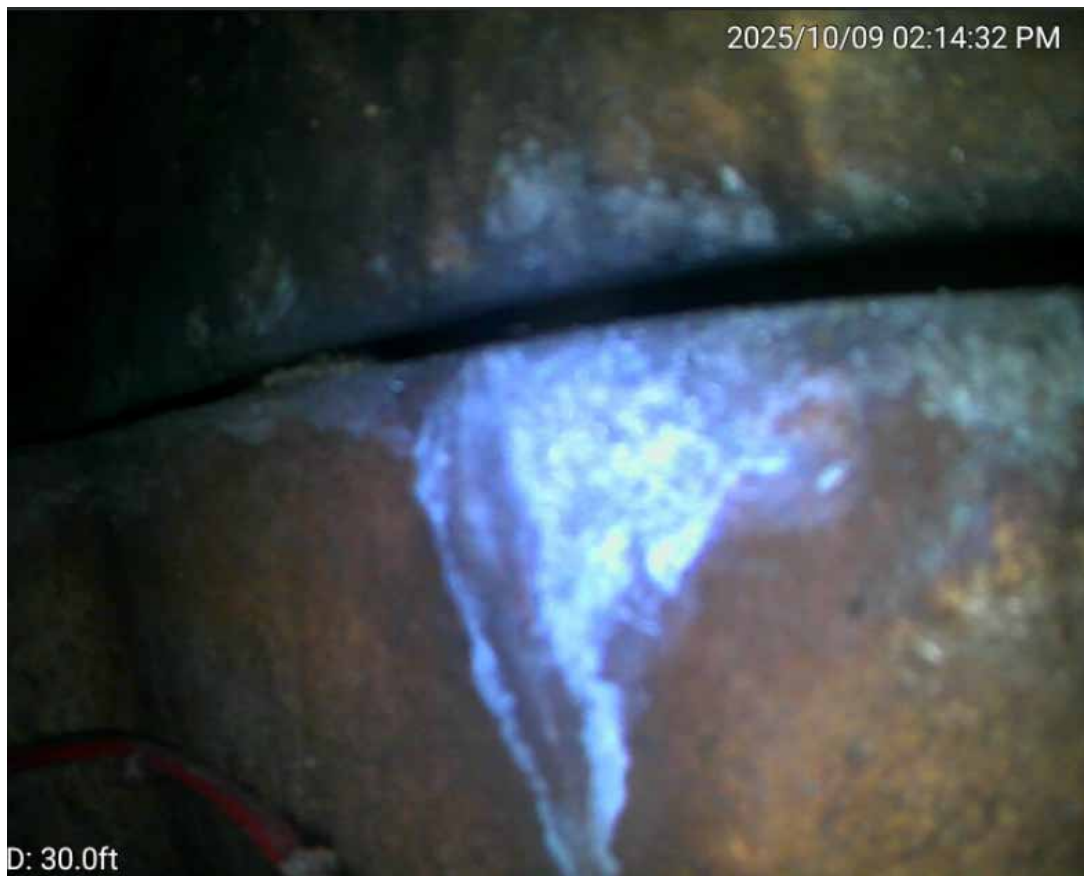
2-3, Chimney tile condition at 30 feet
