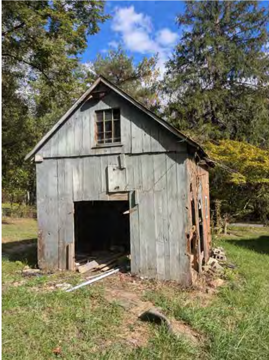
Barn, facing east
