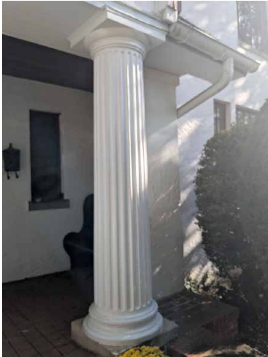
Front porch column detail, facing northeast
