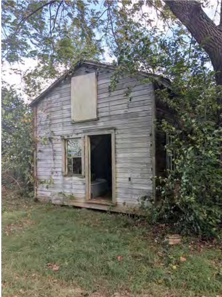
Photo 9: Outbuilding to rear of dwelling, northeast property corner; facing east
