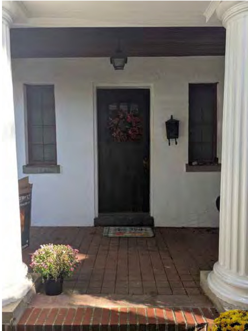
Front Door and casement window detail, facing northeast
