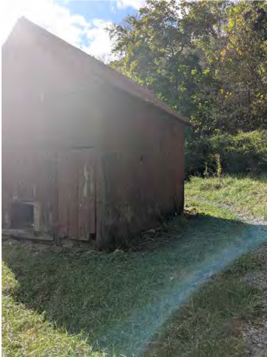
Barn, facing southwest
