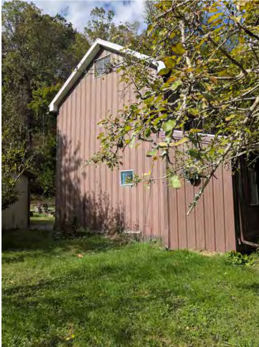
Left side of house, facing north
