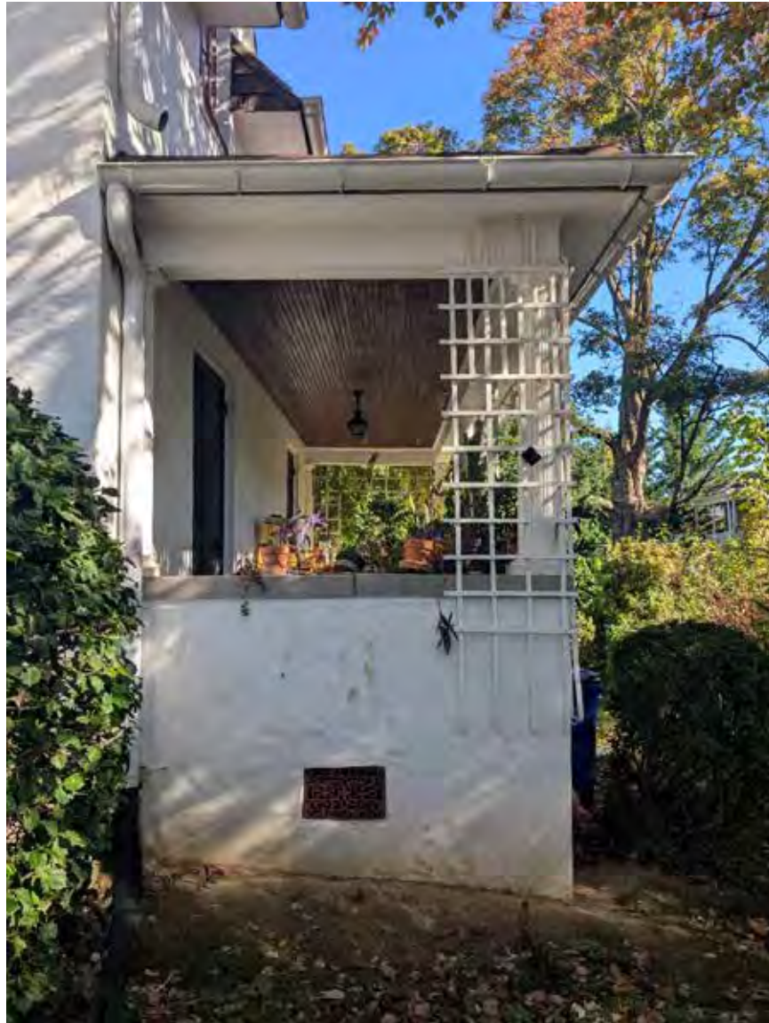
Right elevation/east porch as seen from front elevation, facing north
