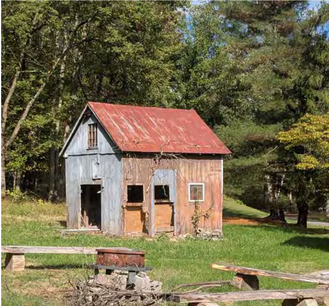
Barn, facing northeast
