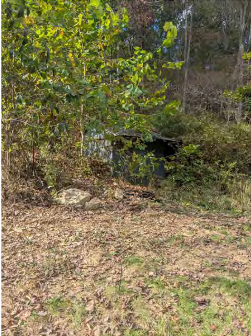
Outbuilding, facing north
