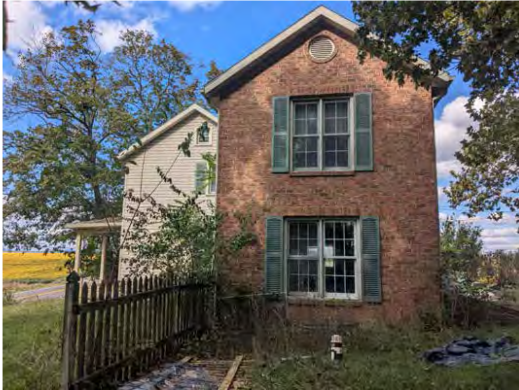
Photo 3: South facing façade, facing north
