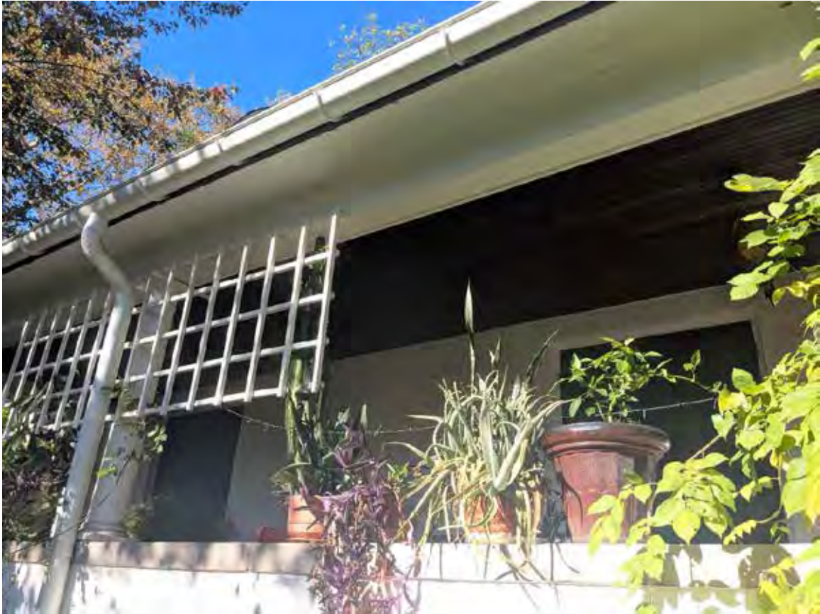
Right elevation/east porch detail facing west
