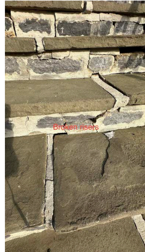
Wink- 817 The Terrace - Broken risers (7)
