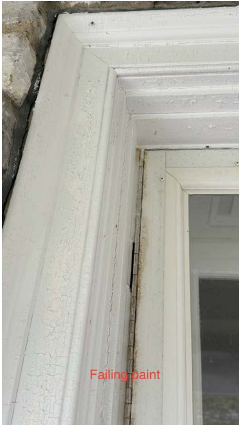
Wink - 817 The Terrace - failing paint (6)
