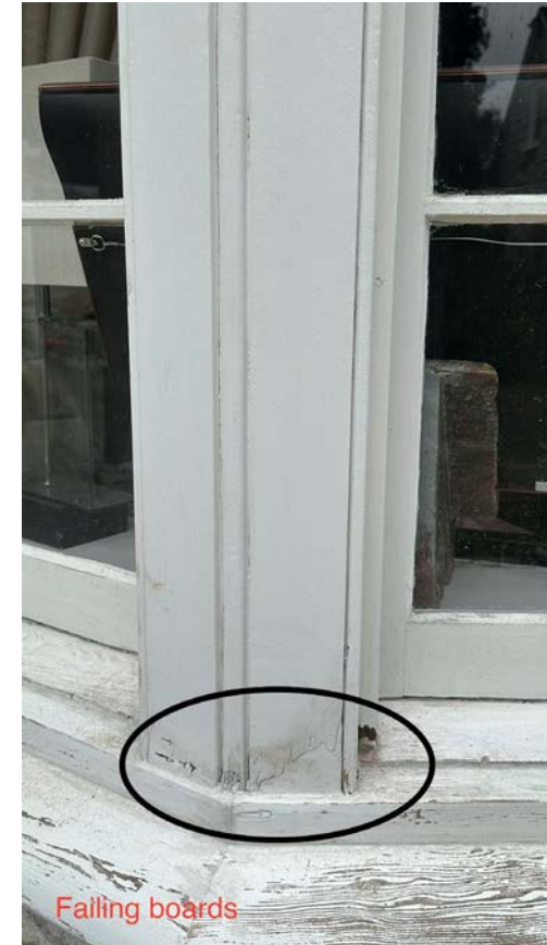
Wink - 817 The Terrace - failing window trim (7)
