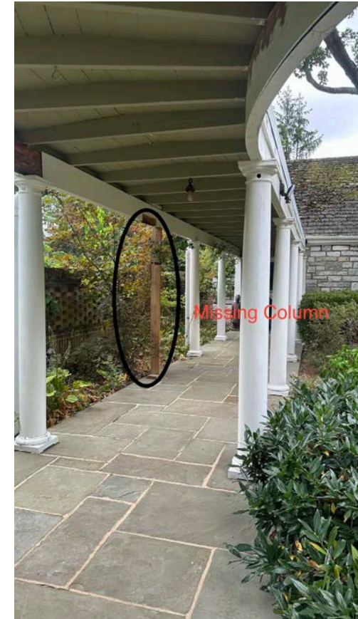
Wink - 817 The Terrace - Missing Column (3)
