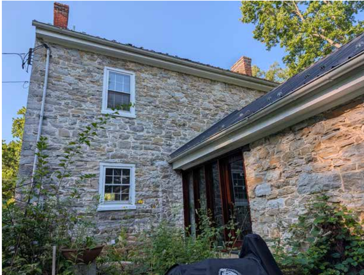
7_Rear Facade, facing S
