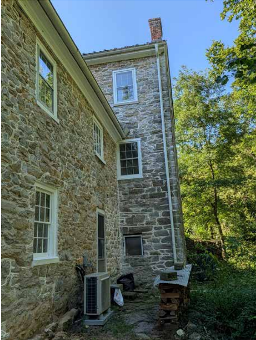
11_Rear Facade, facing south
