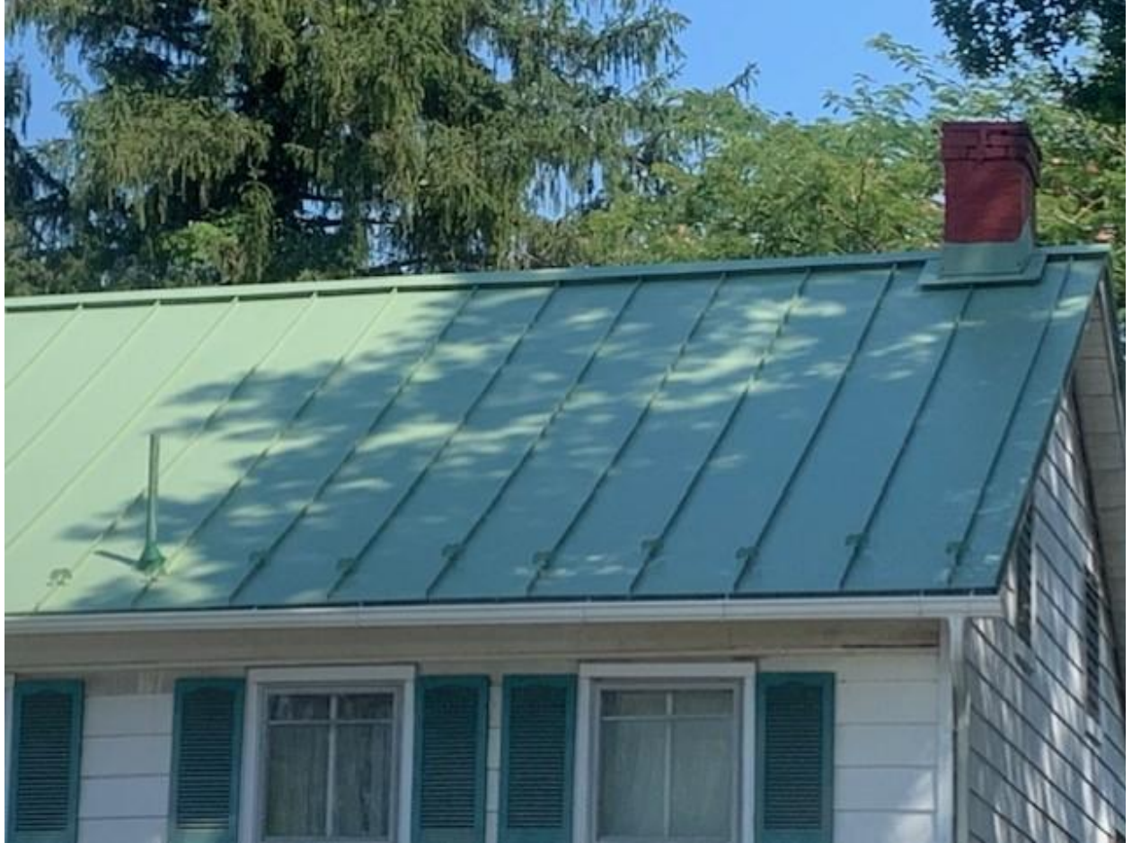
Partial front of house - close up - (after)
