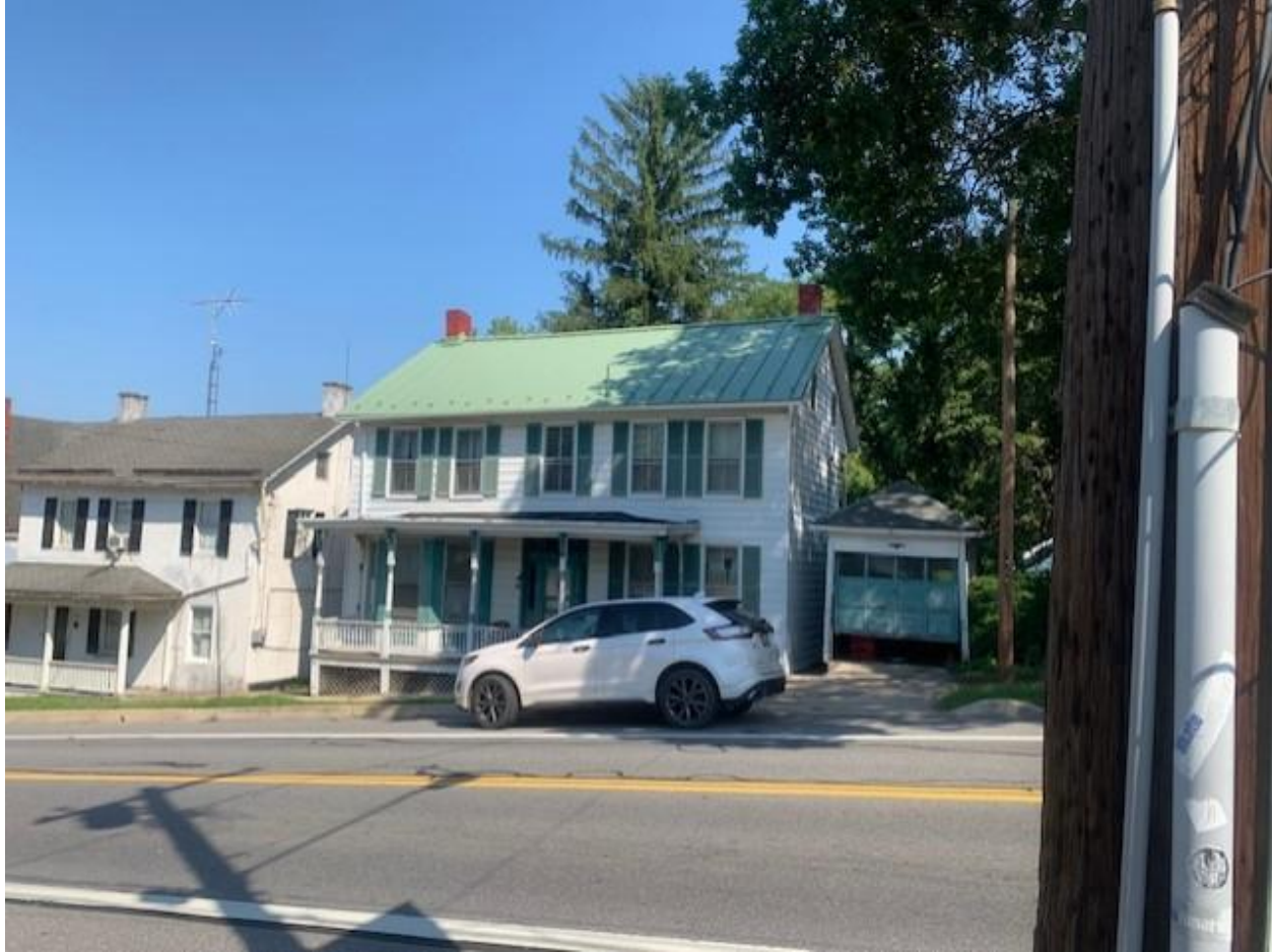
Front of House/Roof (after)
