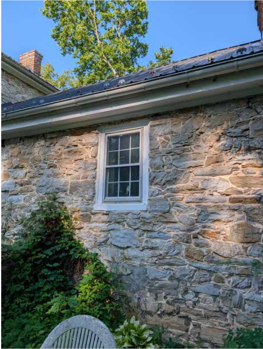
9_original window detail
