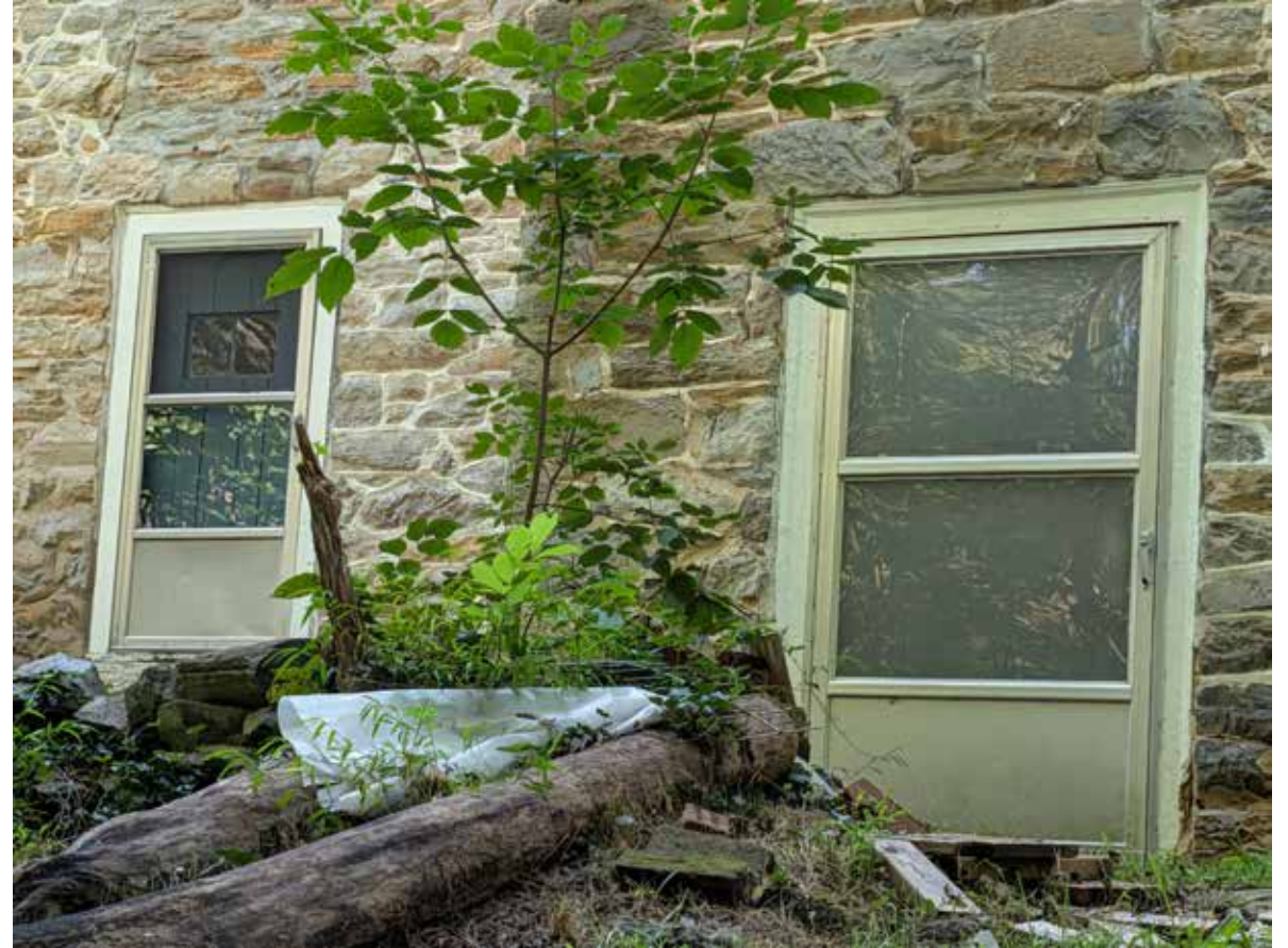
14_ door detail, west side of house, facing northeast
