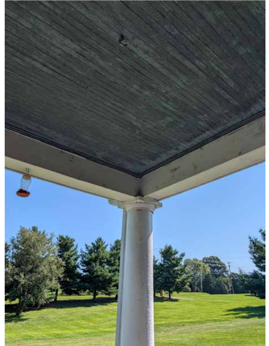
16_front porch ceiling
