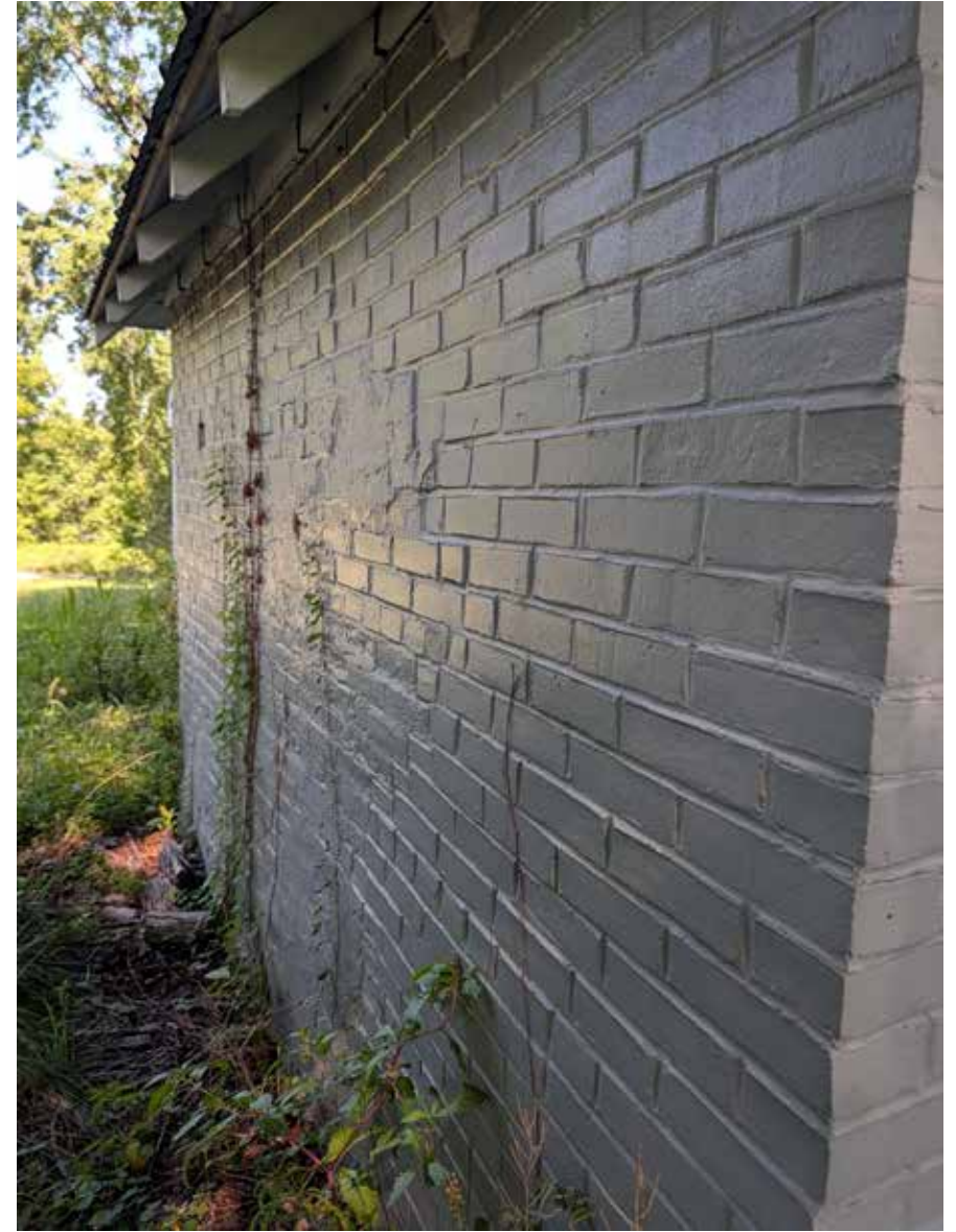
19a_brick detail at smokehouse
