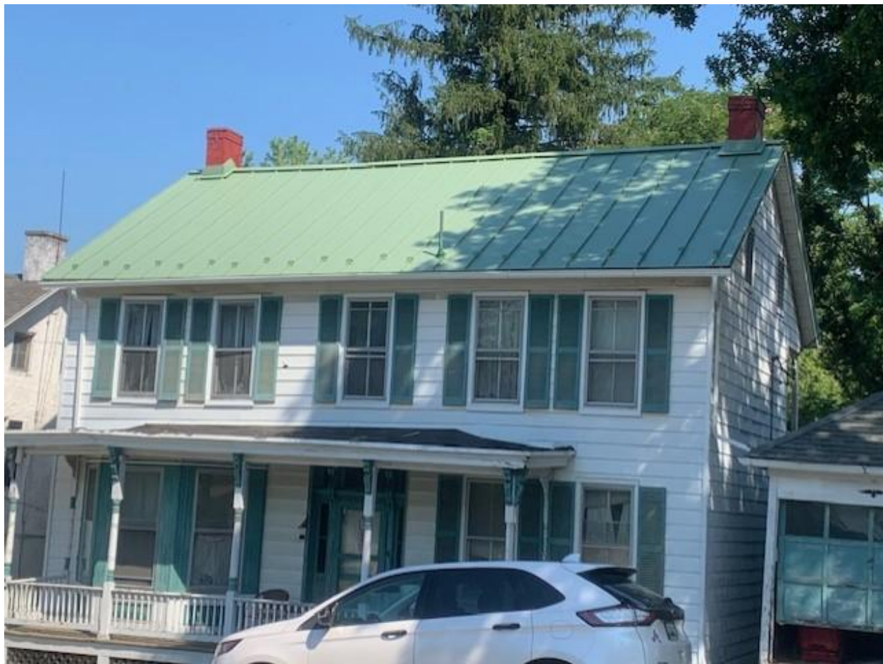
Front of house/roof (After)
