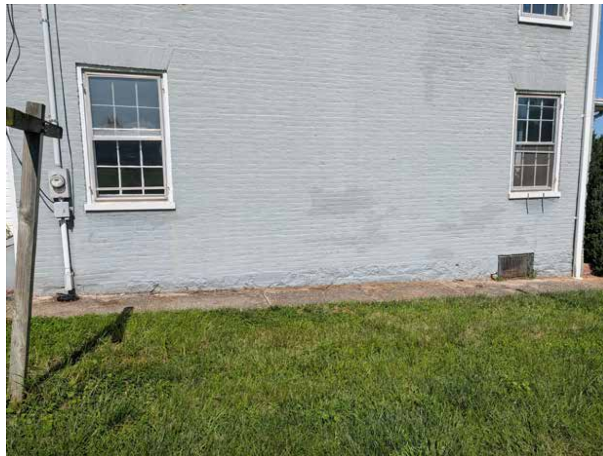
6_left side of house foundation
