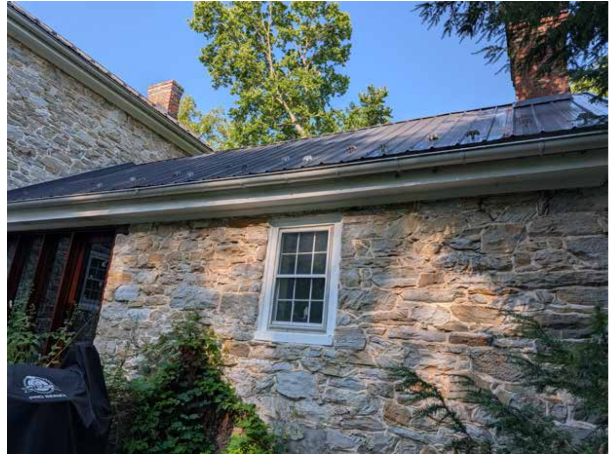
8_original window detail
