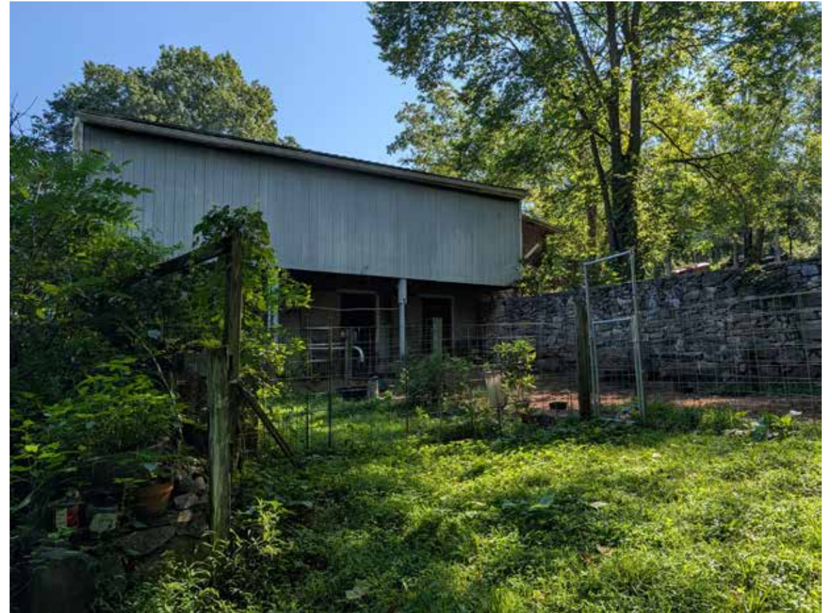
20_barn_southwest facade, facing northeast
