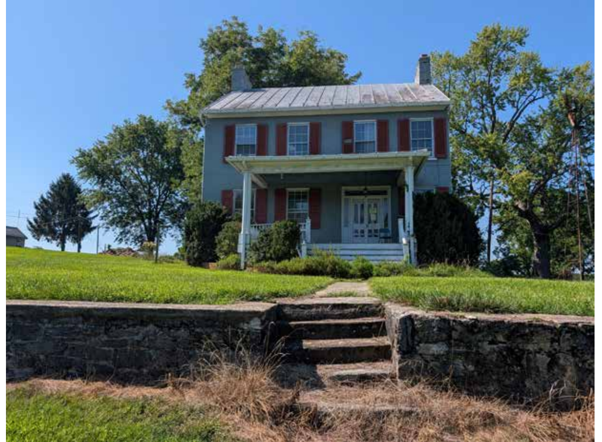
2_Front Facade with Retwall
