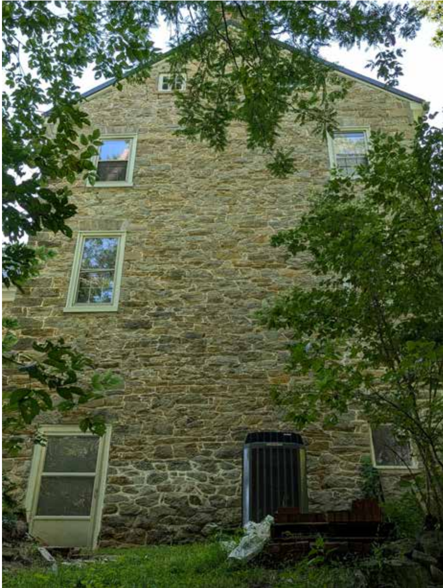
15_western side of the structure, facing east
