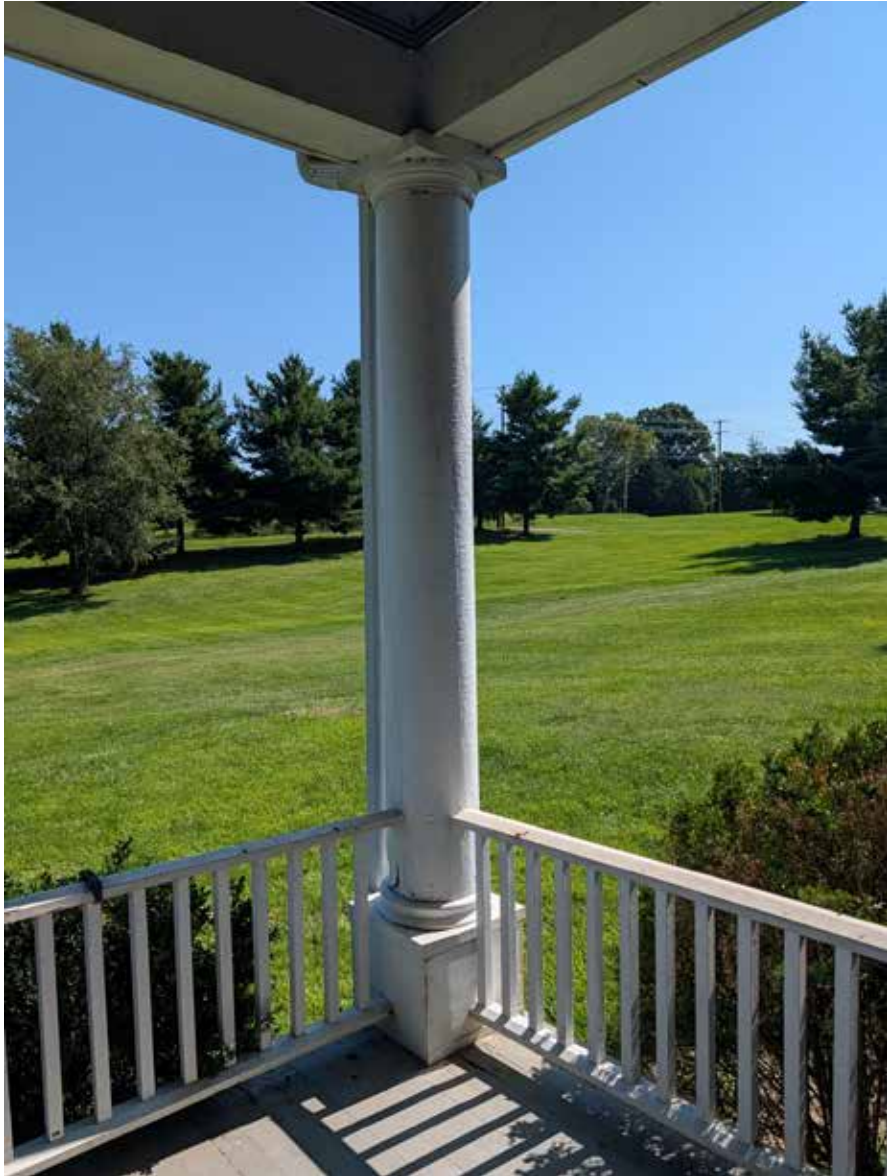
17_front porch column_railing
