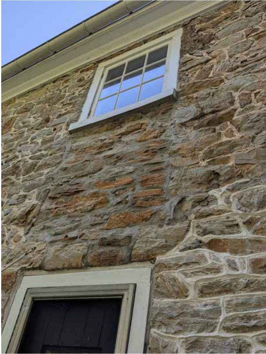
13_facing SE, rear section at filled opening
