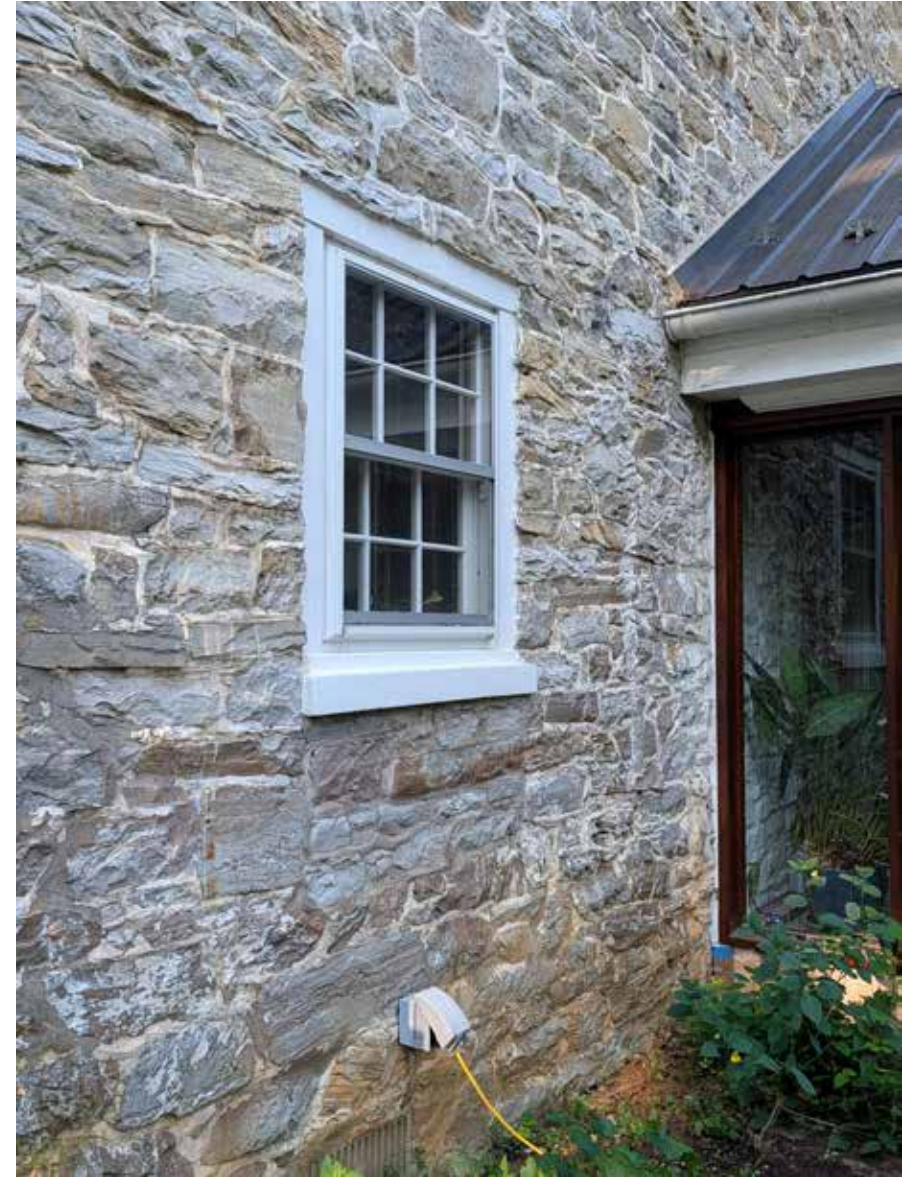
6_window detail, rear facade
