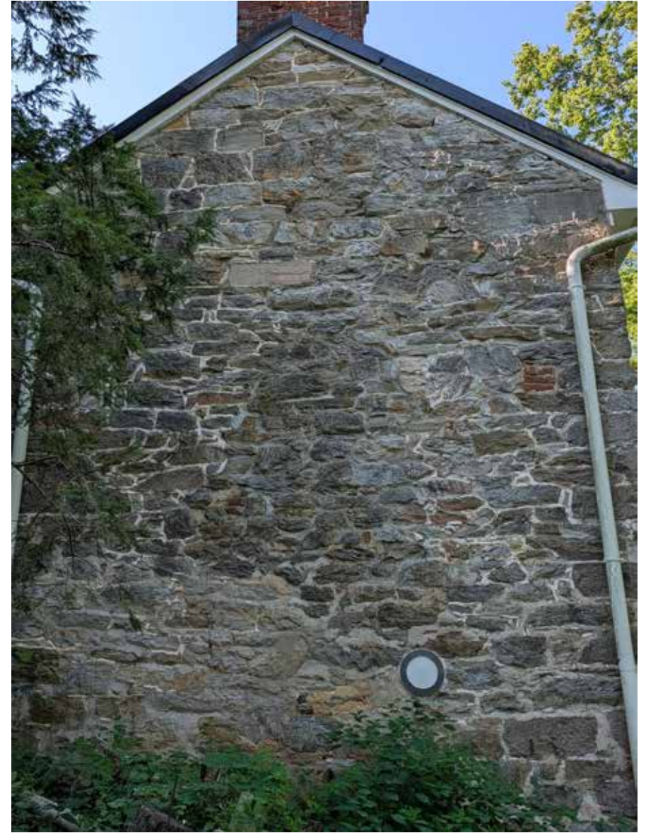
10_rear facade at northernmost end, facing SW
