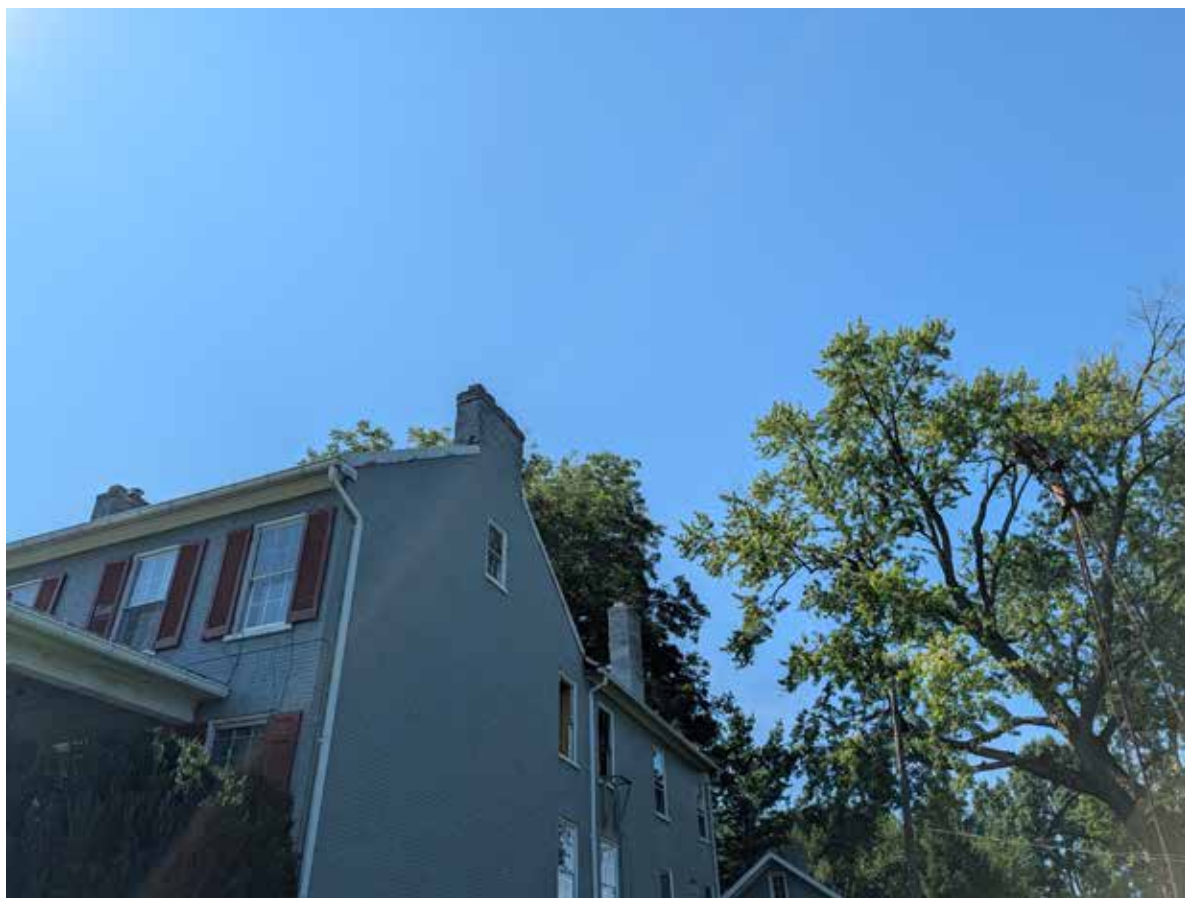
11_right facade at chimney
