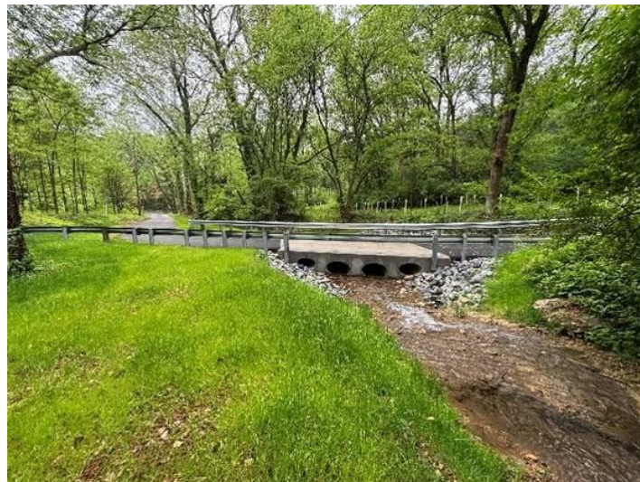
Remsburg Road Culvert Replacement project
