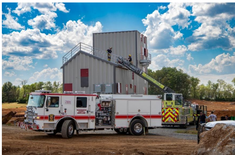
New burn building at Public Safety Training Center
