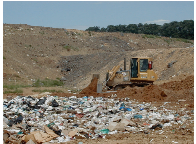
Providing daily cover on 40 West Landfill waste stream
