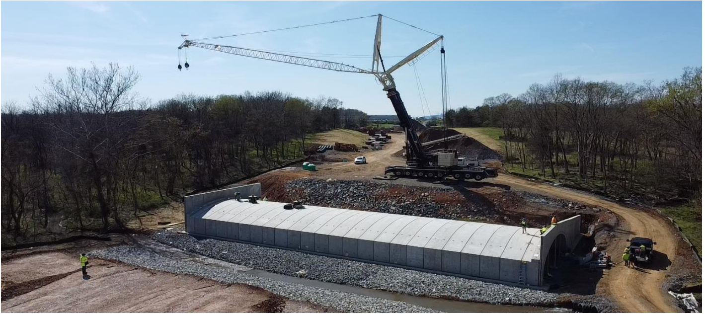
Halfway Boulevard project – bridge construction phase
