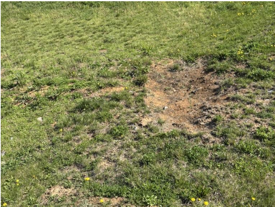
Eroded channel end
