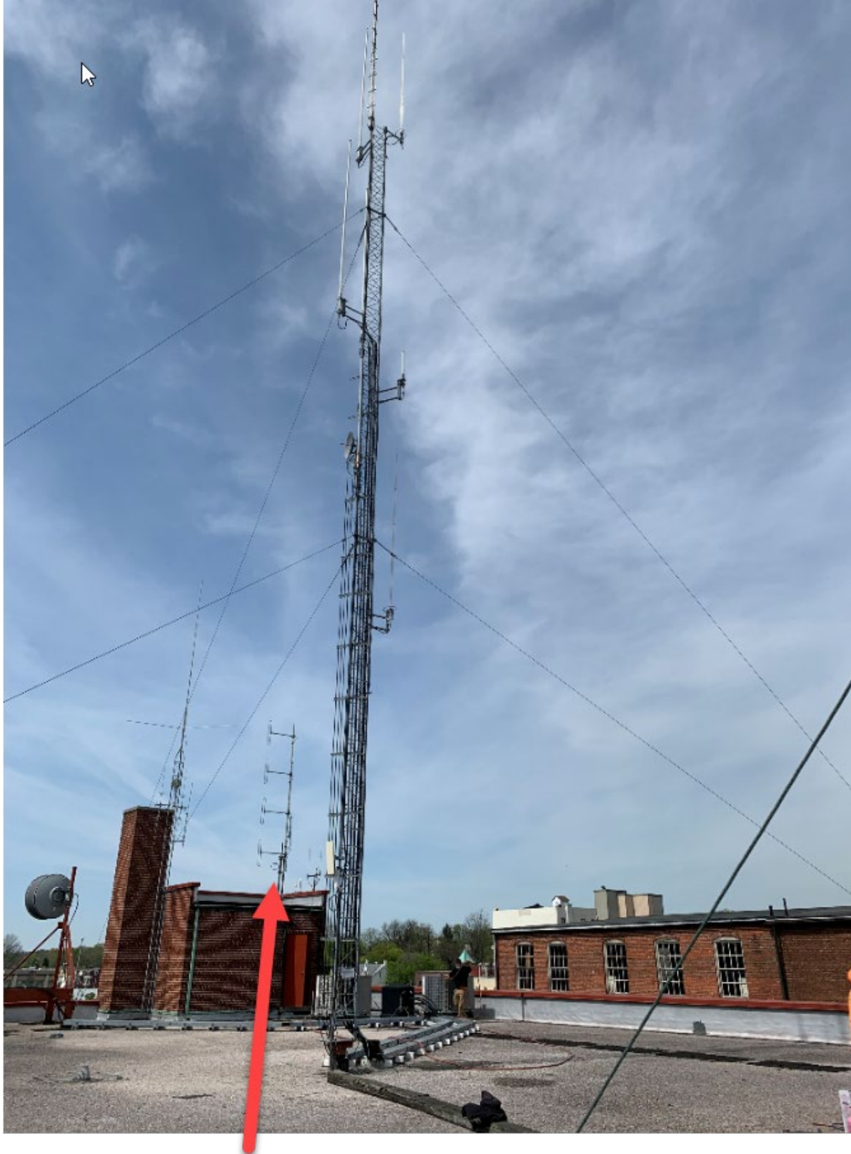
Elevator Shaft Antenna
