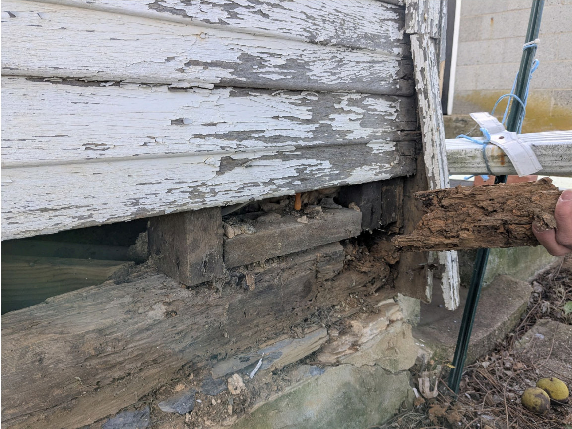
Addition log foundation/stone (western façade) condition
