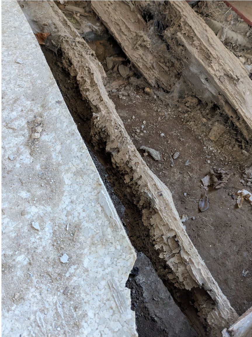
Addition floor beam condition
