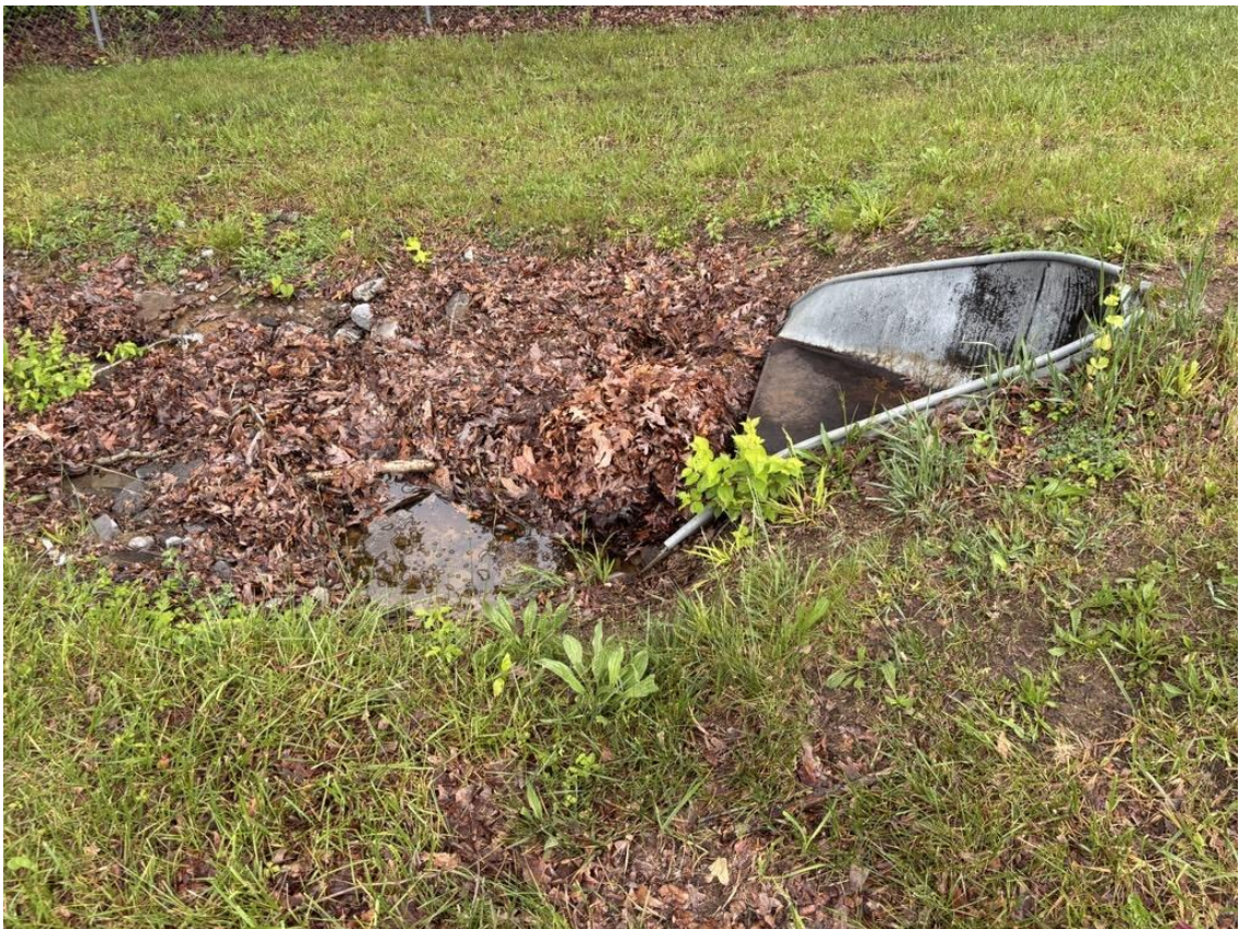
Eroded riprap.
