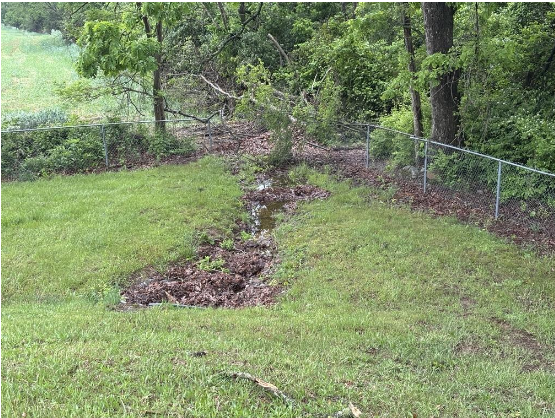
Eroded riprap.
