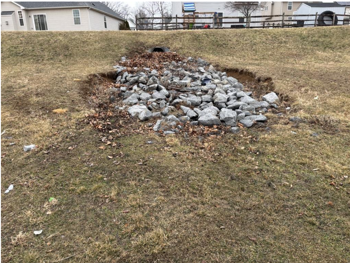
Eroded riprap.
