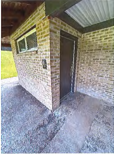
Women's Toilet Room Entrance
