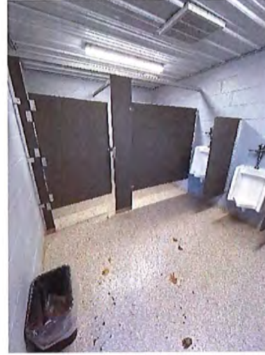
Men's Toilet Room Interior
