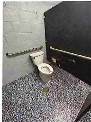
Pavilion #3 Women's Toilet Room Accessible Water Closet / Stall
