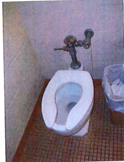
Women's Toilet Room Water Closet
