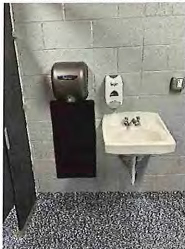
Pavilion #3 Women's Toilet Room Sink
