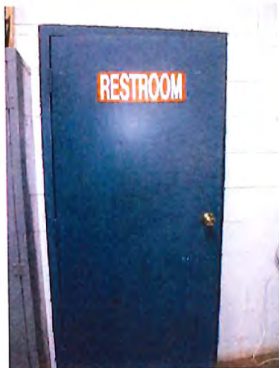
Toilet Room Entrance
