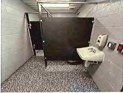
Pavilion #2 Women's Toilet Room Interior
