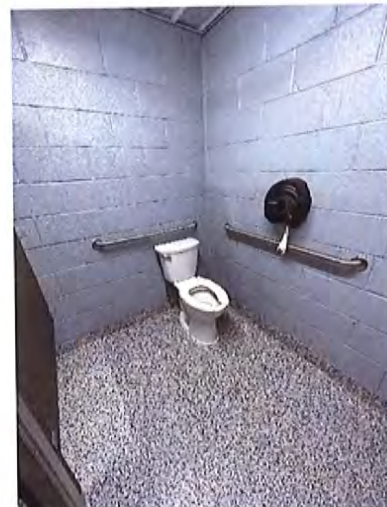
Men's Toilet Room Accessible
