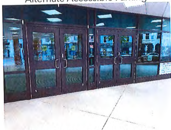
Main Entrance (From Street)
