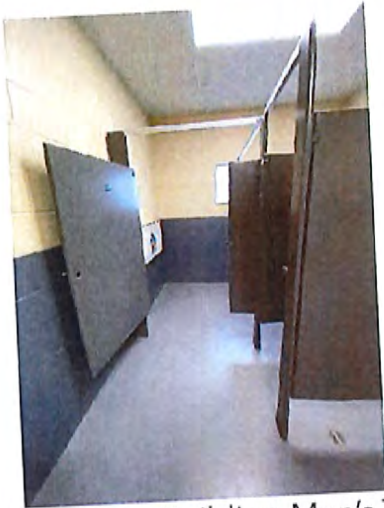
Multi-Purpose Building Men's Toilet Room Interior
