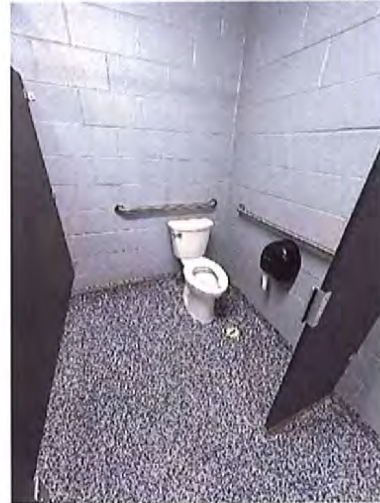
Lower Pavilion - Men's Toilet Room Accessible Water Closet / Stall
