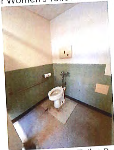
3rd Floor Women's Toilet Room Accessible Water Closet / Stall
