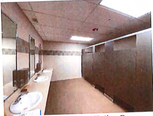
1st Floor Women's Toilet Room
