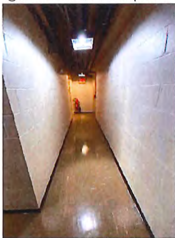
Basement Entrance Route
