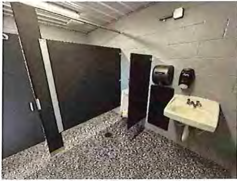
Little League Right Toilet Room Interior
