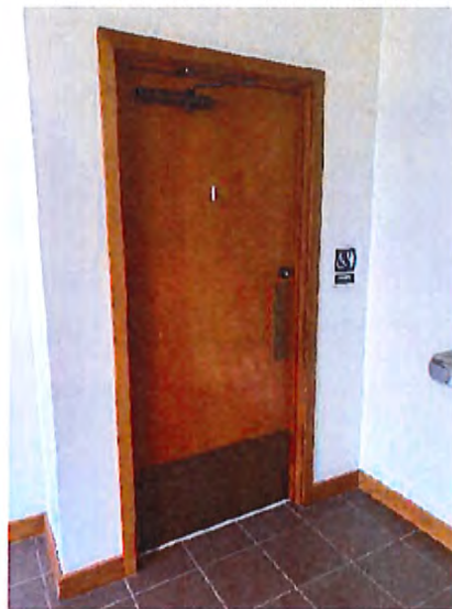
Women's Toilet Room Entrance
