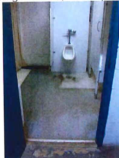
Toilet Room Interior
