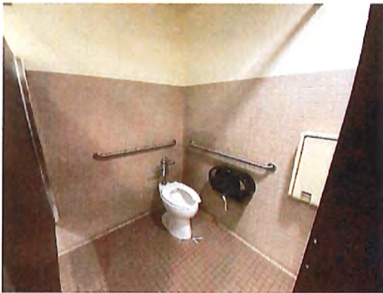
Men's Toilet Room Accessible Water Closet / Stall
