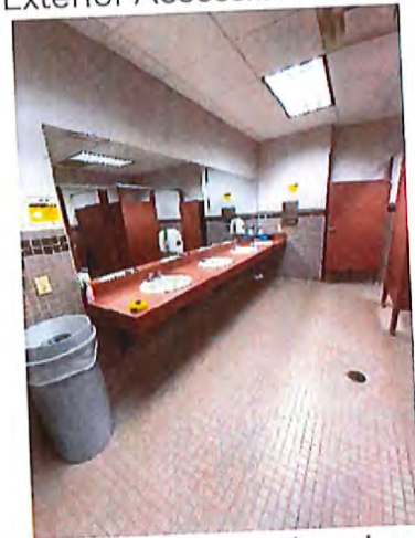
Women's Toilet Room Interior / Sinks
