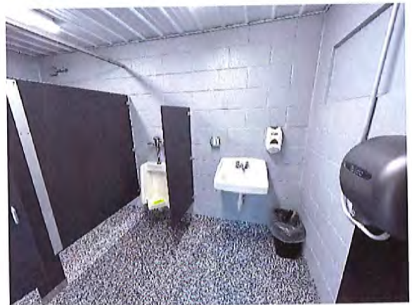
Southern Pavilion Left/North Toilet Room Interior
