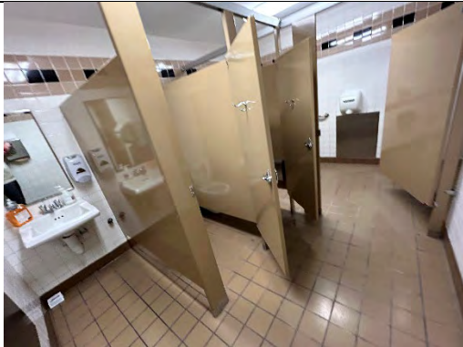
Rear Women's Toilet Room Interior
