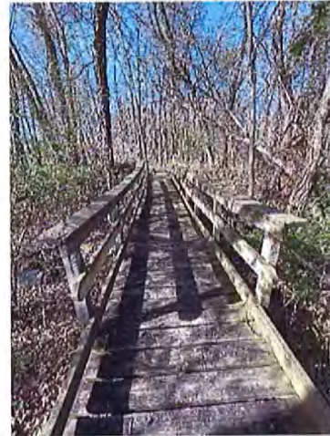
Elevated Walkway with Handrails
