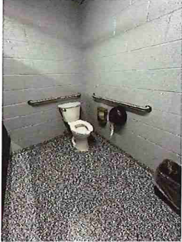
Little League Left Toilet Room Accessible Water Closet / Stall
