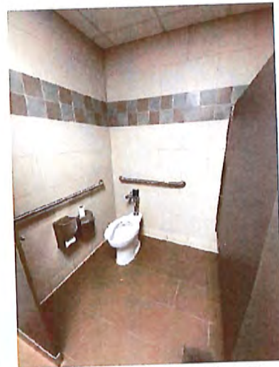
1st Floor Women's Toilet Room Accessible Stall
