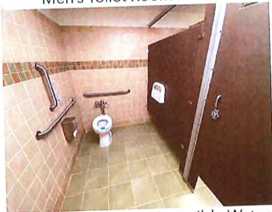
Men's Toilet Room Accessible Water Closet / Stall
