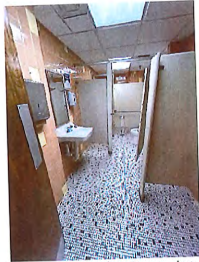
3rd Floor Men's Toilet Room Interior / Sink
