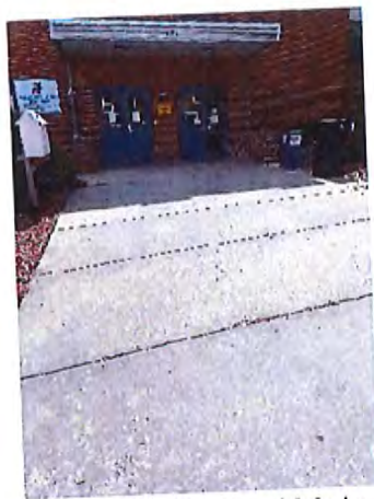
Exterior Entrance Route / Main Entrance
