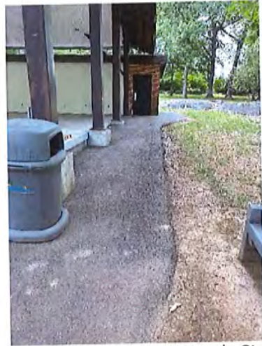
Arts Pavilion Ramp (North Side)
