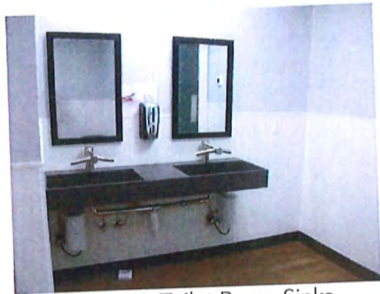
Women's Toilet Room Sinks
