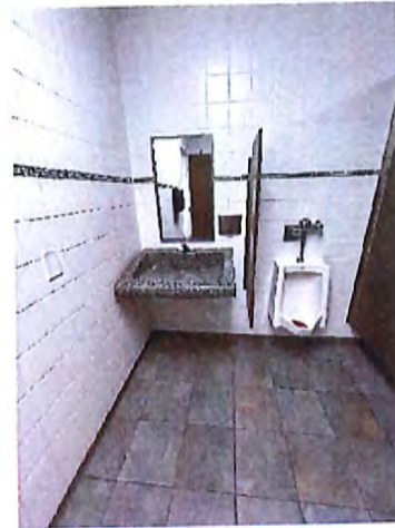
1st Floor Men's Toilet Room Sink
