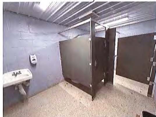
Women's Toilet Room Interior
