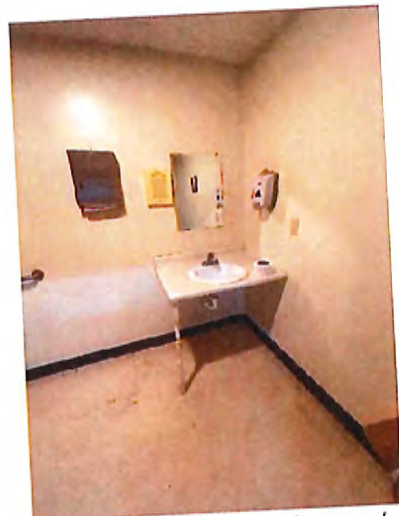
Kennel Club Building Women's Toilet Room Sinks
