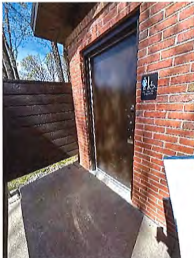
Women's Toilet Room Entrance
