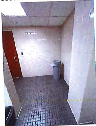
1st Floor Men's Toilet Room Interior Access Route
