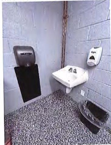
Arts Pavilion Men's Toilet Room Sink
