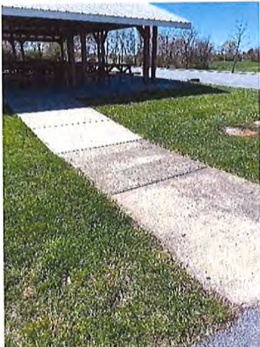
Exterior Accessible Route to Toilet Rooms
