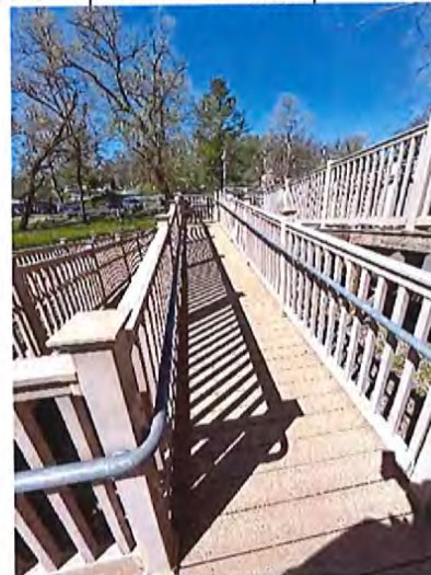
Middle Portion of Ramp to Bridge
