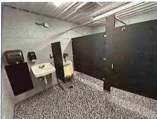
Little League Left Toilet Room Interior
