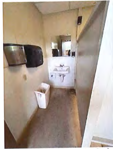
Women's Toilet Room Sink
