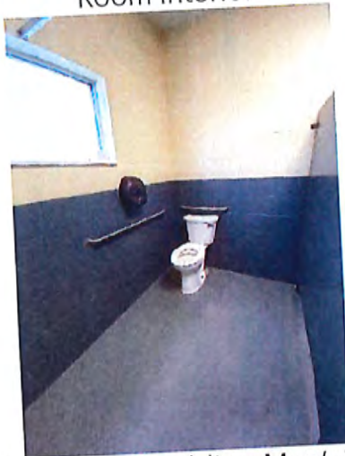
Multi-Purpose Building Men's Toilet Room Accessible Water Closet / Stall
