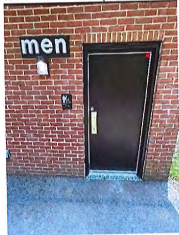
Arts Pavilion Men's Toilet Room Entrance
