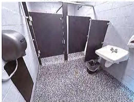
Northern Pavilion Left/East Toilet Room Interior
