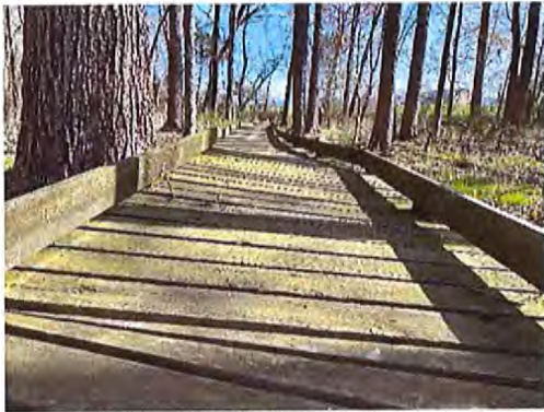
Elevated Walkway Surface
