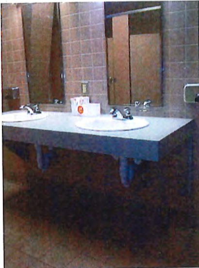
Women's Toilet Room Sinks
