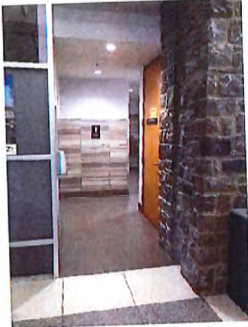
Women's Toilet Room Entrance
