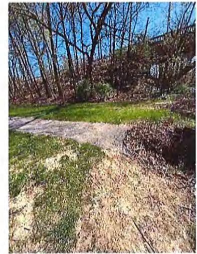
Exterior Accessible Route Endpoint (To Water)
