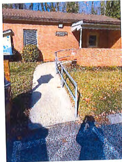
(Right) Ramp to Main Entrance
