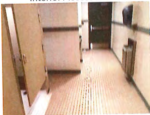
Men's Toilet Room Interior
