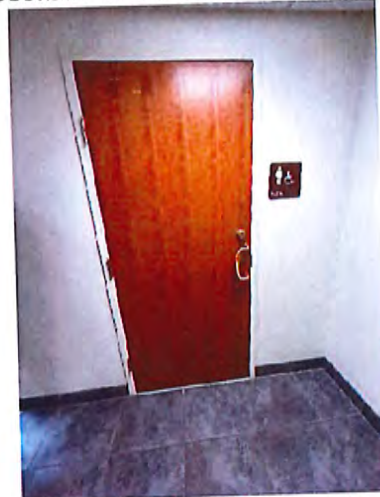
2 nd Floor Men's Toilet Room Entrance
