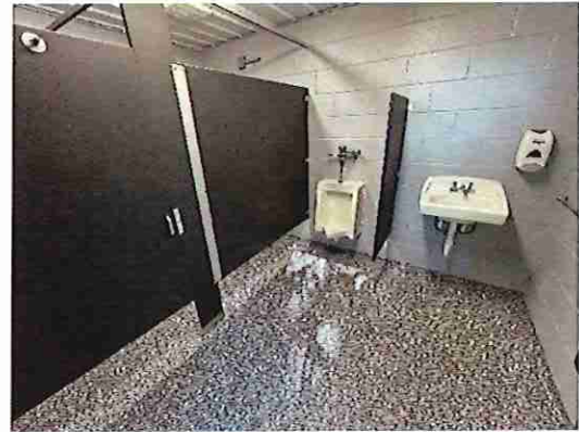
Tennis Court Right Toilet Room Interior
