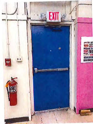
Main Entrance Interior
