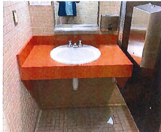
Men's Toilet Room Sink
