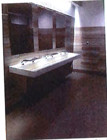
Women's Toilet Room Sinks
