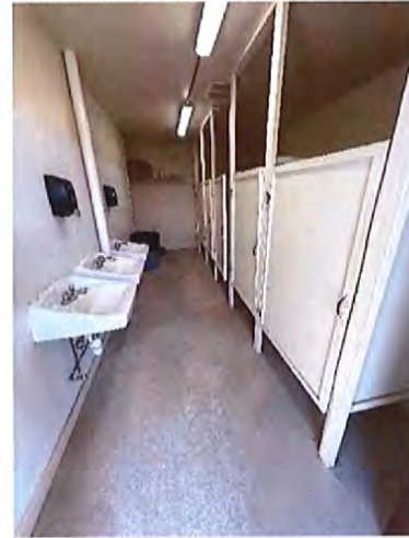
Women's Toilet Room Interior
