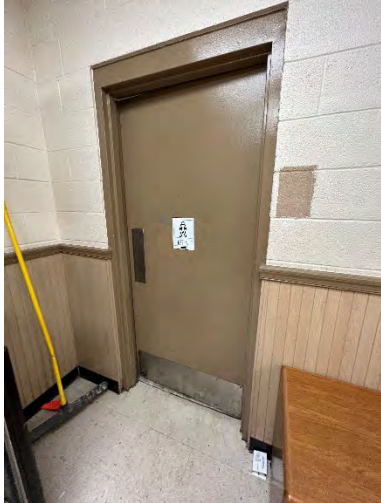
Rear Men's Toilet Room Entrance
