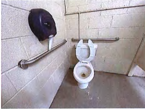
Women's Toilet Room Accessible Water Closet
