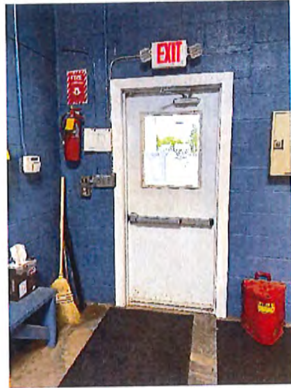
Main Entrance Interior
