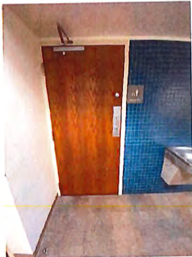
3rd Floor Women's Toilet Room Entrance
