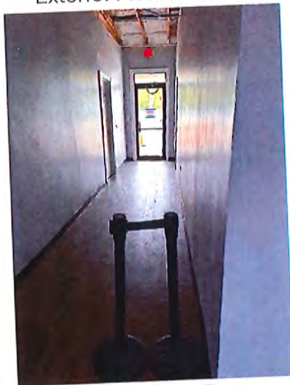
Interior Access Route
