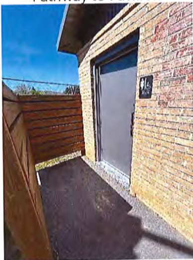
Women's Toilet Room Entrance
