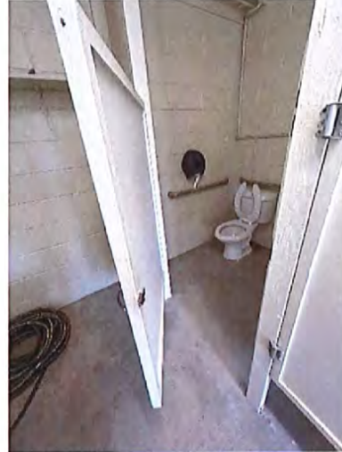
Women's Toilet Room Accessible Stall
