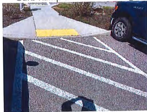
Curb Ramp at Access Aisle
