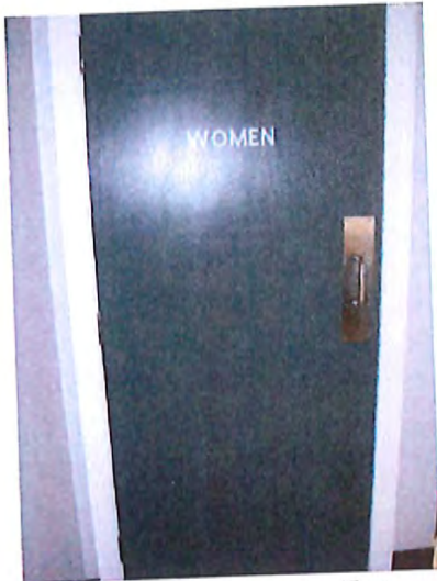
Women's Toilet Room Entrance
