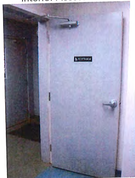
Toilet Room Entrance
