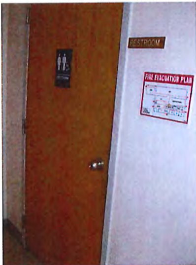
Toilet Room Entrance
