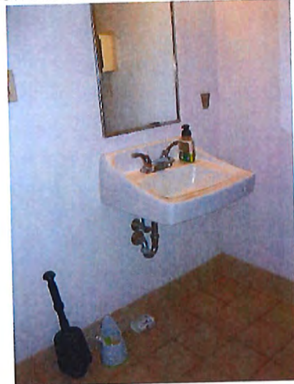
Men's Toilet Room Sink
