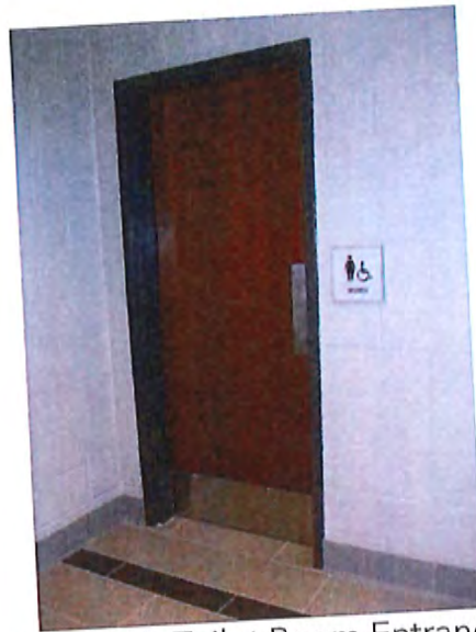
Women's Toilet Room Entrance
