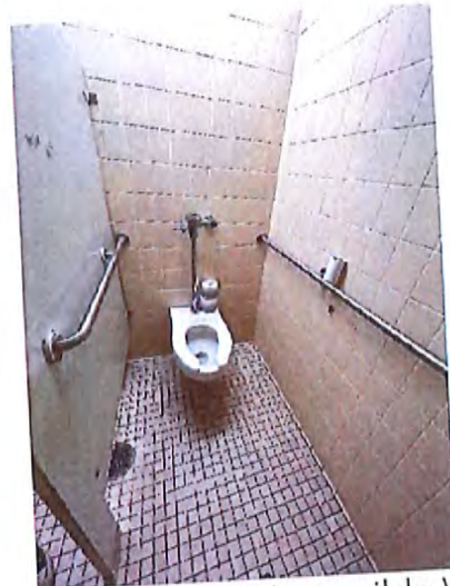
Men's Toilet Room Accessible Water Closet / Stall
