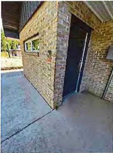
Pavilion #3 Women's Toilet Room Entrance
