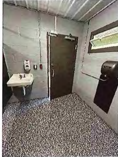
Pavilion #2 Women's Toilet Room Sink
