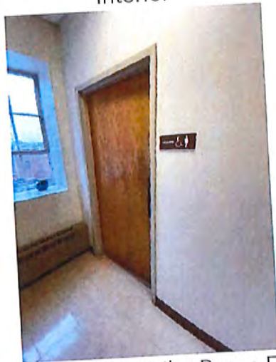
3rd Floor Women's Toilet Room Entrance
