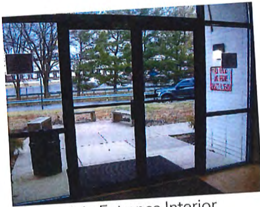
Main Entrance Interior
