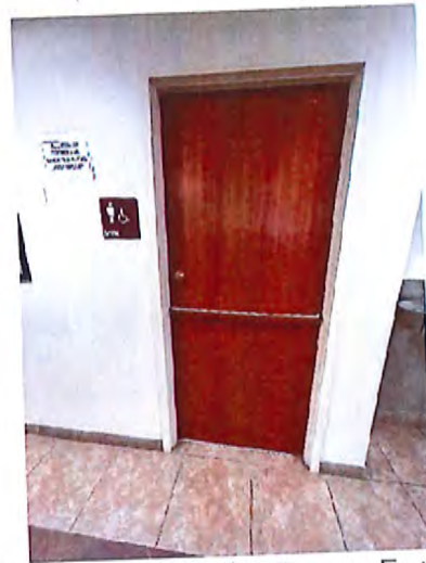
1st Floor Men's Toilet Room Entrance
