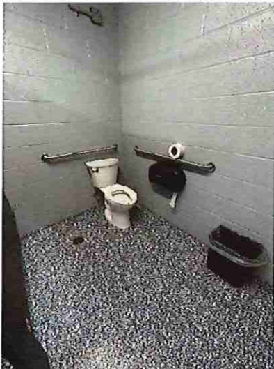
Pavilion #2 Men's Toilet Room Accessible Water Closet / Stall
