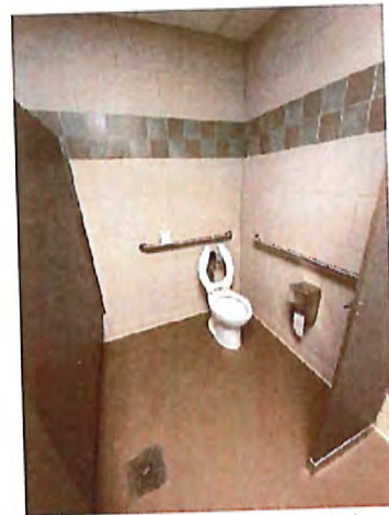
1 st Floor Men's Toilet Room Accessible Stall
