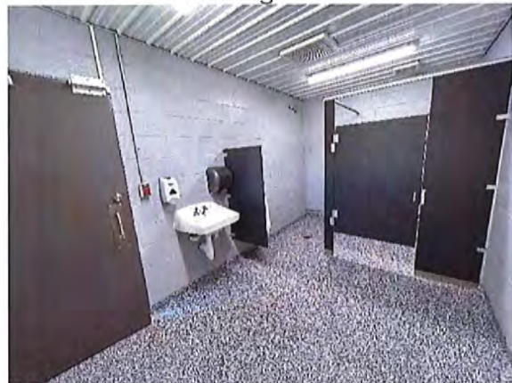
Lower Pavilion - Men's Toilet Room Interior
