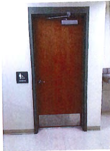
Women's Toilet Room Entrance
