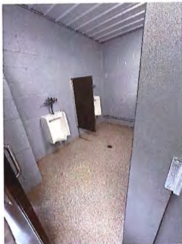
Pavilion Men's Toilet Room Interior
