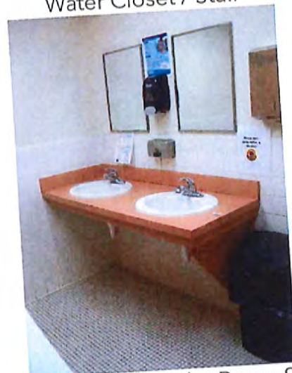
(Left) Women's Toilet Room Sink
