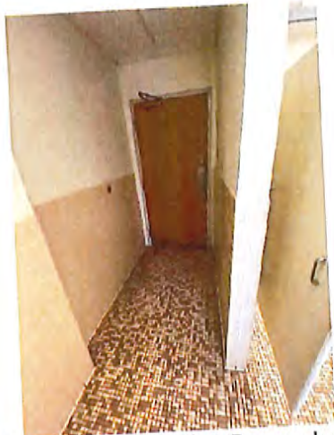
3rd Floor Men's Toilet Room Interior Entrance
