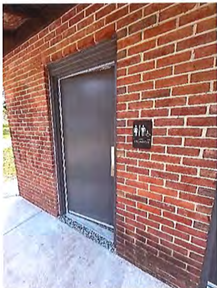
Northern Pavilion Left/East Toilet Room Entrance
