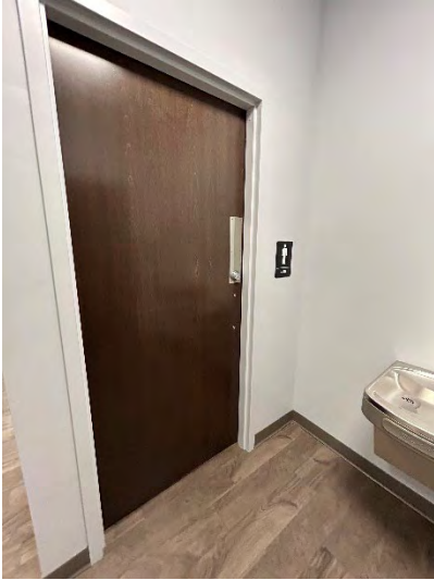
Front Men's Toilet Room Entrance
