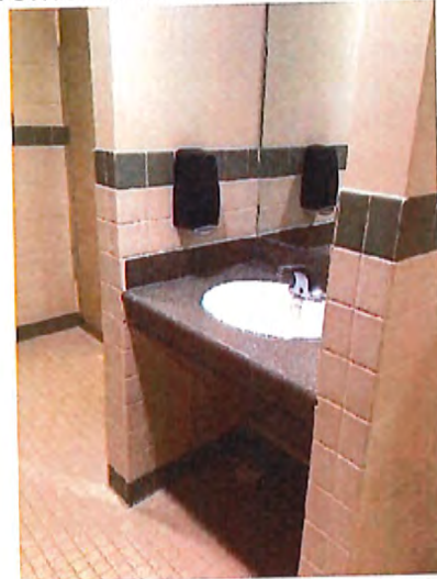
Women's Toilet Room Sink
