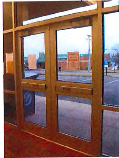
Main Entrance Interior
