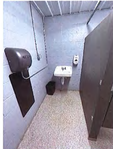
Women's Toilet Room Sink
