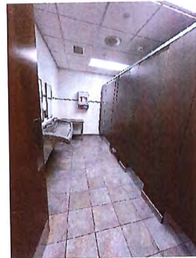
2nd Floor Women's Toilet Room Interior
