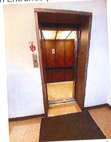
Elevator Entrance / Interior
