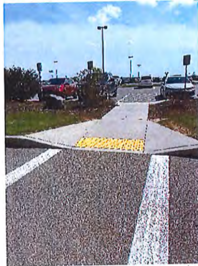
Curb Ramp at Road Crossing
