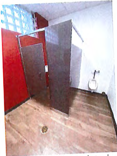
Men's Toilet Room Interior
