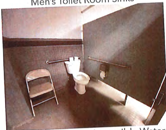
Men's Toilet Room Accessible Water Closet / Stall
