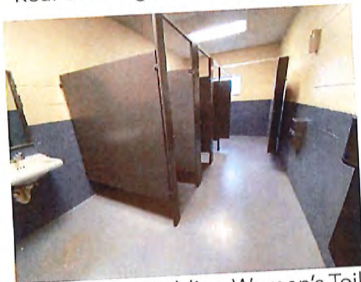
Multi-Purpose Building Women's Toilet Room Interior
