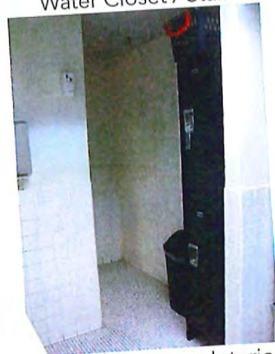
(Right) Men's Toilet Room Interior Access Route
