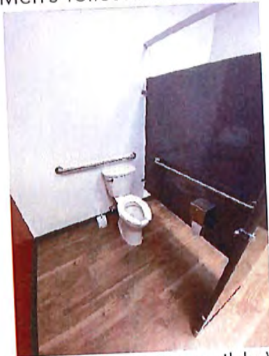
Men's Toilet Room Accessible Water Closet / Stall
