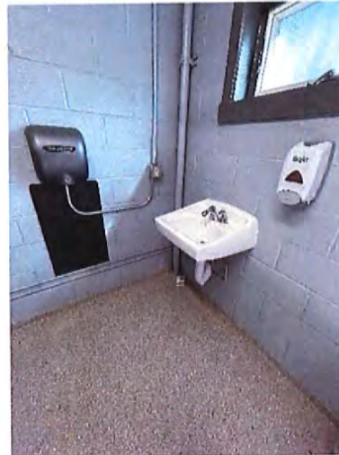
Pavilion Men's Toilet Room Sink
