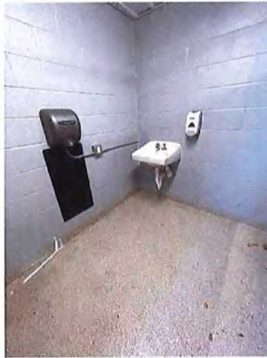
Women's Toilet Room Sink
