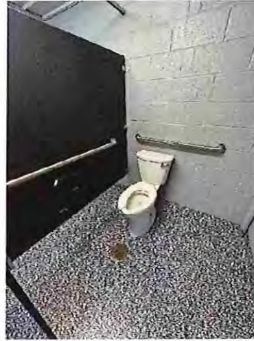
Pavilion #3 Men's Toilet Room Accessible Water Closet / Stall
