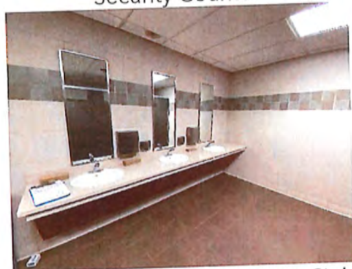
1st Floor Women's Toilet Room Sinks
