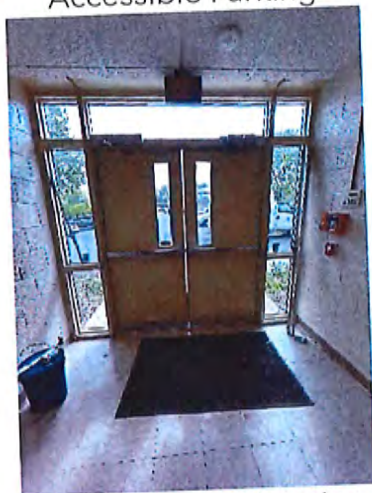
Main Entrance Interior
