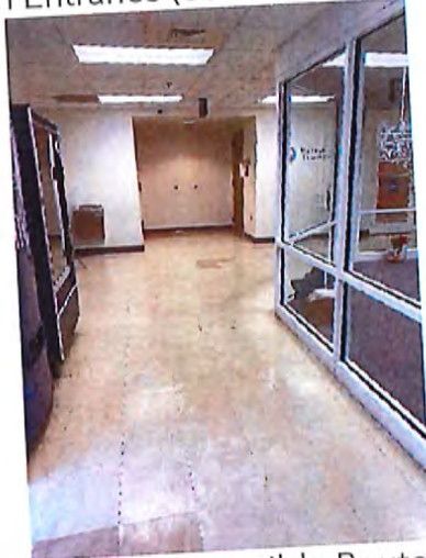
Interior Accessible Route
