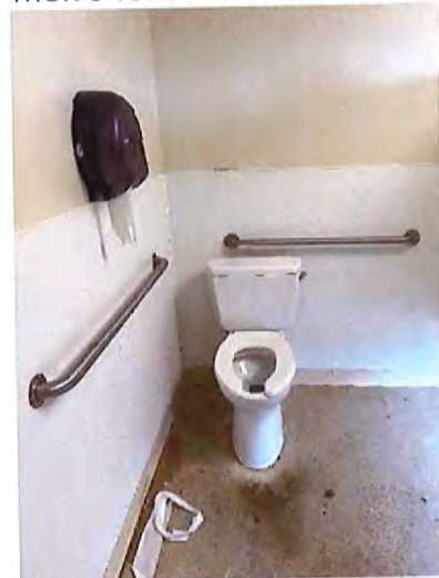
Men's Toilet Room Accessible Water Closet / Stall
