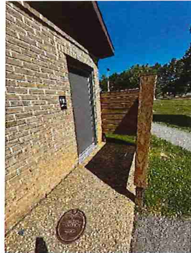
Little League Right Toilet Room Entrance
