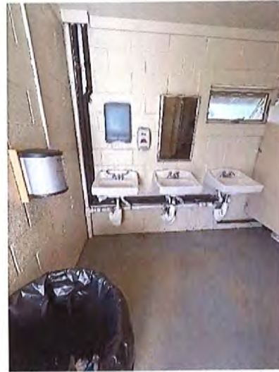
Women's Toilet Room Sinks
