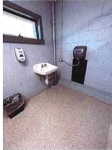
Pavilion Women's Toilet Room Sink
