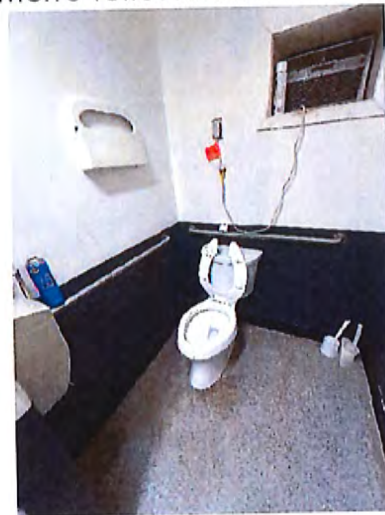
Men's Toilet Room Accessible Water Closet / Stall
