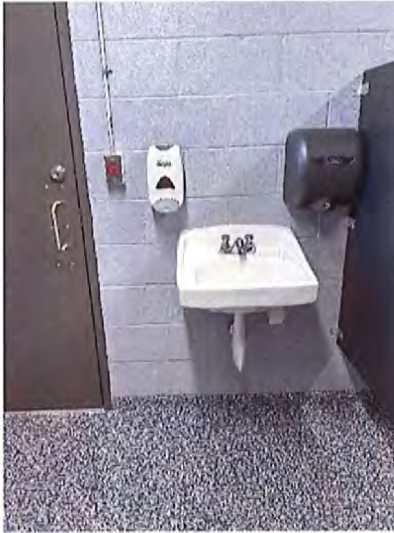
Lower Pavilion - Men's Toilet Room Sink
