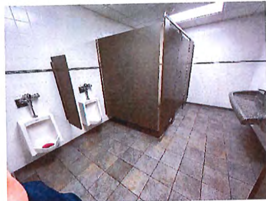
2 nd Floor Men's Toilet Room Interior
