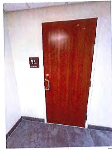
2 nd Floor Women's Toilet Room Entrance
