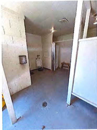
Men's Toilet Room Interior
