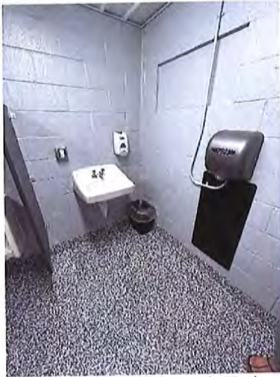
Southern Pavilion Left/North Toilet Room Sink
