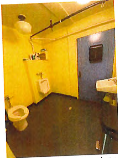
Single-Use Toilet Room Interior
