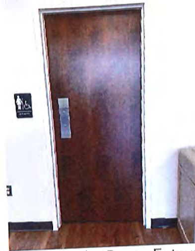
Women's Toilet Room Entrance
