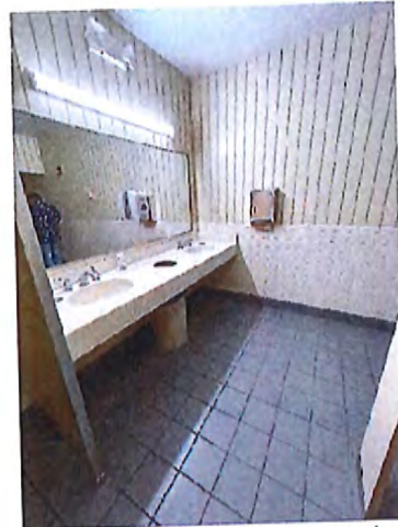
Men's Toilet Room Sinks
