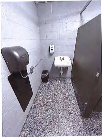
Women's Toilet Room Sink
