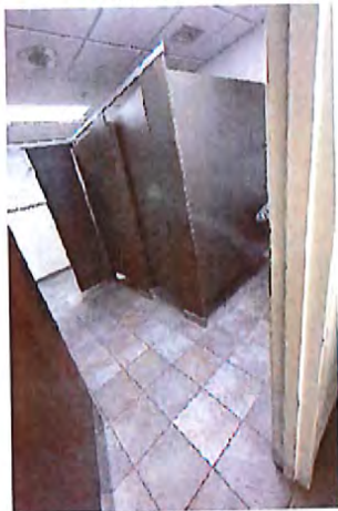
1st Floor Women's Toilet Room Interior
