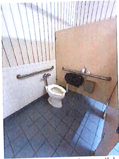
Women's Toilet Room Accessible Stall
