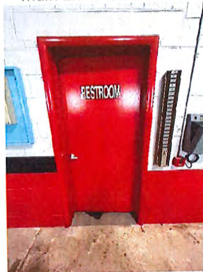
Toilet Room Entrance
