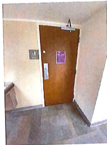
2 nd Floor Men's Toilet Room Entrance
