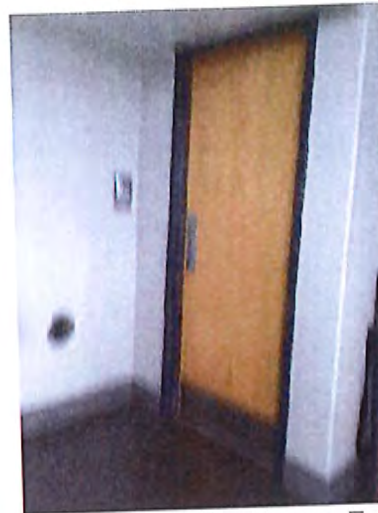
Terminal Men's Toilet Room Entrance
