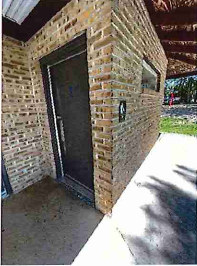
Pavilion #4 Men's Toilet Room Entrance
