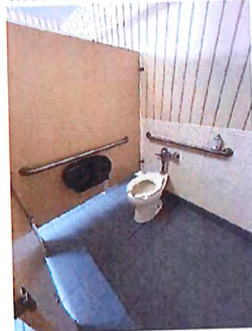
Men's Toilet Room Accessible Stall
