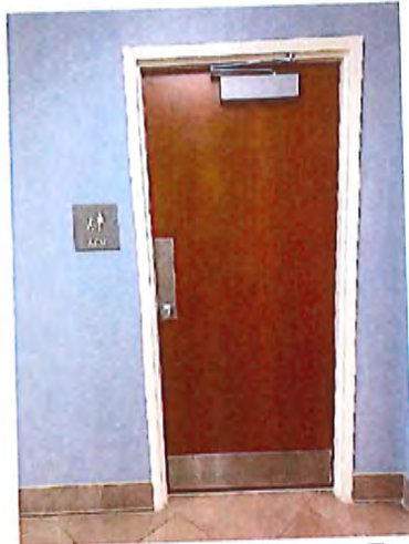
1 st Floor Men's Toilet Room Entrance
