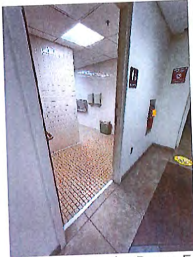
1st Floor Women's Toilet Room Entrance Route
