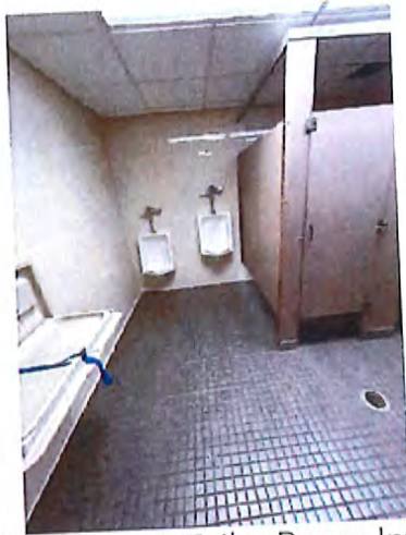
1st Floor Men's Toilet Room Interior
