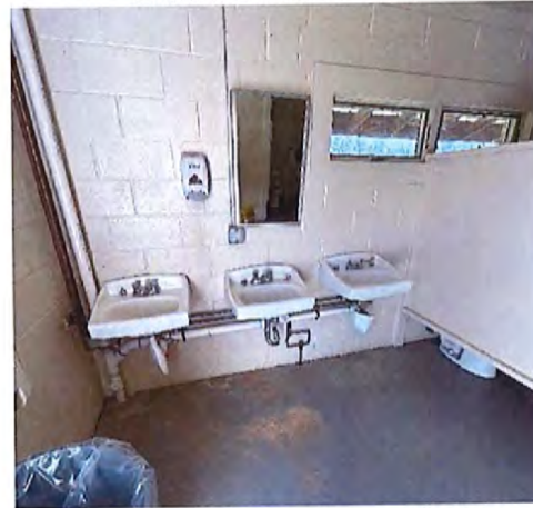
Women's Toilet Room Sinks
