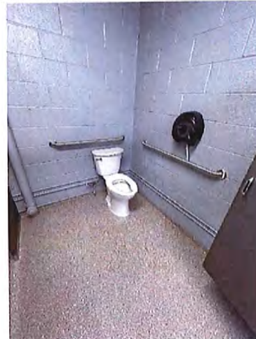
Pavilion Men's Toilet Room Accessible Water Closet / Stall
