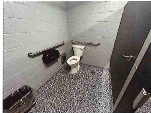
Tennis Court Right Toilet Room Accessible Water Closet / Stall
