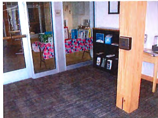
Interior Entrance Automatic Door Control
