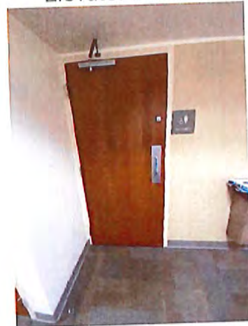
2nd Floor Women's Toilet Room Entrance
