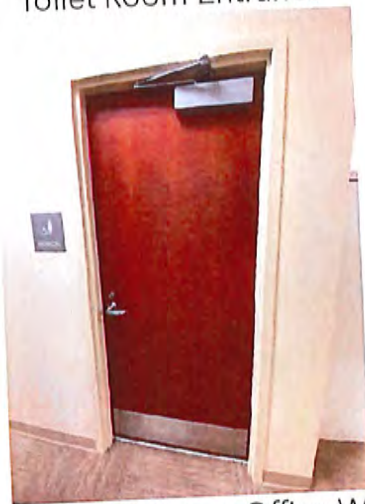
County Commissioner Office Women's Toilet Room Entrance
