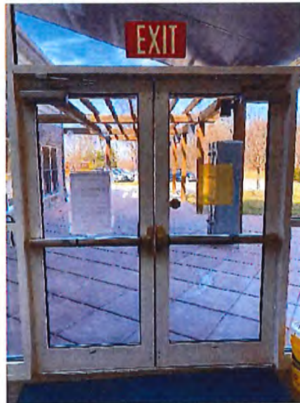
Main Entrance Interior
