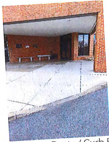
Main Entrance Route / Curb Ramp
