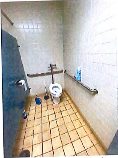
Men's Toilet / Locker Room Accessible Water Closet / Stall
