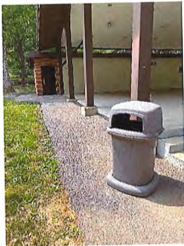
Arts Pavilion Ramp (South Side)
