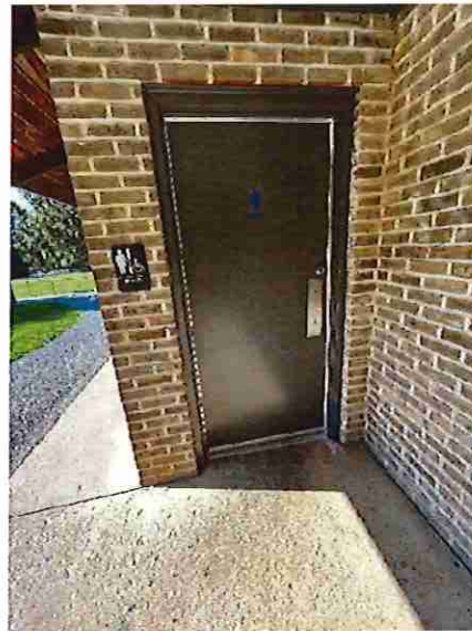
Pavilion #2 Women's Toilet Room Entrance
