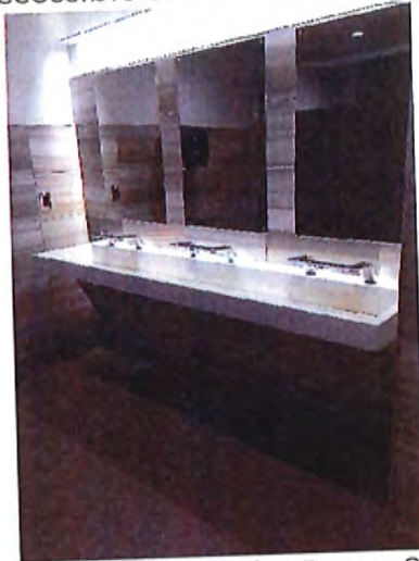
Terminal Men's Toilet Room Sinks
