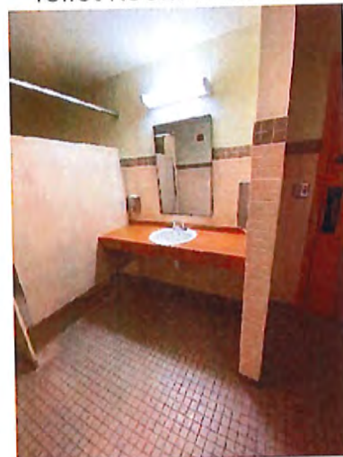
Women's Toilet Room Sink
