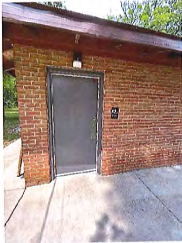
Southern Pavilion Right/South Toilet Room
