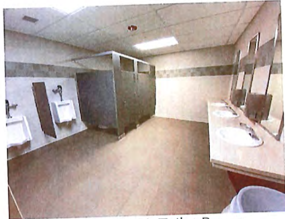
1 st Floor Men's Toilet Room
