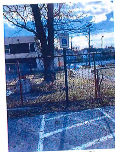
Accessible Parking Signage
