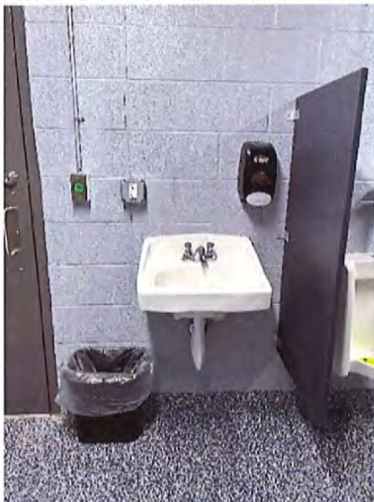
Men's Toilet Room Interior
