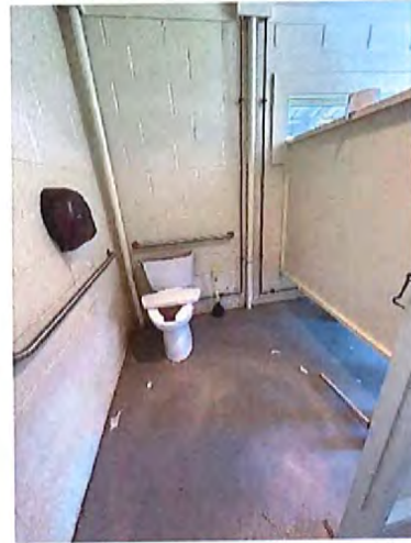
Men's Toilet Room Accessible Water Closet / Stall
