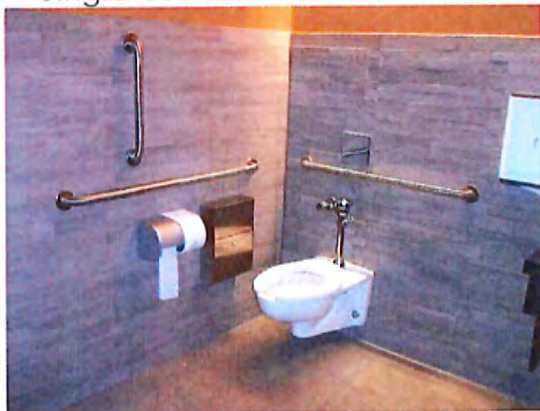
Single-Use Toilet Room Accessible Water Closet
