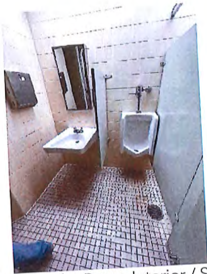
Men's Toilet Room Interior / Sink
