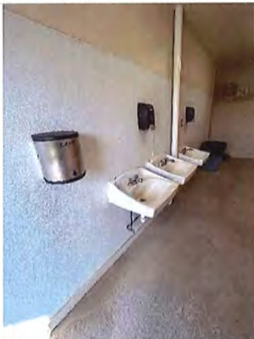
Women's Toilet Room Sinks
