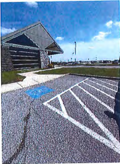
Alternate Accessible Parking Area
