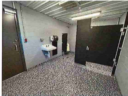
Pavilion #3 Men's Toilet Room Interior
