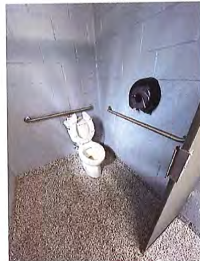
Men's Toilet Room Accessible Water Closet / Stall
