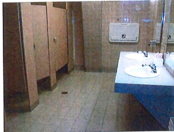
Women's Toilet Room Interior
