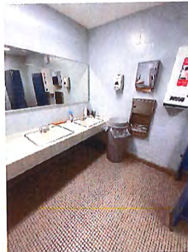
3rd Floor Women's Toilet Room Sinks
