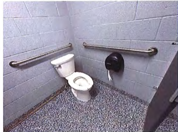
Men's Toilet Room Accessible Water Closet / Stall
