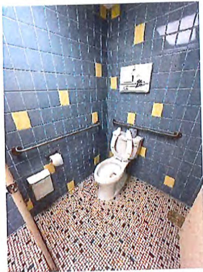
3 rd Floor Women's Toilet Room Accessible Water Closet / Stall
