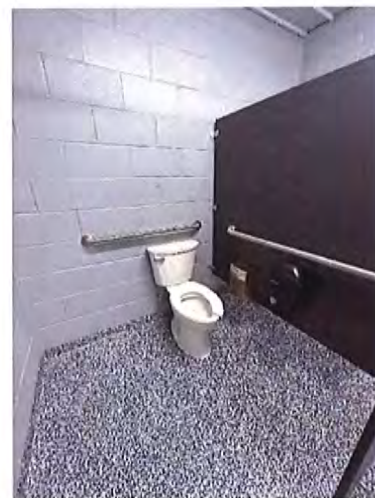
Lower Pavilion - Women's Toilet Room Accessible Water Closet / Stall
