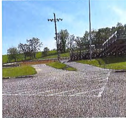
Access Aisle & Exterior Accessible Route
