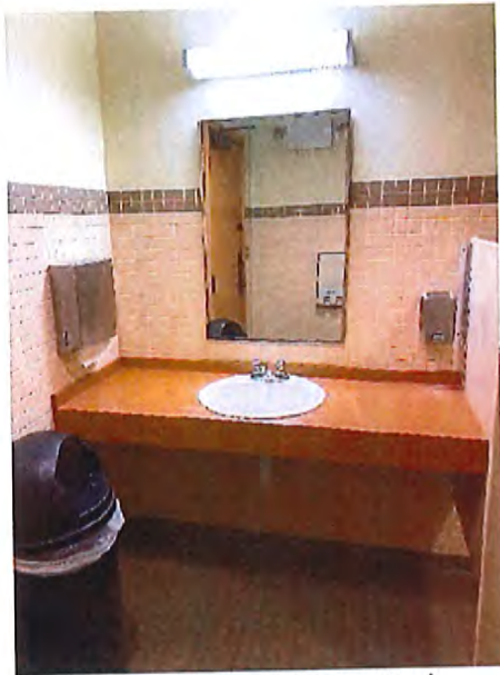
Men's Toilet Room Sink
