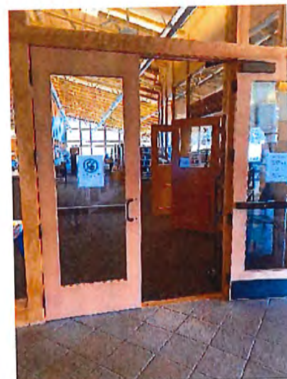
Interior Access Route
