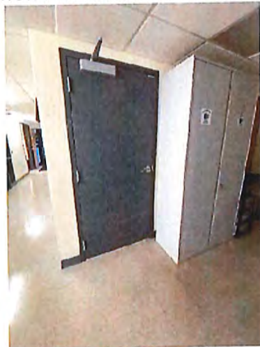
Women's Toilet Room Entrance
