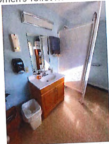
Women's Toilet Room Sink
