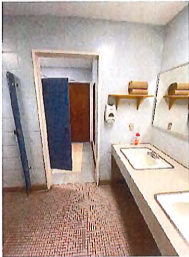
3 rd Floor Women's Toilet Room Interior
