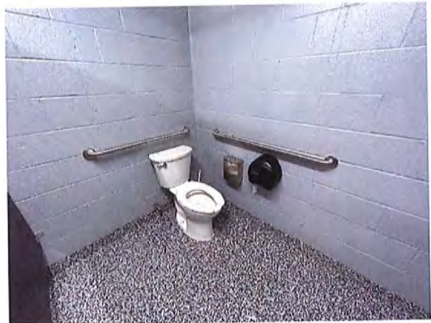
Southern Pavilion Right/South Toilet Room Accessible Water Closet / Stall
