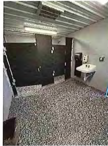
Pavilion #3 Women's Toilet Room Interior
