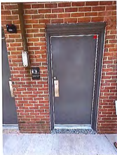
Northern Pavilion Right/West Toilet Room Entrance
