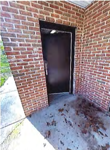
Pavilion Women's Toilet Room Entrance
