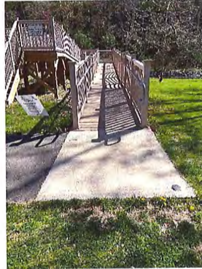
Bottom portion of Ramp to Bridge
