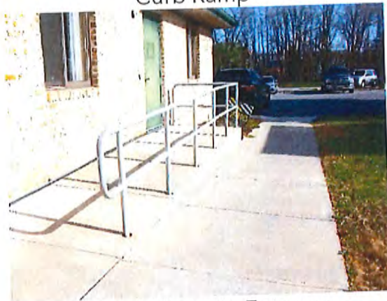
Ramp / Alternate Entrance
