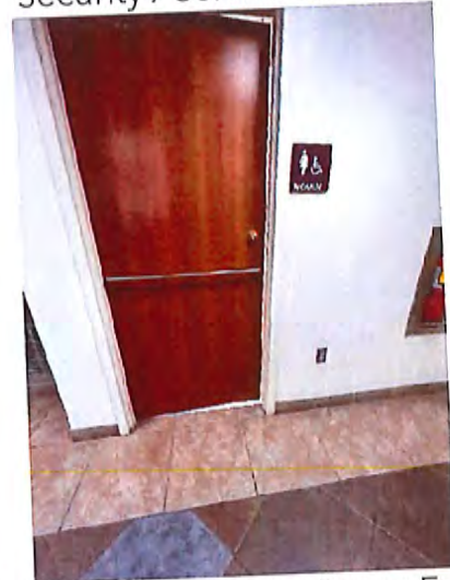
1st Floor Women's Toilet Room Entrance
