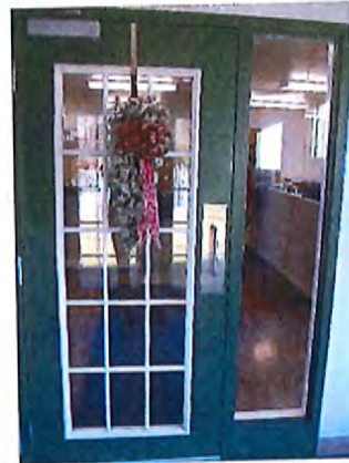
Main Entrance - Interior Door
