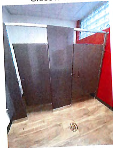
Women's Toilet Room Interior
