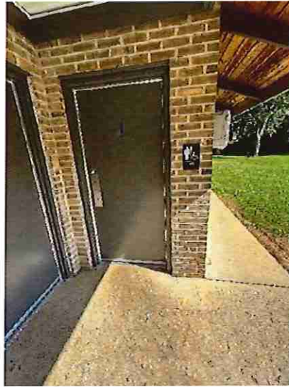
Pavilion #2 Men's Toilet Room Entrance
