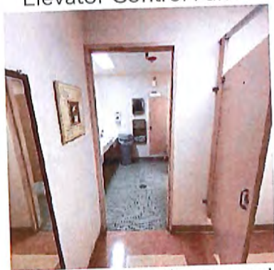
2nd Floor Women's Toilet Room Interior
