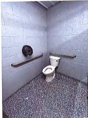
Men's Toilet Room Accessible Water Closet / Stall
