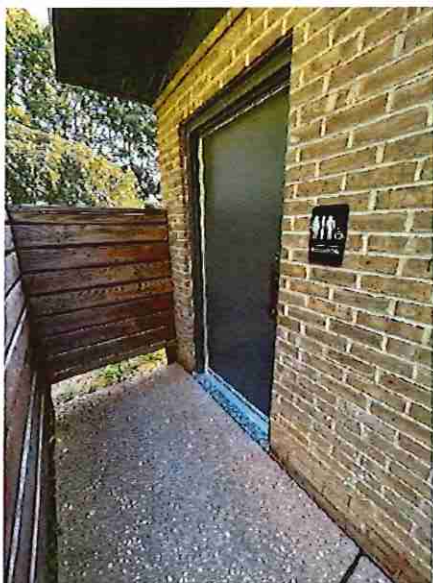
Tennis Court Left Toilet Room Entrance
