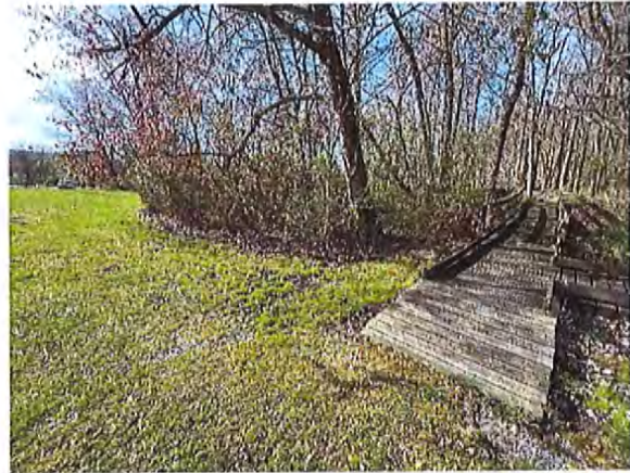
Exterior Access Route / Entrance to Elevated Walkway
