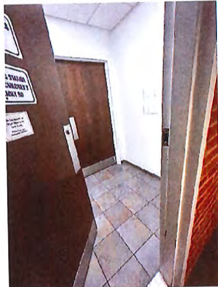
1st Floor Men's Toilet Room Entrance
