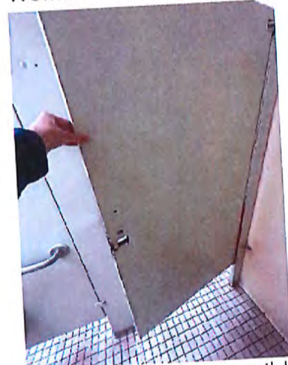
Women's Toilet Room Accessible Stall Door
