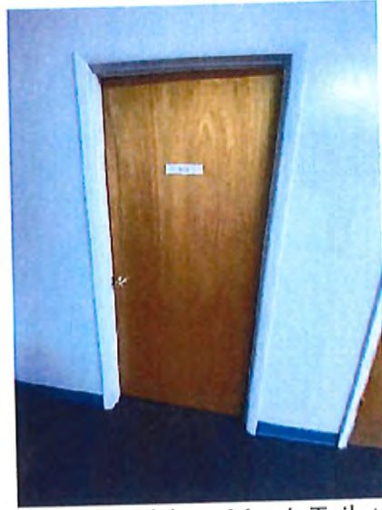
Kennel Club Building Men's Toilet Room Entrance
