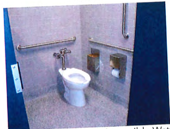
Women's Locker Room Accessible Water Closet / Stall
