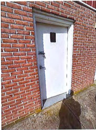
Women's Toilet Room Entrance
