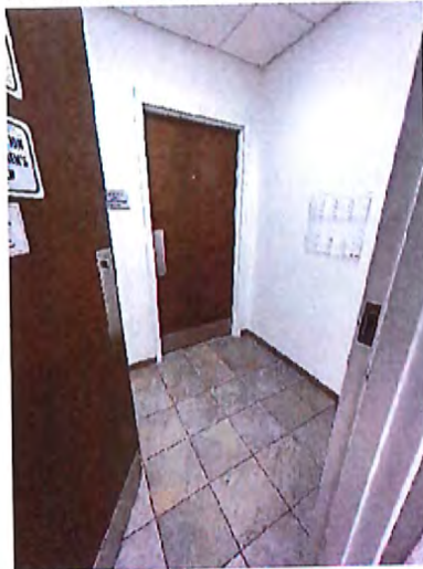
2 nd Floor Men's Toilet Room Entrance
