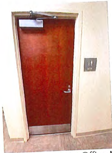
County Commissioner Office Men's Toilet Room Entrance
