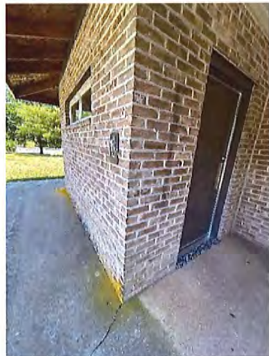
Upper Pavilion - Women's Toilet Room Entrance
