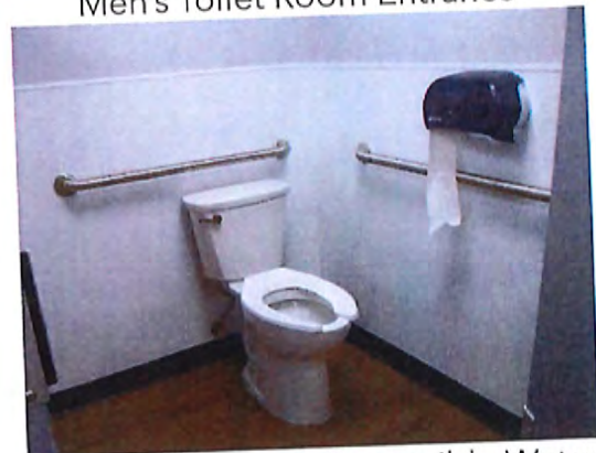
Men's Toilet Room Accessible Water Closet / Stall
