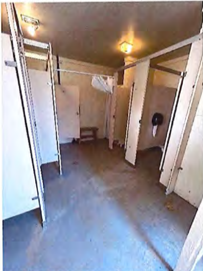
Women's Toilet Room Interior
