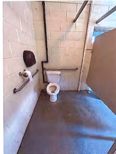
Men's Toilet Room Accessible Water Closet / Stall
