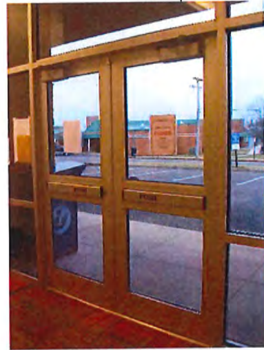
Main Entrance Interior
