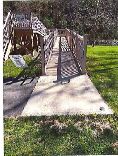
Bottom portion of Ramp to Bridge
