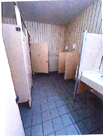
Men's Toilet Room
