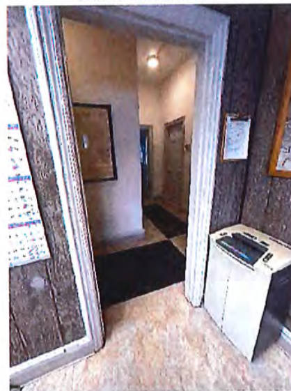
Interior Access Route
