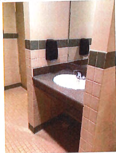
Women's Toilet Room Sink
