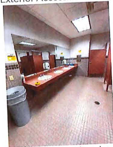
Women's Toilet Room Interior / Sinks
