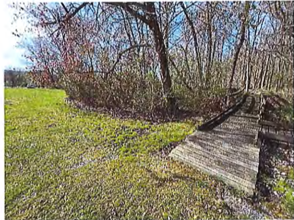
Exterior Access Route / Entrance to Elevated Walkway
