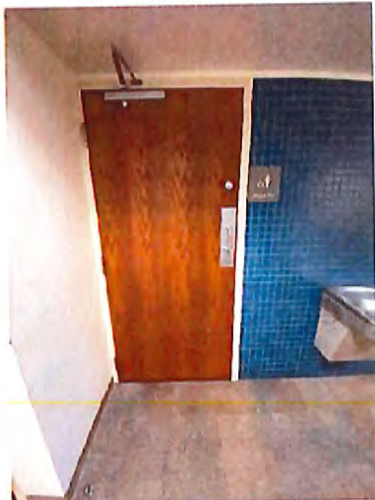
3rd Floor Women's Toilet Room Entrance
