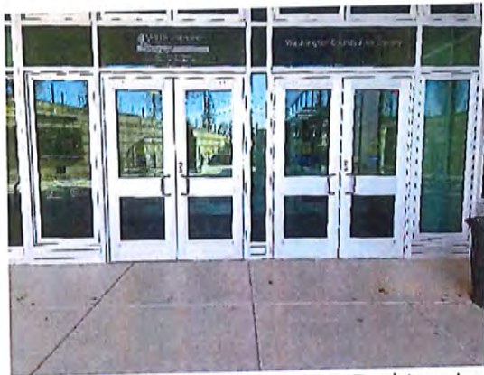
Alternative Entrance (From Parking Lot)
