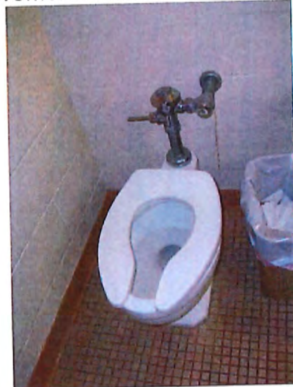
Women's Toilet Room Water Closet
