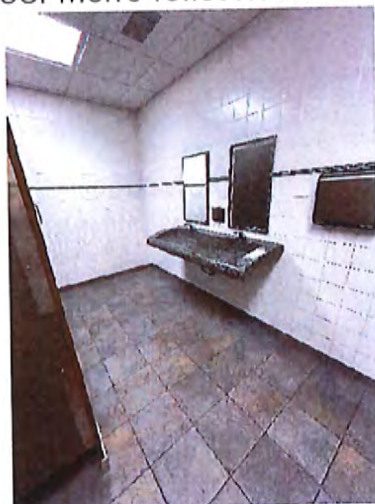
2 nd Floor Men's Toilet Room Sink
