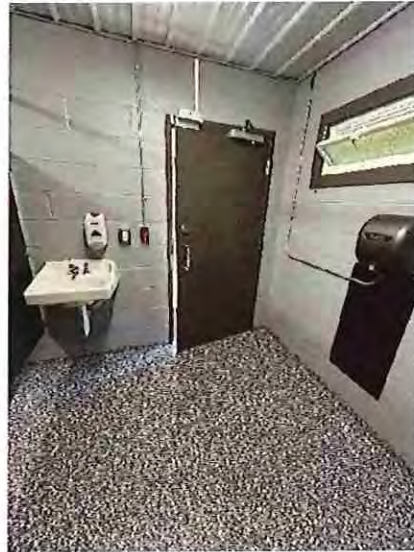
Pavilion #2 Women's Toilet Room Sink
