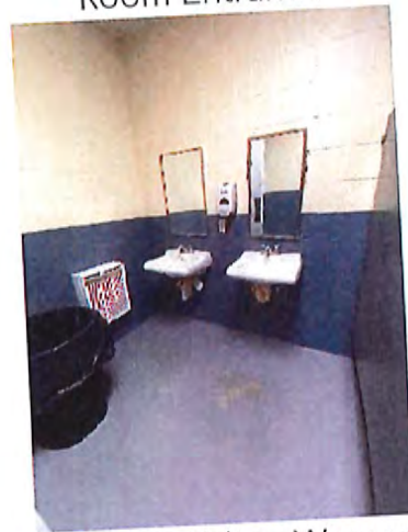
Multi-Purpose Building Women's Toilet Room Sinks
