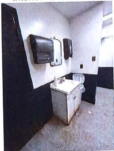
Men's Toilet Room Sink
