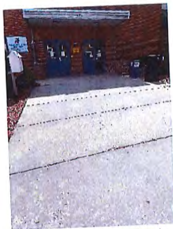
Exterior Entrance Route / Main Entrance
