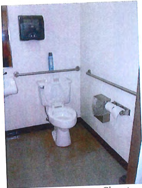
Toilet Room Water Closet
