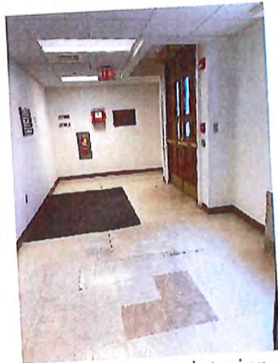
Main Entrance Interior
