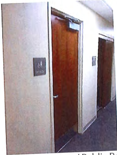
Business Development / Public Relations Women's Toilet Room Entrance
