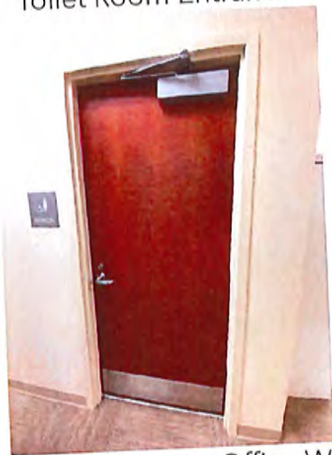
County Commissioner Office Women's Toilet Room Entrance
