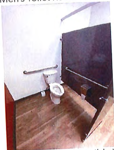
Men's Toilet Room Accessible Water Closet / Stall
