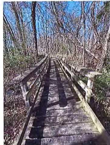
Elevated Walkway with Handrails
