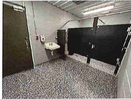
Pavilion #4 Men's Toilet Room Interior
