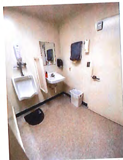
Men's Toilet Room Interior / Sinks
