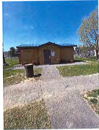
Pathway to Toilet Rooms
