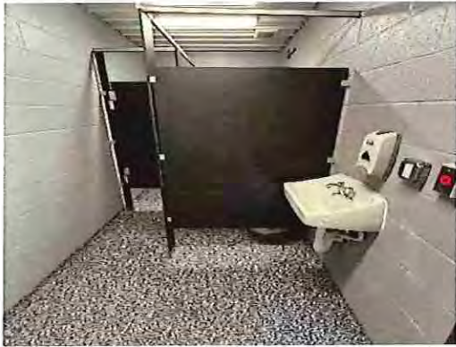
Pavilion #2 Women's Toilet Room Interior
