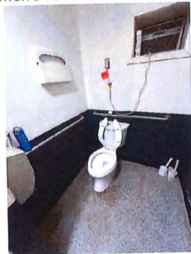
Men's Toilet Room Accessible Water Closet / Stall
