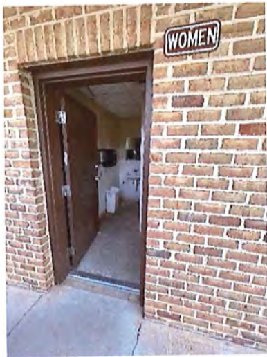
Women's Toilet Room Entrance
