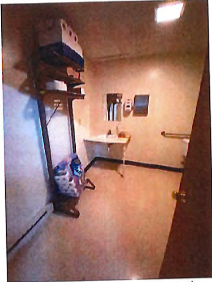
Kennel Club Building Men's Toilet Room Sink / Interior
