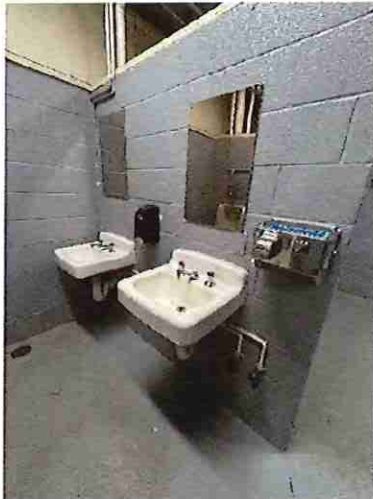
Pool Men's Toilet Room Sinks
