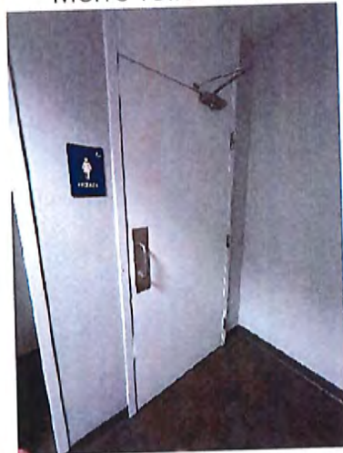
Women's Toilet Room Entrance
