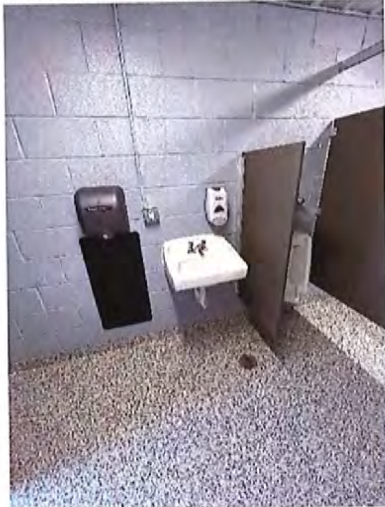
Men's Toilet Room Sink
