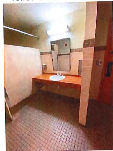
Women's Toilet Room Sink
