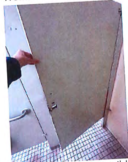
Women's Toilet Room Accessible Stall Door
