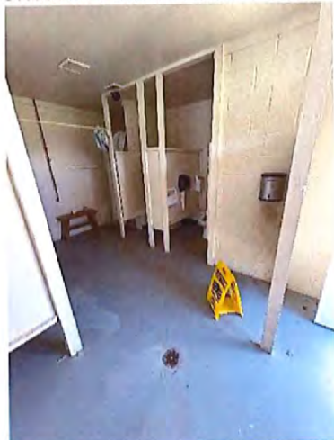
Women's Toilet Room Interior
