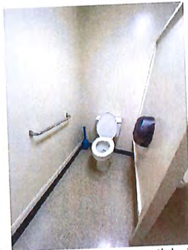
Men's Toilet Room Accessible Water Closet / Stall
