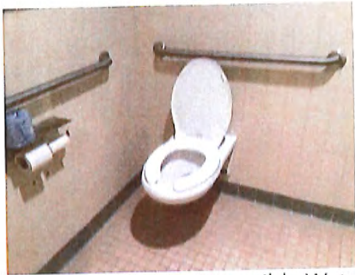
Men's Toilet Room Accessible Water Closet / Stall
