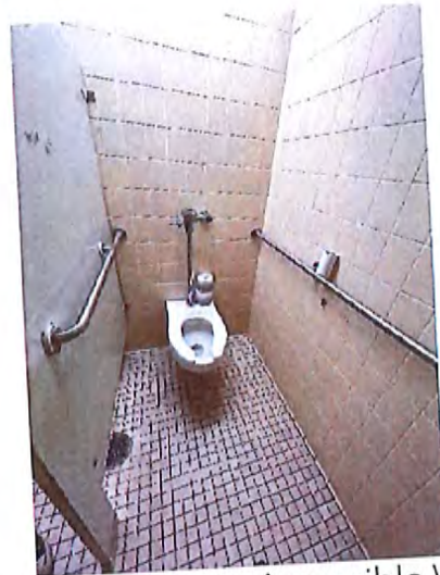
Men's Toilet Room Accessible Water Closet / Stall
