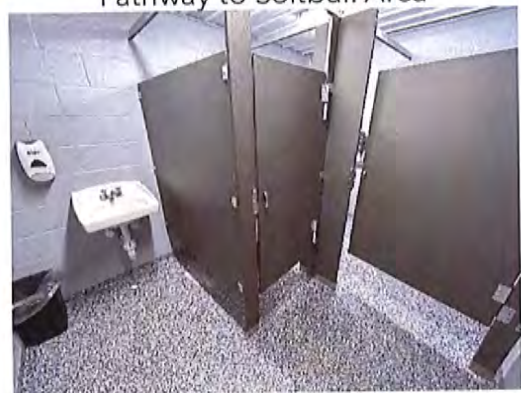
Women's Toilet Room Interior
