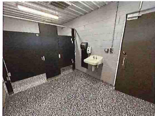
Pavilion #4 Women's Toilet Room Interior
