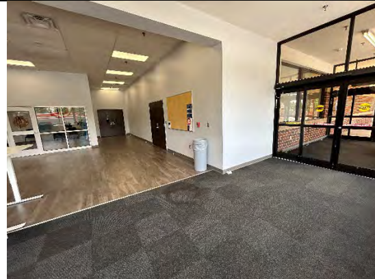
Interior Accessible Route
