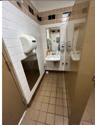
Rear Women's Toilet Room Sink
