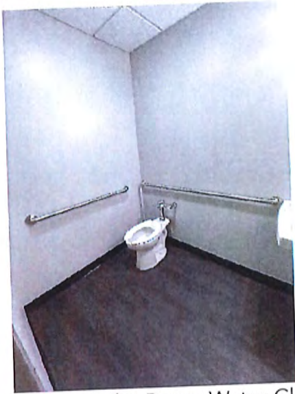
Accessible Toilet Room Water Closet
