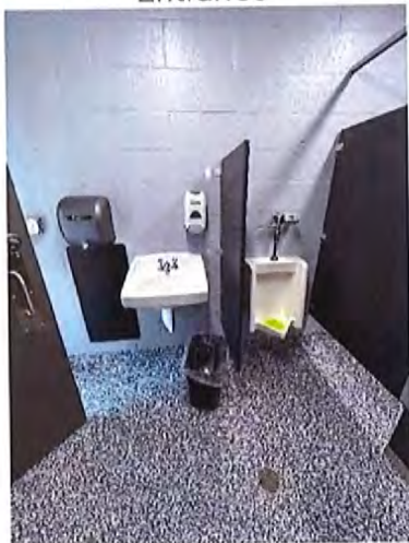
Northern Pavilion Right/West Toilet Room Sink
