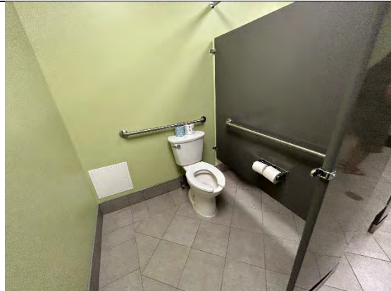
Front Men's Toilet Accessible Stall
