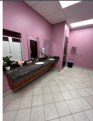
Front Women's Toilet Room Sinks
