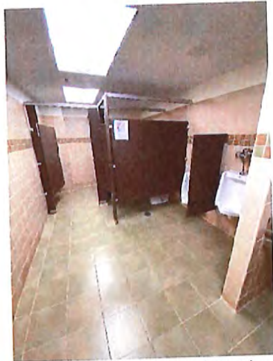
Men's Toilet Room Interior
