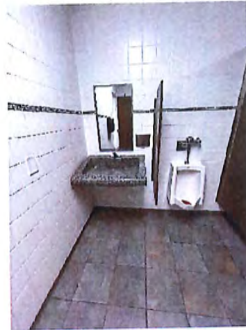
1st Floor Men's Toilet Room Sink
