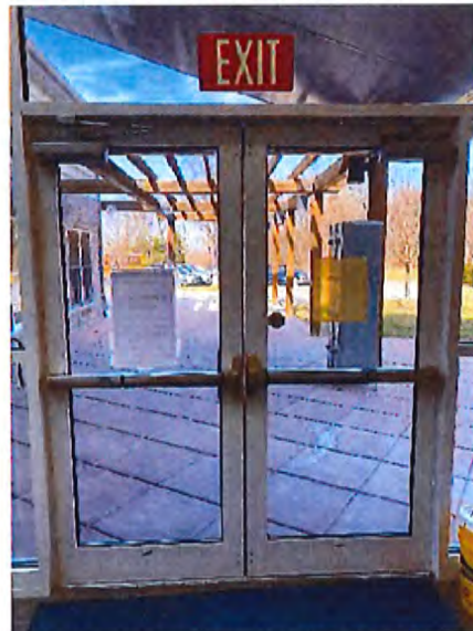
Main Entrance Interior
