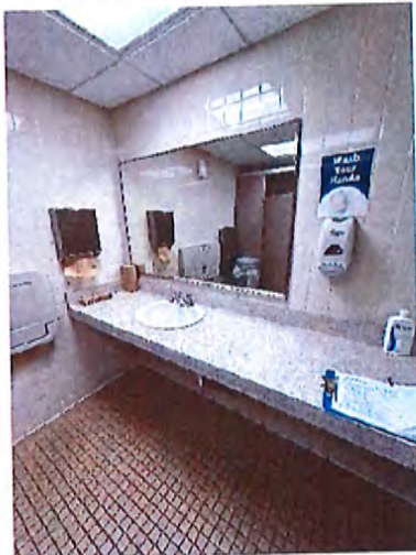
2 nd Floor Women's Toilet Room Sink
