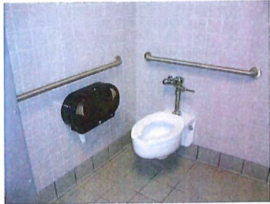
Men's Toilet Room Accessible Water Closet / Stall
