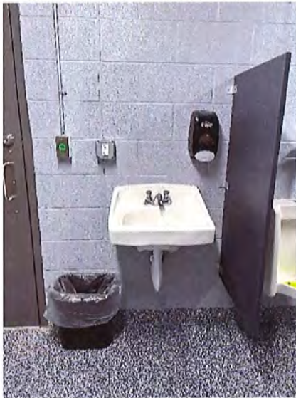
Men's Toilet Room Interior
