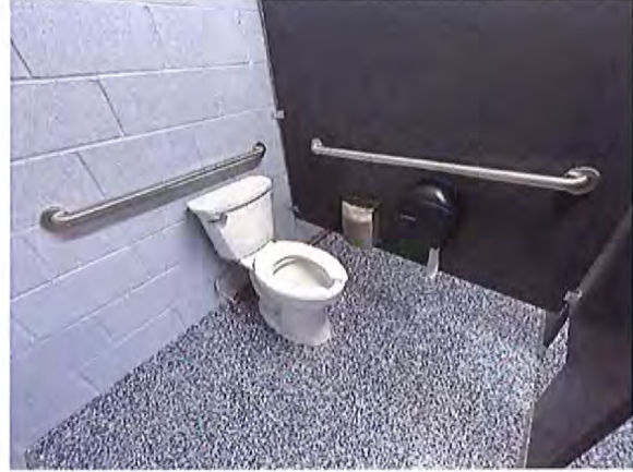
Upper Pavilion - Women's Toilet Room Accessible Water Closet / Stall
