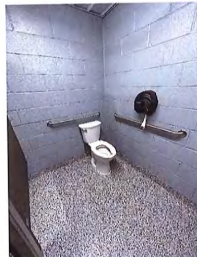
Men's Toilet Room Accessible
