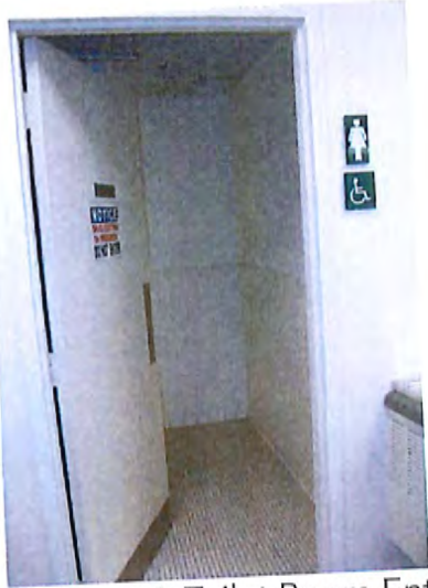
(Right) Women's Toilet Room Entrance
