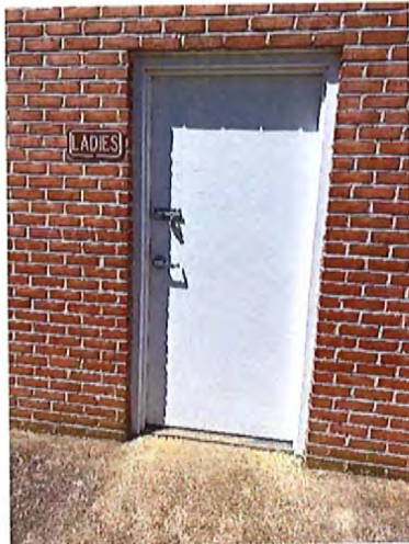
Women's Toilet Room Entrance
