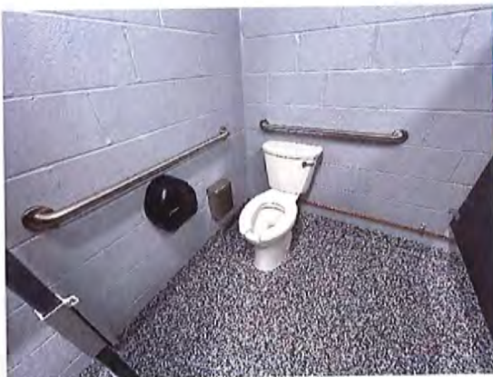
Arts Pavilion Women's Toilet Room Accessible Water Closet / Stall
