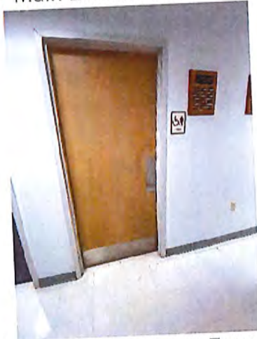
Women's Toilet Room Entrance
