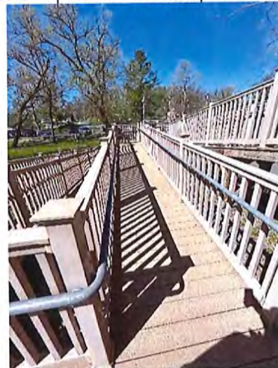
Middle Portion of Ramp to Bridge
