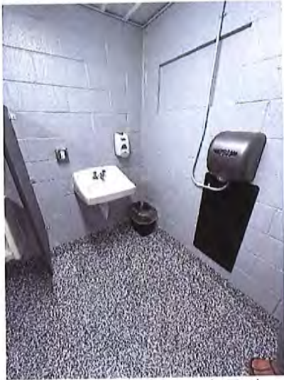
Southern Pavilion Left/North Toilet Room Sink
