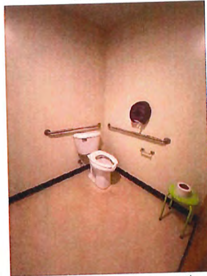
Kennel Club Building Men's Toilet Room Accessible Water Closet
