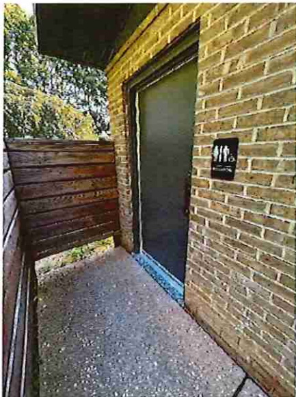
Tennis Court Left Toilet Room Entrance
