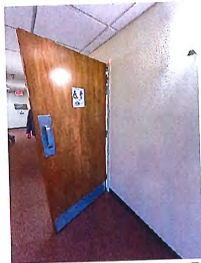
3rd Floor Women's Toilet Room Entrance
