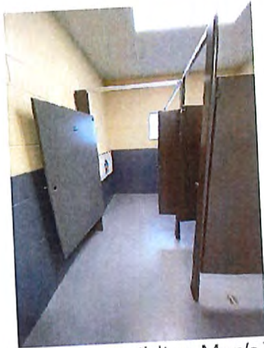
Multi-Purpose Building Men's Toilet Room Interior
