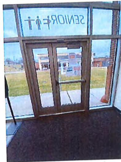
Main Entrance Interior
