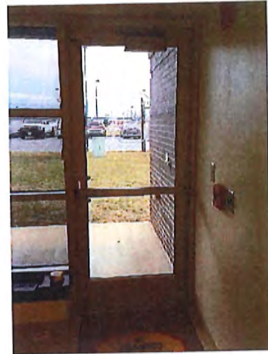
Main Entrance Interior
