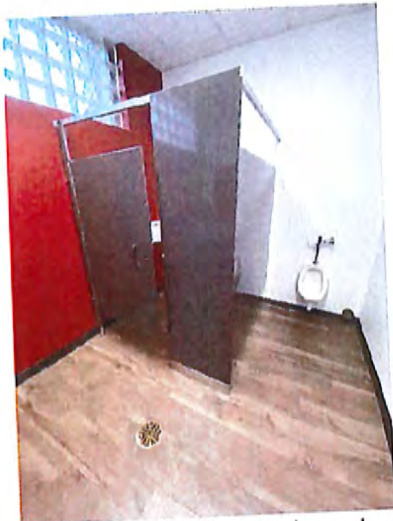
Men's Toilet Room Interior
