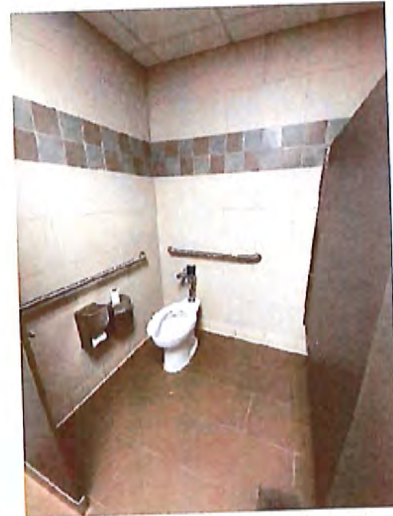
1st Floor Women's Toilet Room Accessible Stall
