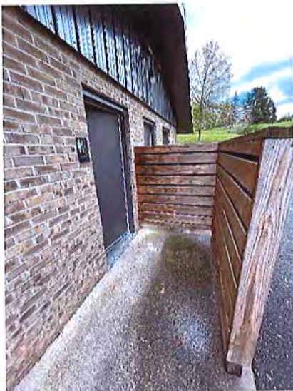
Women's Toilet Room Entrance
