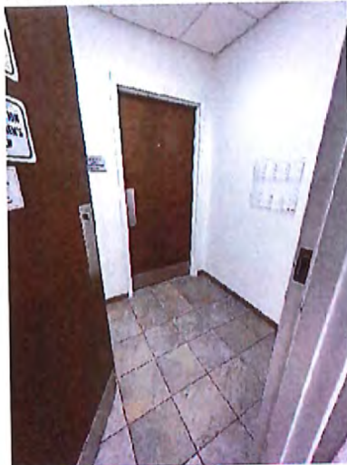
2 nd Floor Men's Toilet Room Entrance
