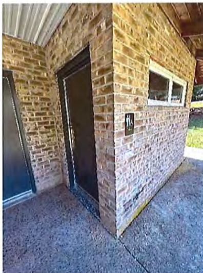
Lower Pavilion - Men's Toilet Room Entrance
