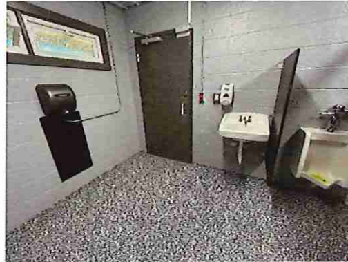
Pavilion #2 Men's Toilet Room Sink
