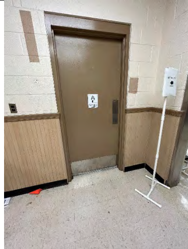
Rear Women's Toilet Room Entrance
