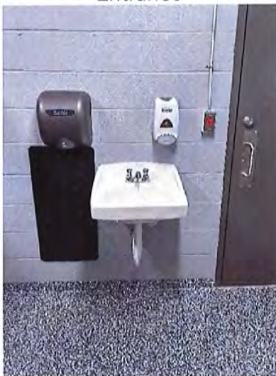
Lower Pavilion - Women's Toilet Room Sink
