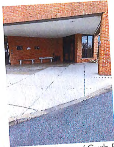
Main Entrance Route / Curb Ramp
