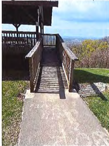
Ramp Entrance to Overlook Structure
