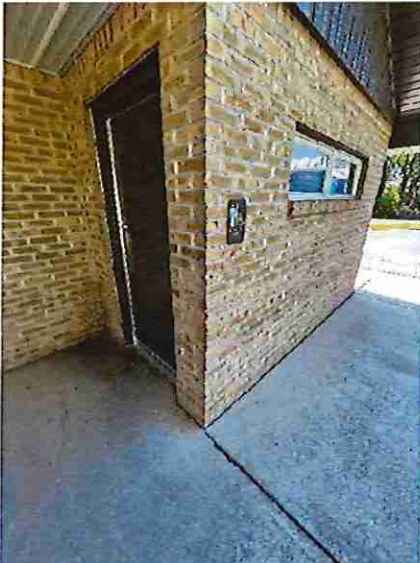
Pavilion #3 Men's Toilet Room Entrance
