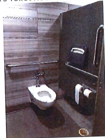
Men's Toilet Room Accessible Water Closet / Stall
