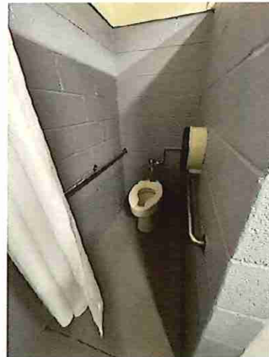
Pool Men's Toilet Room Accessible Water Closet / Stall
