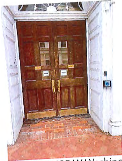
Main Entrance (35 W Washington)
