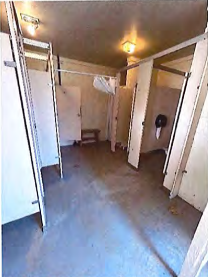
Women's Toilet Room Interior
