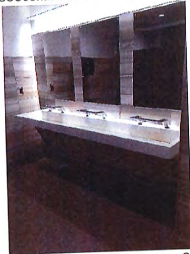
Terminal Men's Toilet Room Sinks
