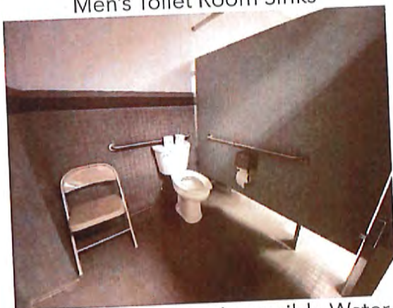
Men's Toilet Room Accessible Water Closet / Stall
