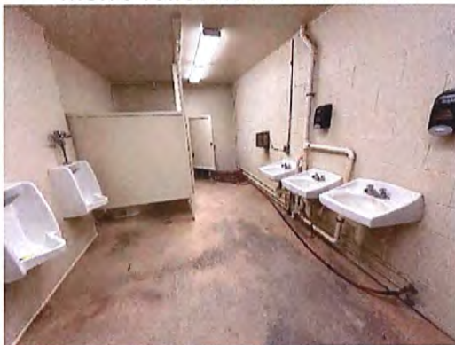
Men's Toilet Room Interior
