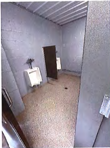
Pavilion Men's Toilet Room Interior
