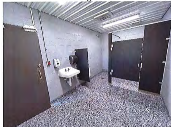
Lower Pavilion - Men's Toilet Room Interior
