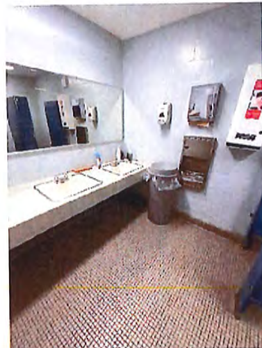
3rd Floor Women's Toilet Room Sinks
