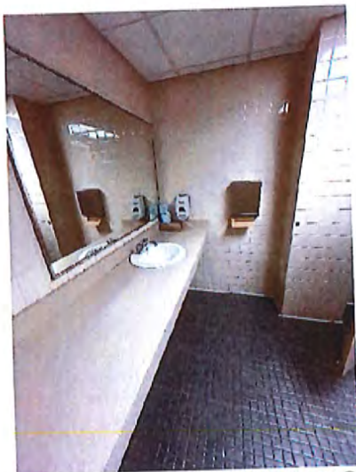
2 nd Floor Men's Toilet Room Sink
