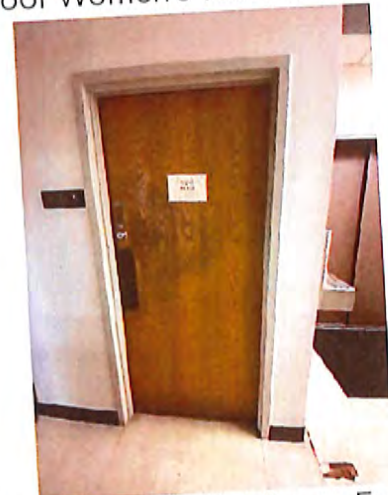
3rd Floor Men's Toilet Room Entrance
