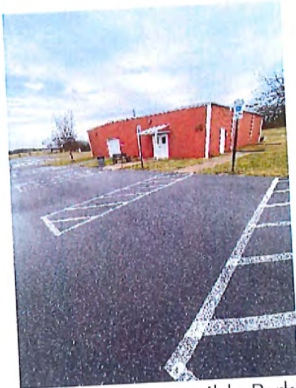
Rear Building Accessible Parking
