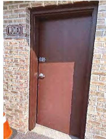
Women's Toilet Room Entrance
