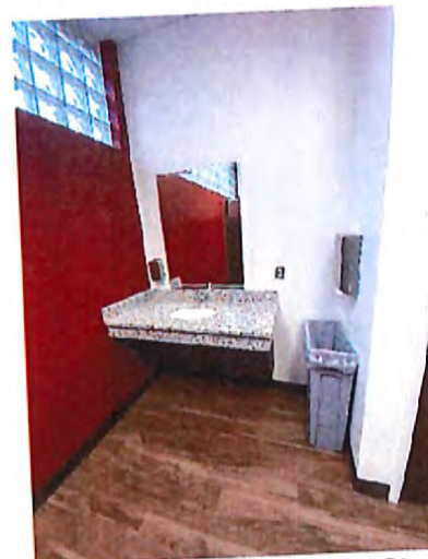
Women's Toilet Room Sink
