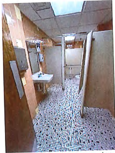
3rd Floor Men's Toilet Room Interior / Sink
