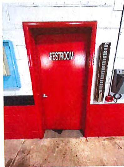
Toilet Room Entrance
