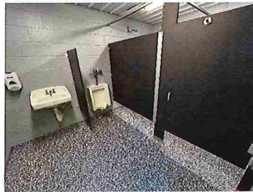
Tennis Court Left Toilet Room Interior
