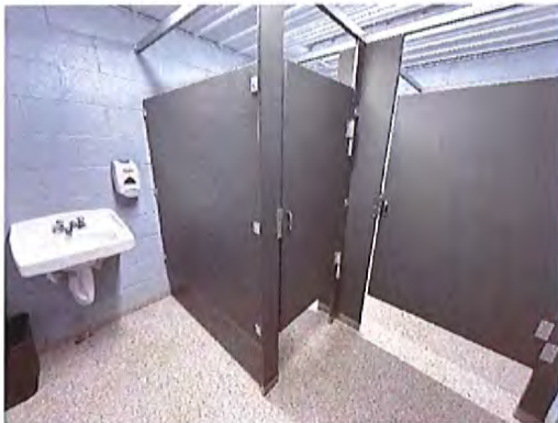
Women's Toilet Room Interior
