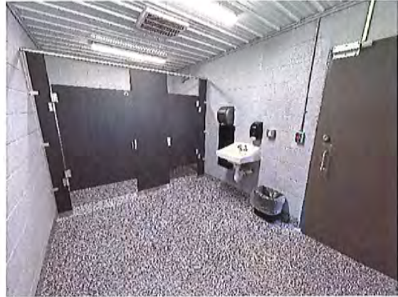
Women's Toilet Room Interior
