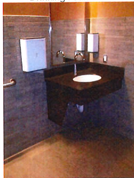
Single-Use Toilet Room Sink
