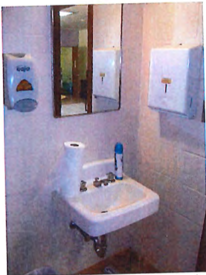
Women's Toilet Room Sink
