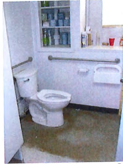
Toilet Room Accessible Water Closet / Stall
