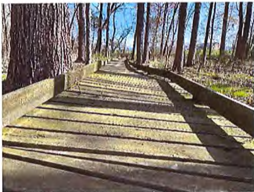
Elevated Walkway Surface
