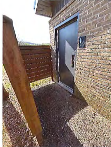
Women's Toilet Room Entrance
