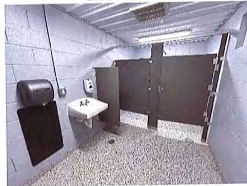
Men's Toilet Room Interior
