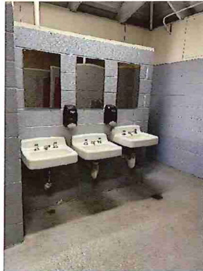
Pool Women's Toilet Room Sinks
