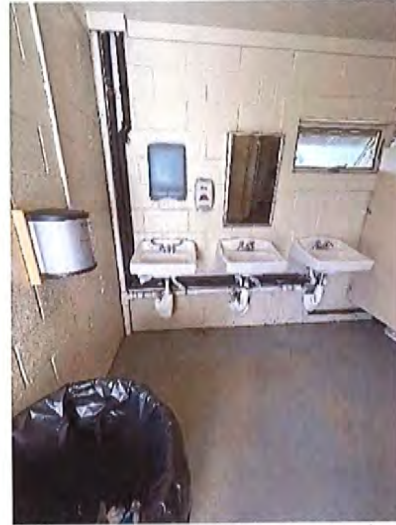
Women's Toilet Room Sinks
