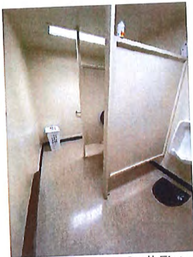
Men's Toilet Room Stall Fixtures
