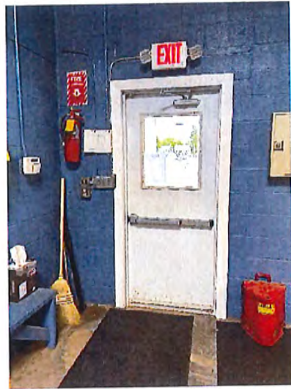
Main Entrance Interior
