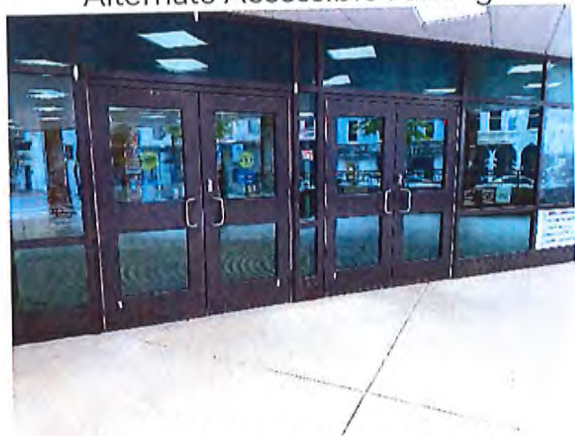
Main Entrance (From Street)
