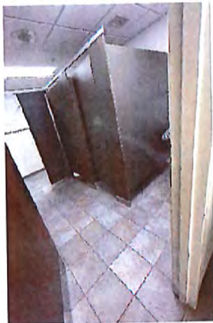
1st Floor Women's Toilet Room Interior
