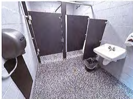
Northern Pavilion Left/East Toilet Room Interior
