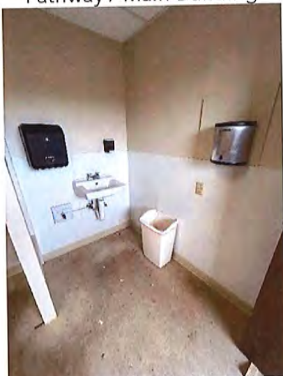
Men's Toilet Room Sink
