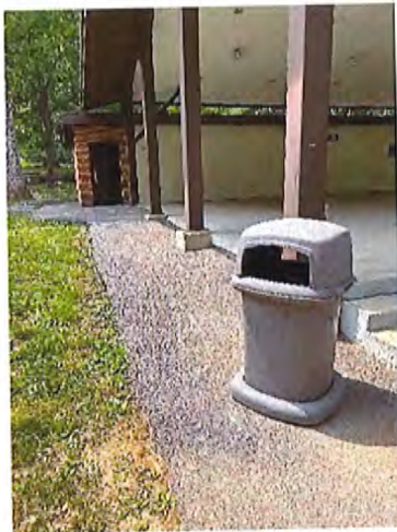
Arts Pavilion Ramp (South Side)
