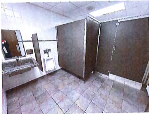
1st Floor Men's Toilet Room Interior
