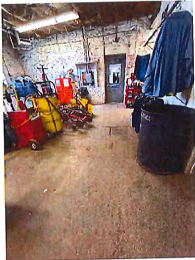
Interior Access Route
