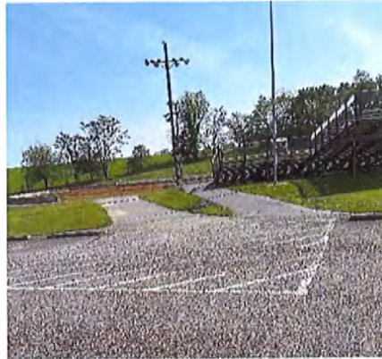
Access Aisle & Exterior Accessible Route
