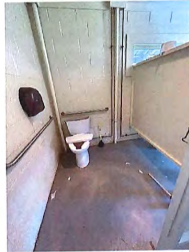
Men's Toilet Room Accessible Water Closet / Stall
