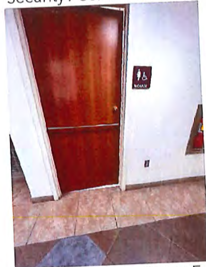
1st Floor Women's Toilet Room Entrance
