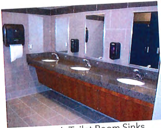
Women's Toilet Room Sinks
