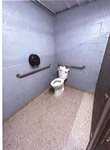
Men's Toilet Room Accessible Water Closet / Stall
