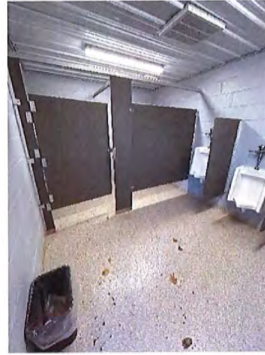
Men's Toilet Room Interior
