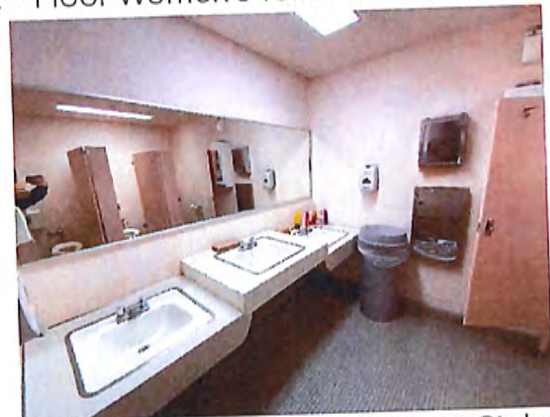
2nd Floor Women's Toilet Room Sinks
