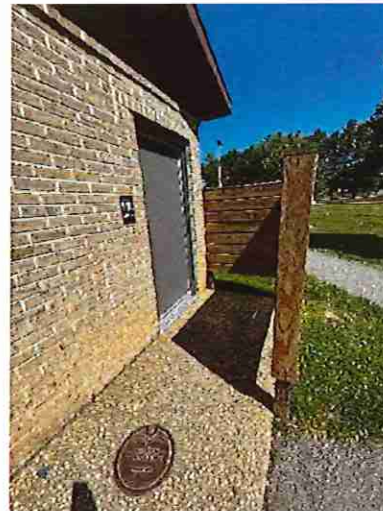
Little League Right Toilet Room Entrance
