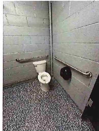
Pavilion #4 Men's Toilet Room Accessible Water Closet / Stall
