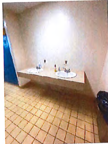
Men's Toilet / Locker Room Sinks
