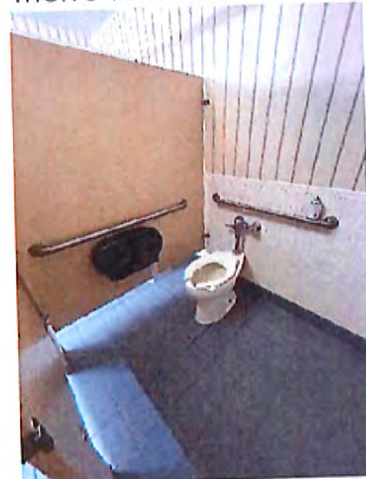
Men's Toilet Room Accessible Stall
