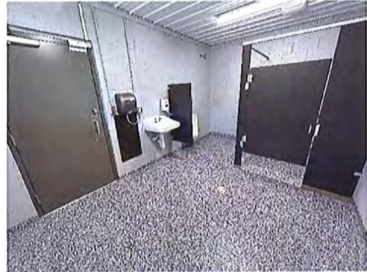
Upper Pavilion - Men's Toilet Room Interior
