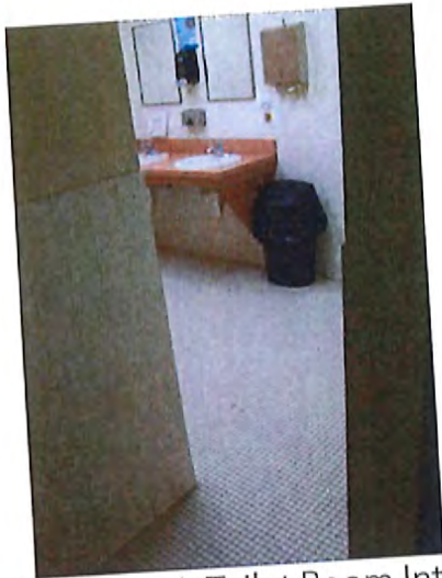
(Left) Women's Toilet Room Interior Access Route
