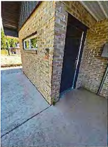
Pavilion #3 Women's Toilet Room Entrance
