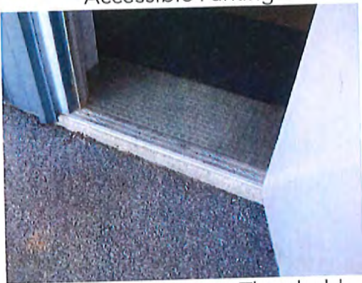
Main Entrance Door Threshold
