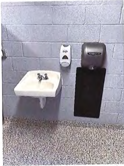
Women's Toilet Room Sink
