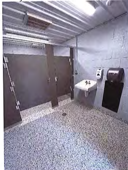
Women's Toilet Room Interior
