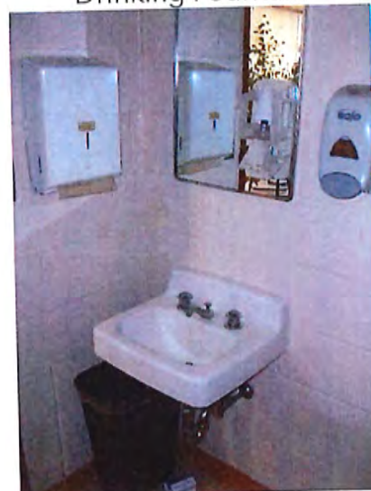
Men's Toilet Room Sink
