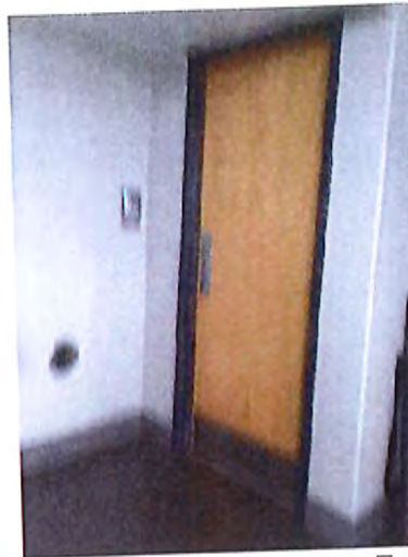
Terminal Men's Toilet Room Entrance
