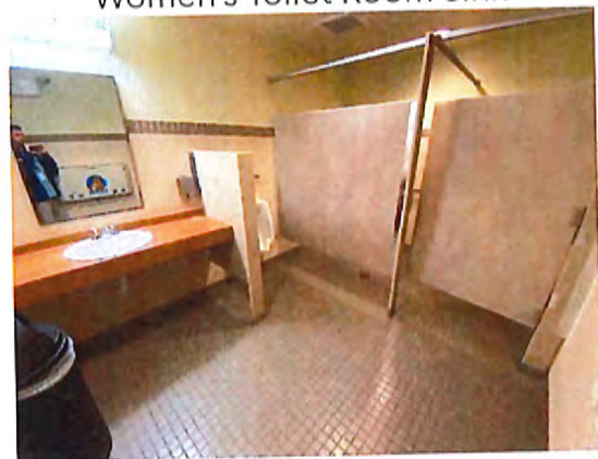
Men's Toilet Room Interior
