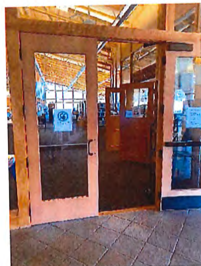
Interior Access Route
