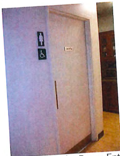
(Left) Women's Toilet Room Entrance
