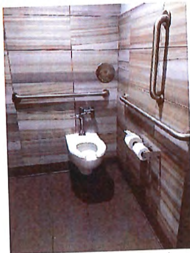
Terminal Men's Toilet Room Accessible Water Closet / Stall
