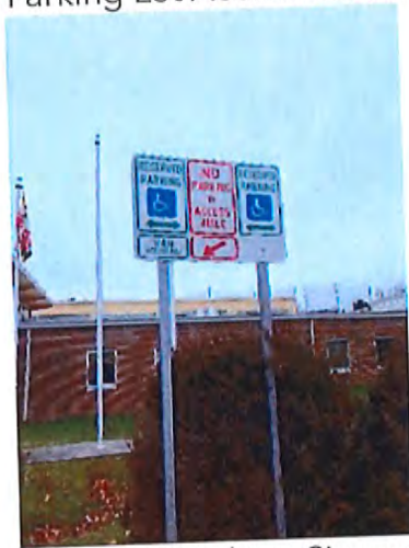
Accessible Parking Signage
