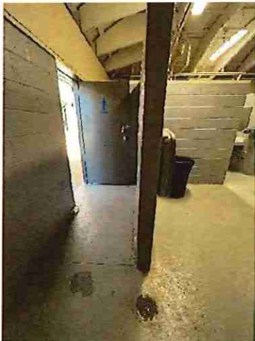
Pool Men's Toilet Room Entrance Interior
