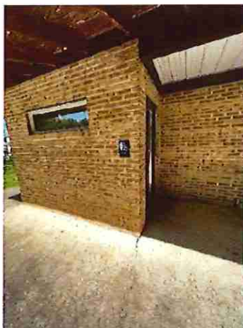
Pavilion #4 Women's Toilet Room Entrance
