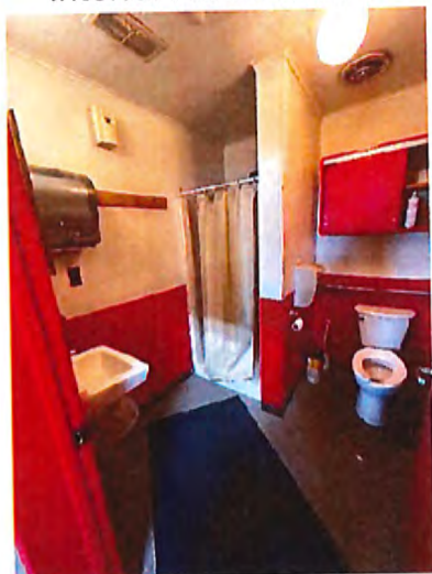
Toilet Room Interior
