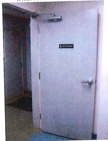
Toilet Room Entrance
