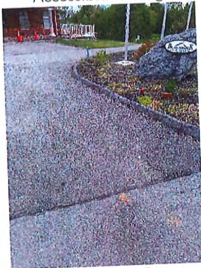
Exterior Access Route
