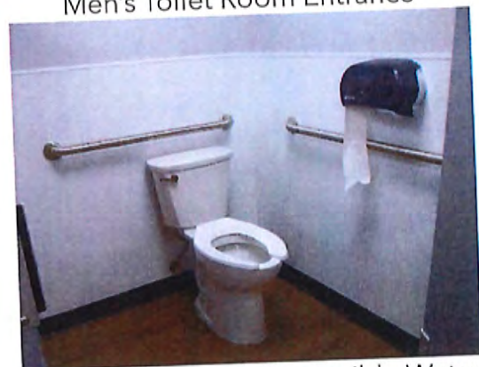
Men's Toilet Room Accessible Water Closet / Stall
