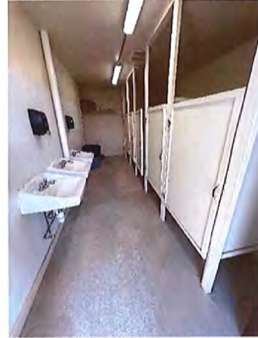
Women's Toilet Room Interior
