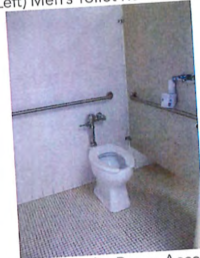
(Left) Men's Toilet Room Accessible Water Closet / Stall
