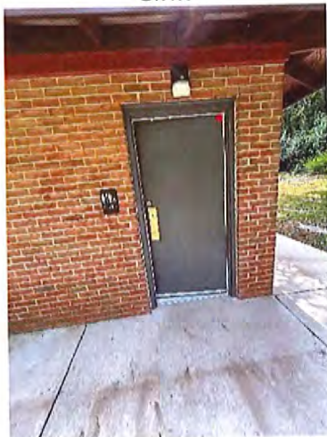
Southern Pavilion Left/North Toilet Room Entrance
