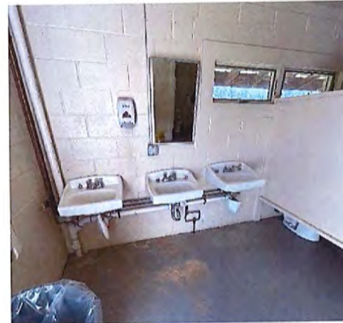
Women's Toilet Room Sinks
