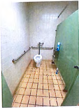
Women's Toilet / Locker Room Accessible Water Closet / Stall
