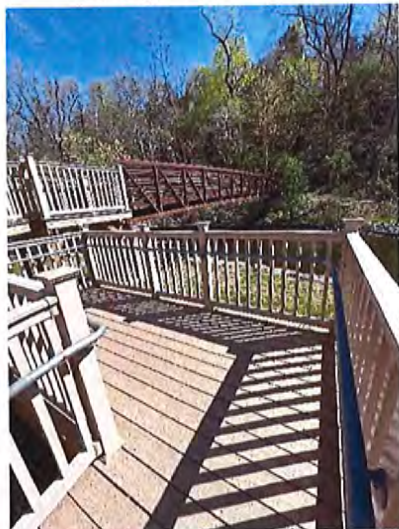
Bridge Ramp Landing Area / Turning Space
