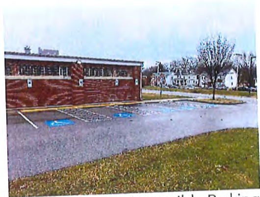
Rear Parking Lot Accessible Parking
