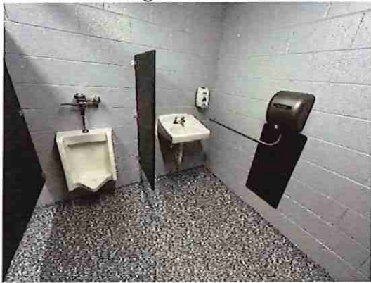
Tennis Court Right Toilet Room Sink
