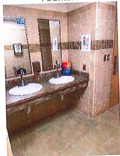
Men's Toilet Room Sinks
