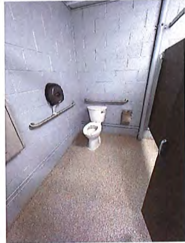
Pavilion Women's Toilet Room Accessible Water Closet / Stall
