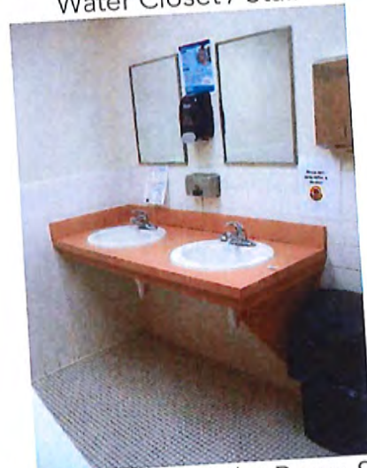
(Left) Women's Toilet Room Sink
