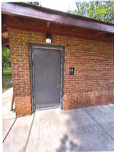
Southern Pavilion Right/South Toilet Room
