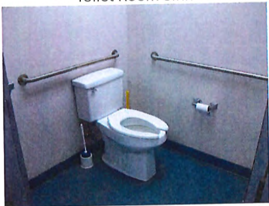
Toilet Room Accessible Water Closet / Stall
