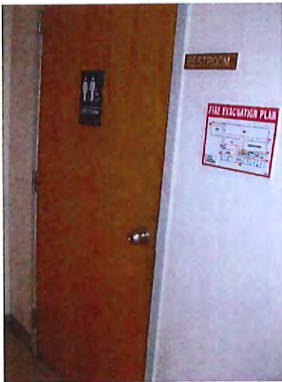
Toilet Room Entrance
