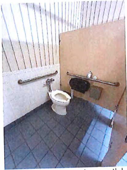
Women's Toilet Room Accessible Stall
