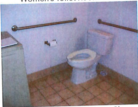
Women's Toilet Room Water Closet
