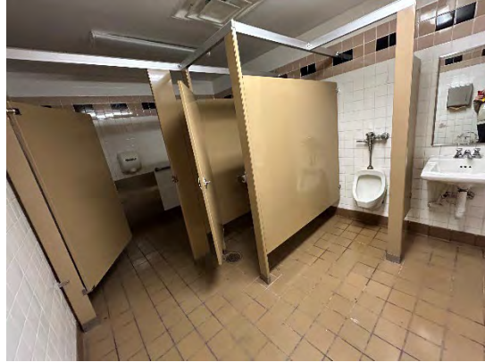
Rear Men's Toilet Room Interior
