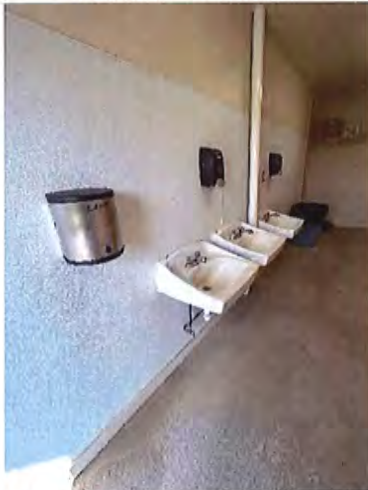
Women's Toilet Room Sinks
