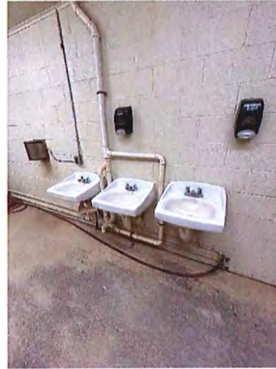
Men's Toilet Room Sinks
