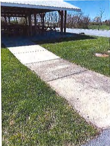
Exterior Accessible Route to Toilet Rooms
