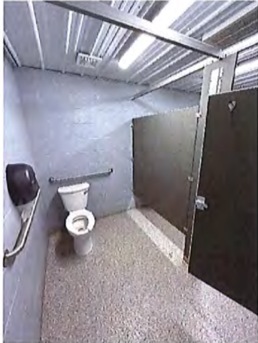
Men's Toilet Room Accessible Water Closet / Stall
