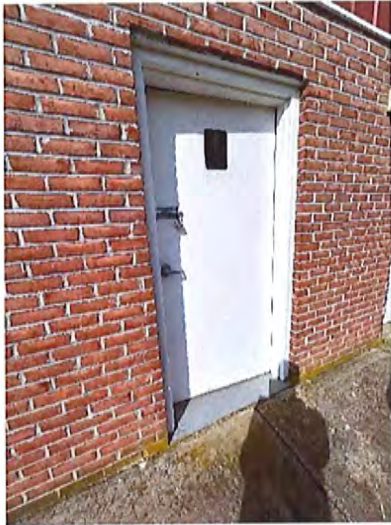
Women's Toilet Room Entrance
