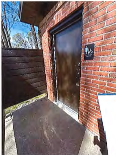
Women's Toilet Room Entrance
