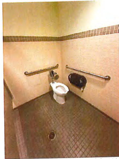
Men's Toilet Room Accessible Water Closet / Stall
