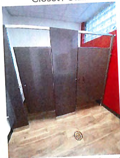
Women's Toilet Room Interior
