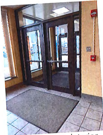
Main Entrance Interior
