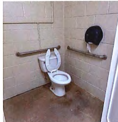
Men's Toilet Room Accessible Water Closet
