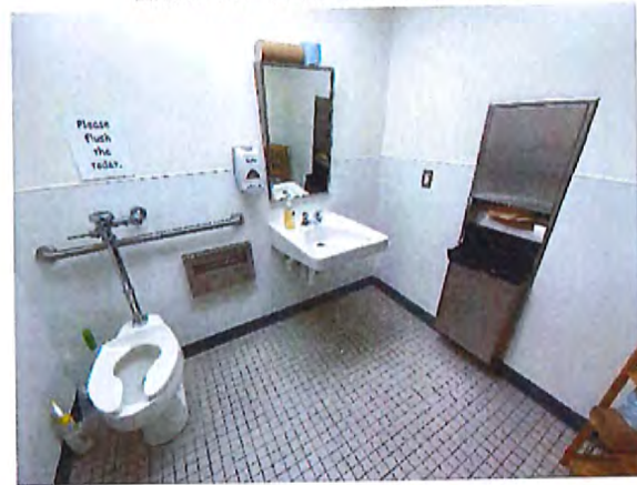
Men's Toilet Room
