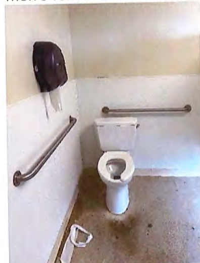
Men's Toilet Room Accessible Water Closet / Stall
