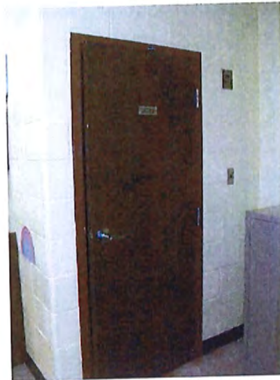
Women's Toilet Room Entrance
