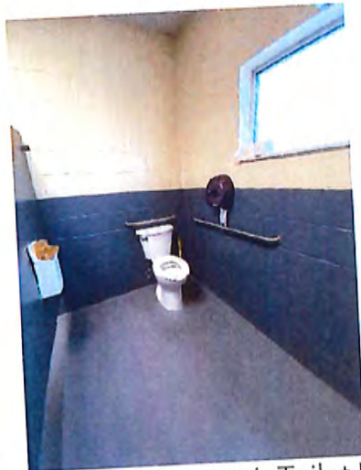
Multi-Purpose Women's Toilet Room Accessible Water Closet / Stall
