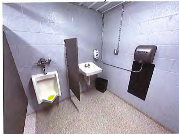
Men's Toilet Room Interior
