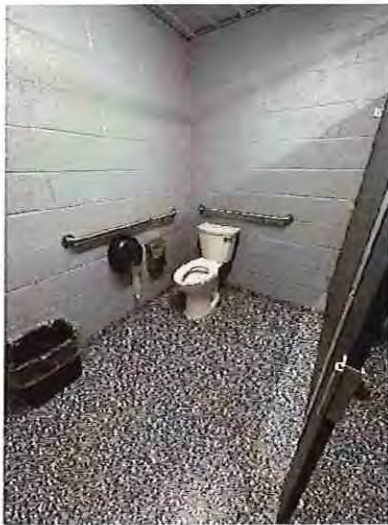
Little League Right Toilet Room Accessible Water Closet / Stall
