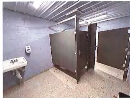
Women's Toilet Room Interior
