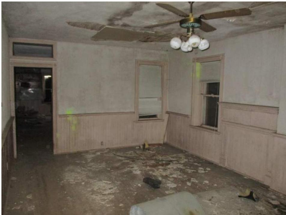
Photo #2: View of the water damage on the ceiling in the Living Room of the Farmhouse.
