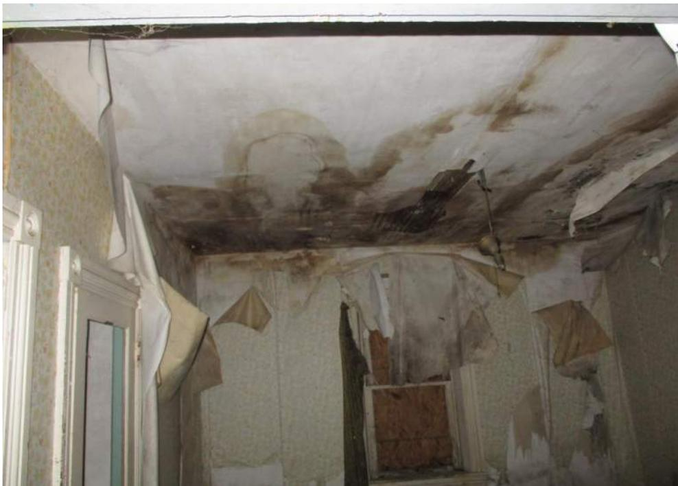
Photo #8: View of mold and water damaged observed in a room located on the 2<sup>nd</sup> floor of the Farmhouse.
