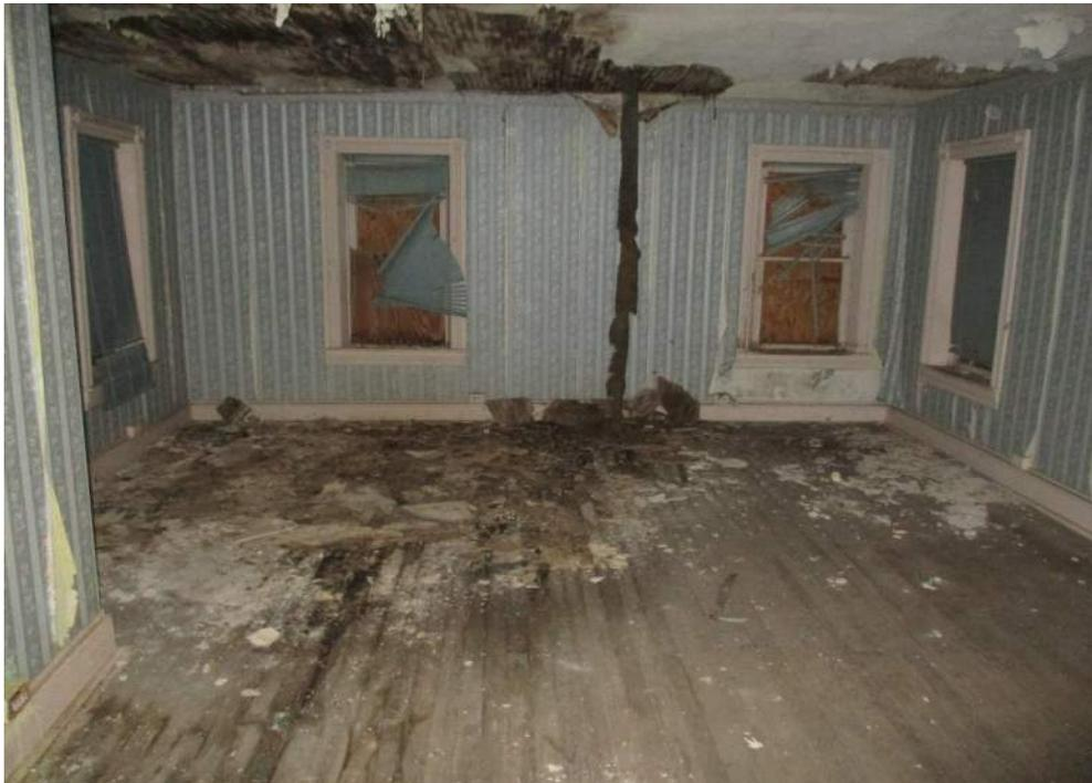
Photo #9: View of mold observed in one of the rooms located on the 2<sup>nd</sup> floor of the Farmhouse.
