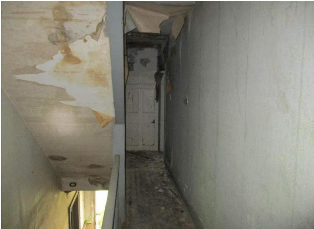
Photo #6: View of mold and water damage observed on the under carriage of the 2<sup>nd</sup> floor stairs.
