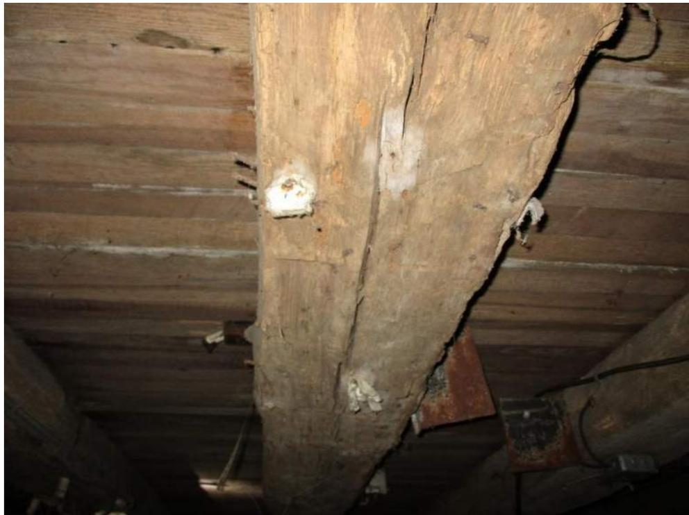
Photo #2: Samples 2A-2C – White insulation collected from a wooden beam located in the basement of the Farmhouse.
