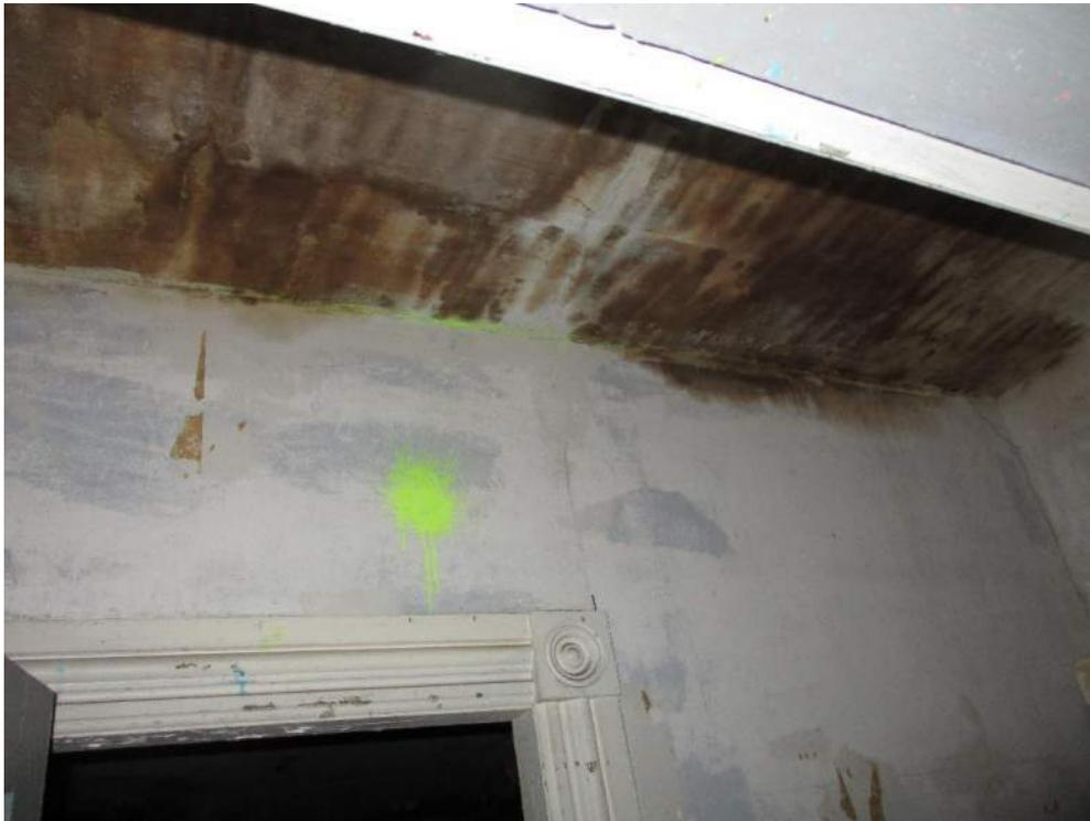
Photo #13: View of mold observed on the 2<sup>nd</sup> floor.
