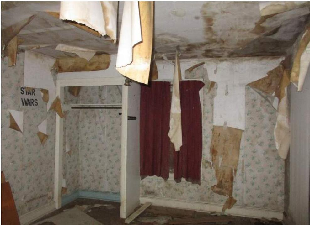
Photo #10: View of water damaged observed in a room located on the 2<sup>nd</sup> floor of the Farmhouse.
