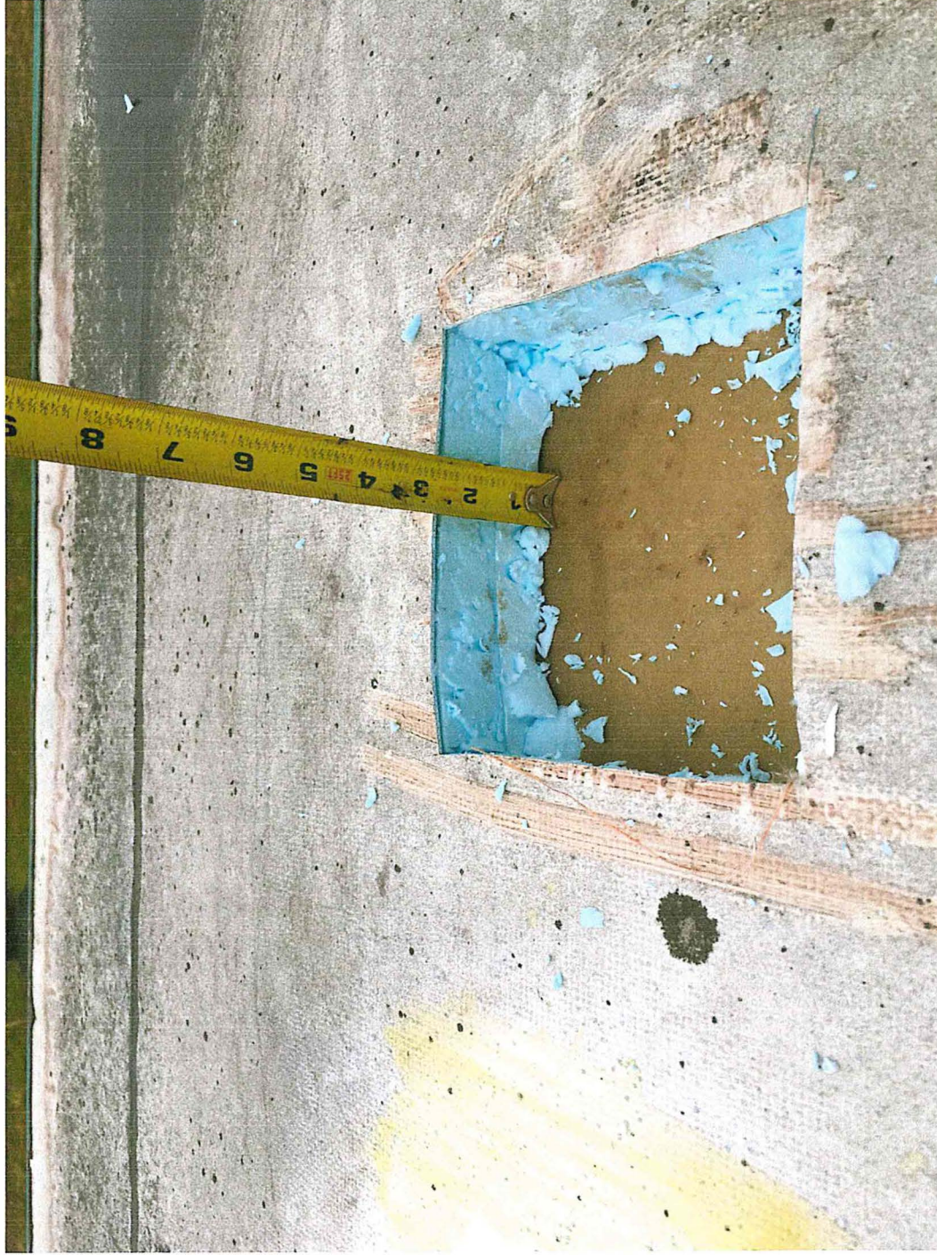
BUILDING #3 SOLID HANDLING UPPER ROOF LOW POINT
