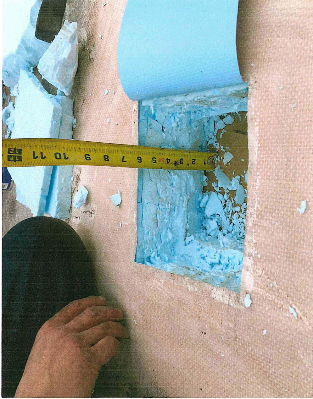
BUILDING #3 SOLID HANDLING UPPER ROOF HIGH POINT
