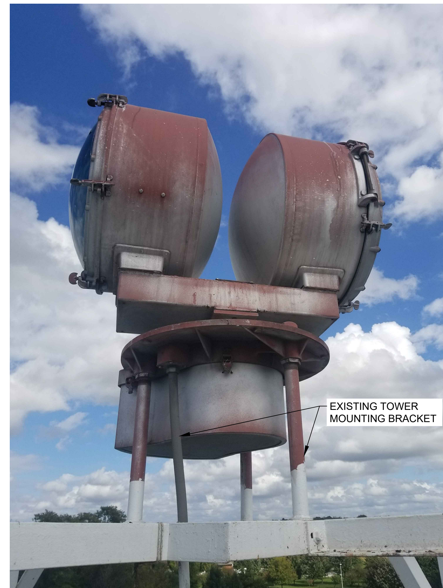
EXISTING ROTATING BEACON - IMAGE 2
