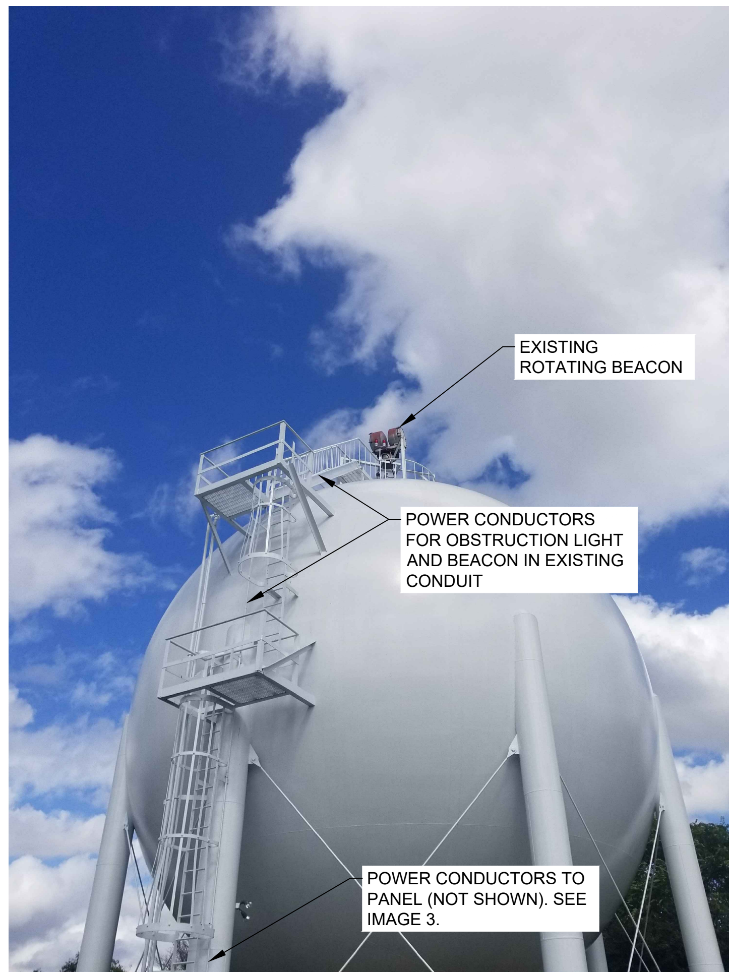
EXISTING ROTATING BEACON - IMAGE 1
