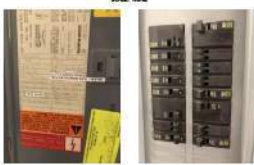
EX. TECH PANELBOARD SCALE NONE
