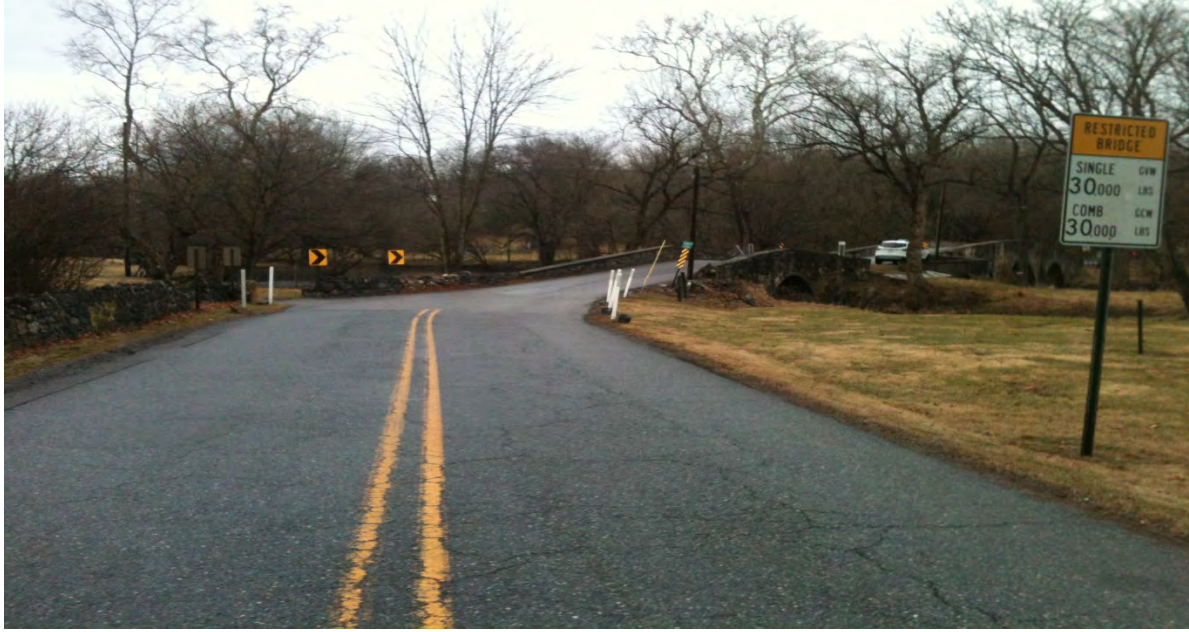
Poffenberger Rd Bridge W4011 & W4012 (Looking East)
