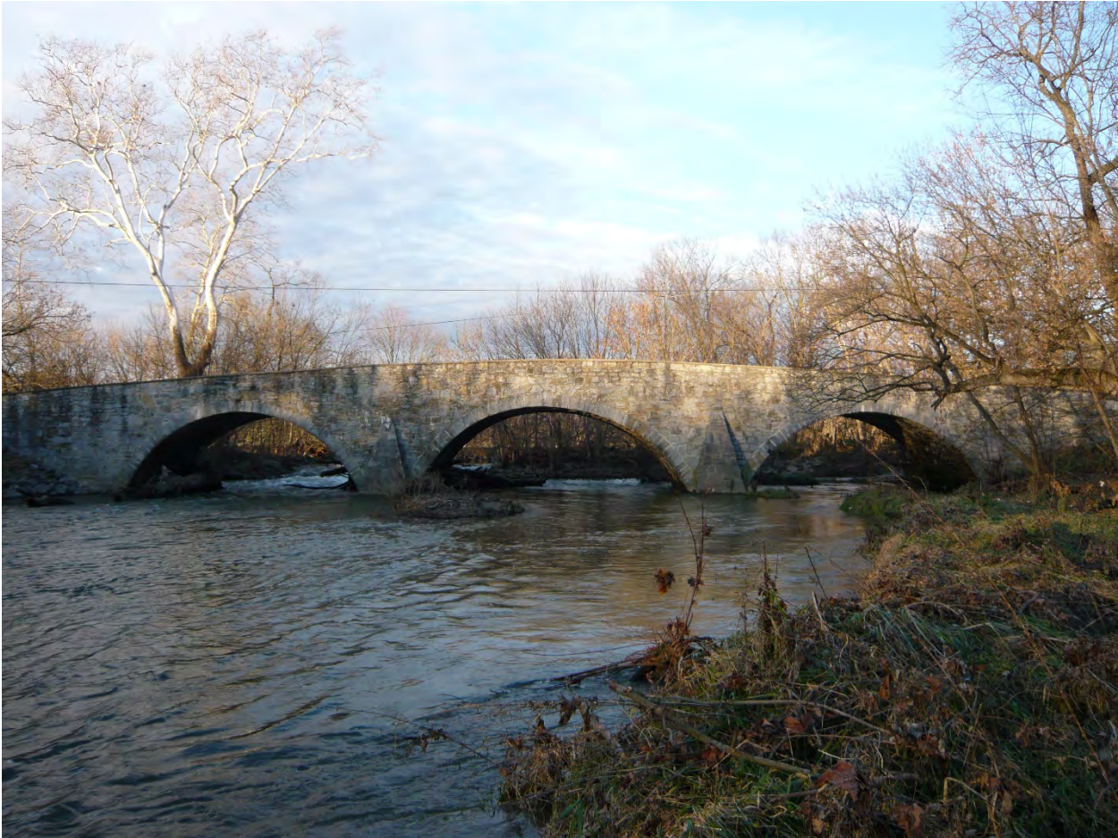
Poffenberger Road Bridge W4012
