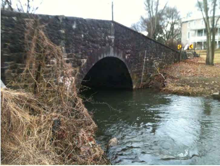
Poffenberger Road Bridge W4011
