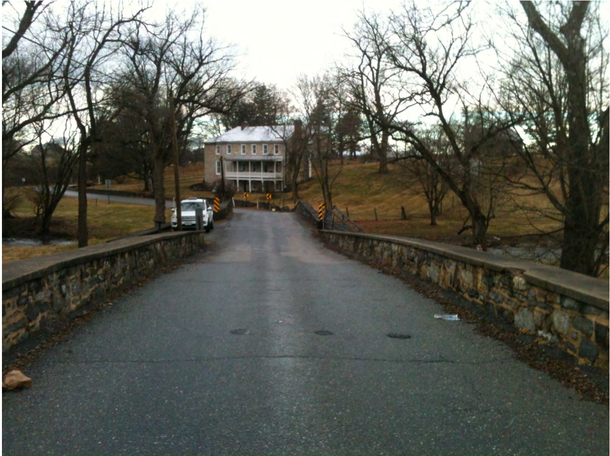
Poffenberger Rd Bridge W4011 & W4012 (Looking West)
