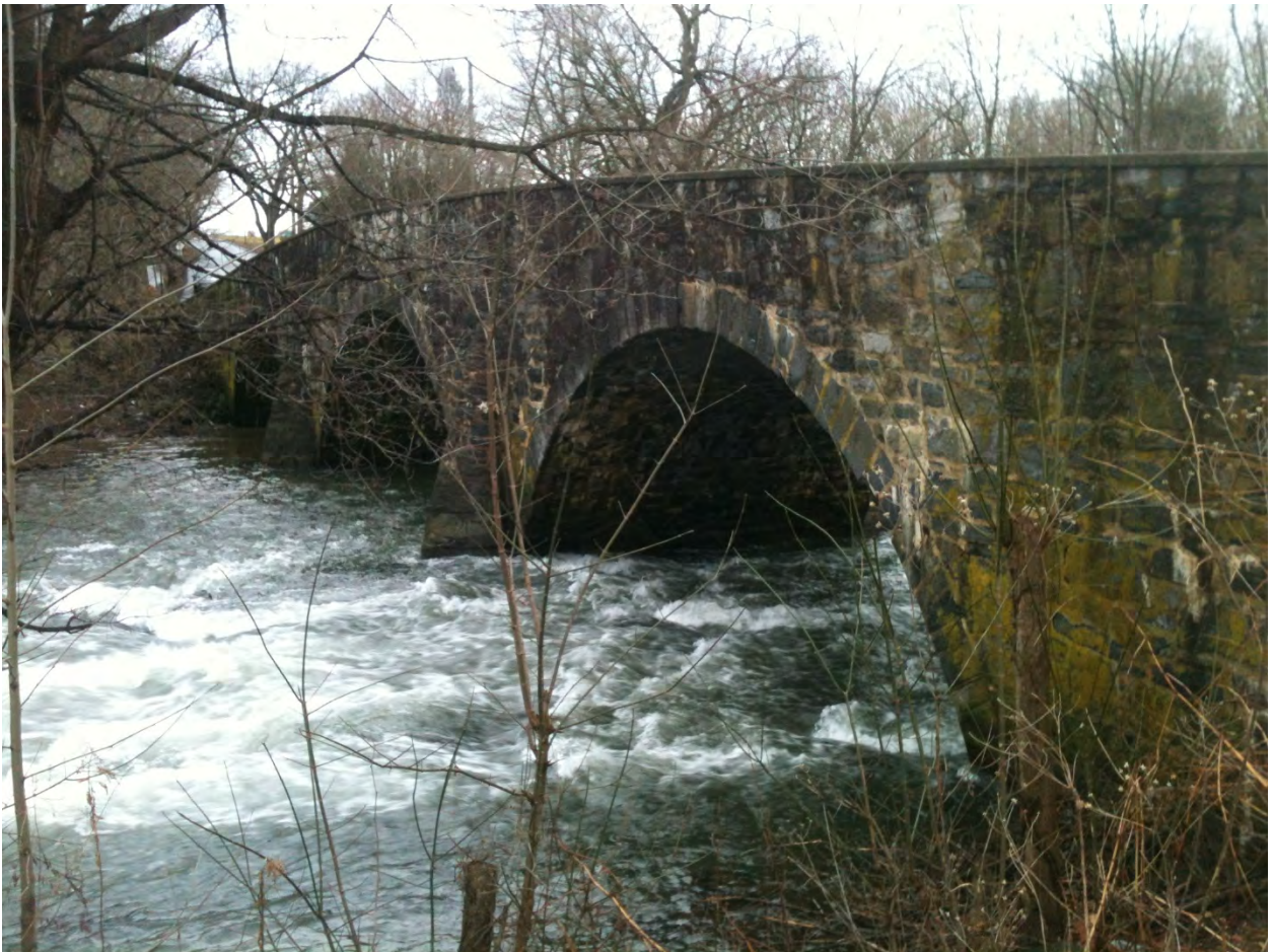
Poffenberger Road Bridge W4012
