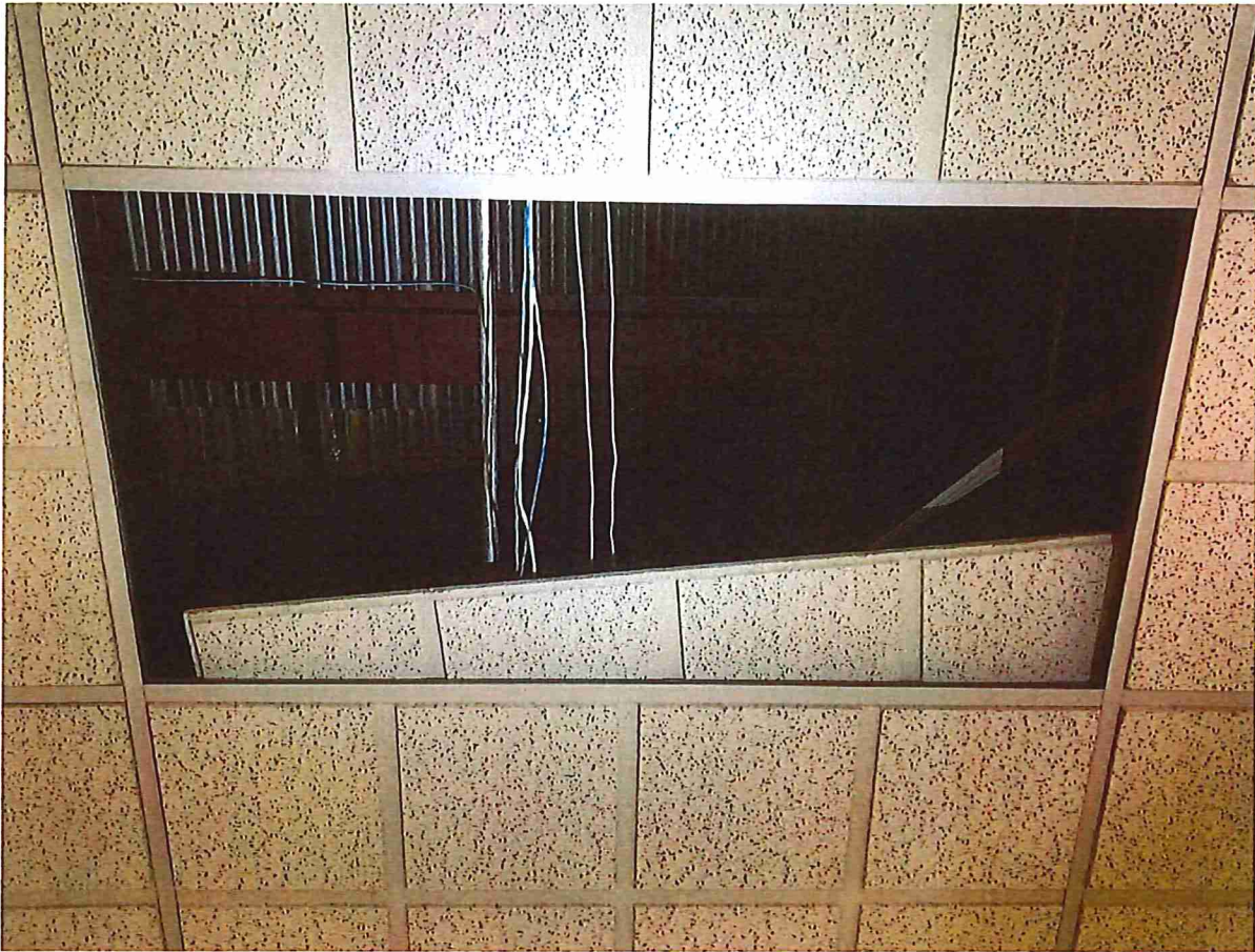
Photo of Ceiling Area Directly Above Proposed Door
